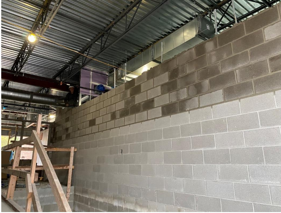
The east masonry stair wall at the second-floor level of Area D is nearly complete.
