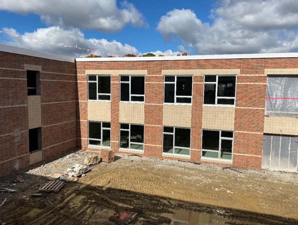
Installation of Area D windows should be complete this week. Installation of storefront doors and glazing is yet to be completed.
