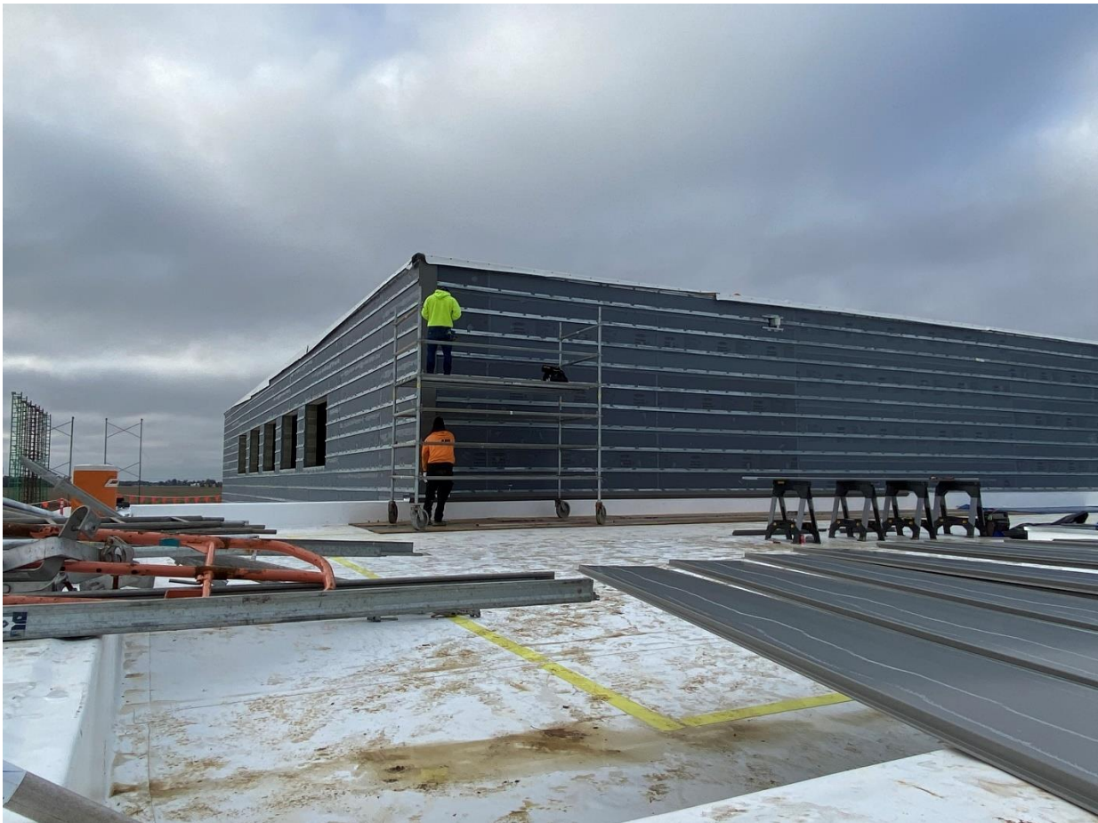
Installation of metal siding at the upper Gym area.
