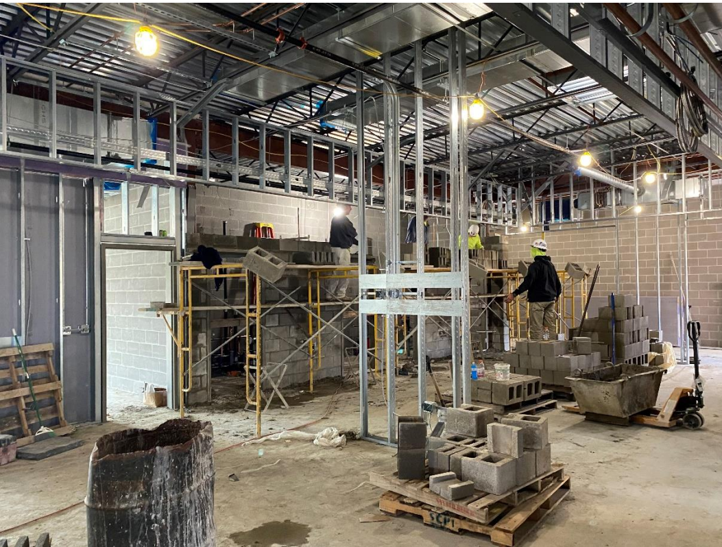
Construction of interior toilet room walls is progressing at Area D.
