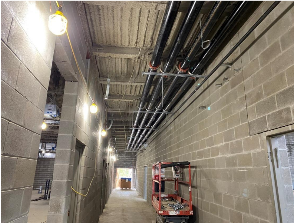
Installation of main line hydronic piping is progressing in the corridor adjacent to the Locker Rooms.
