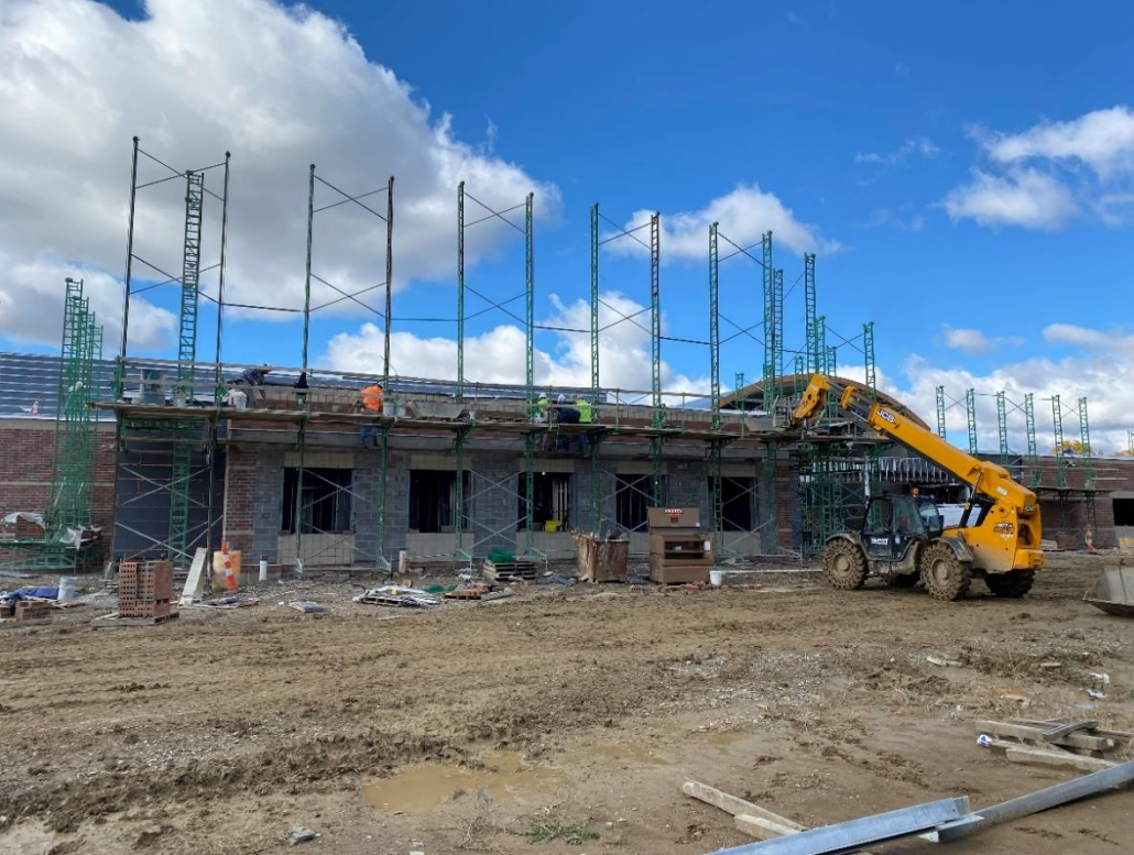
Brick veneer is "topped out" at the east elevation of Area A. Installation of brick piers between the windows and installation of a cornice is yet to be completed.
