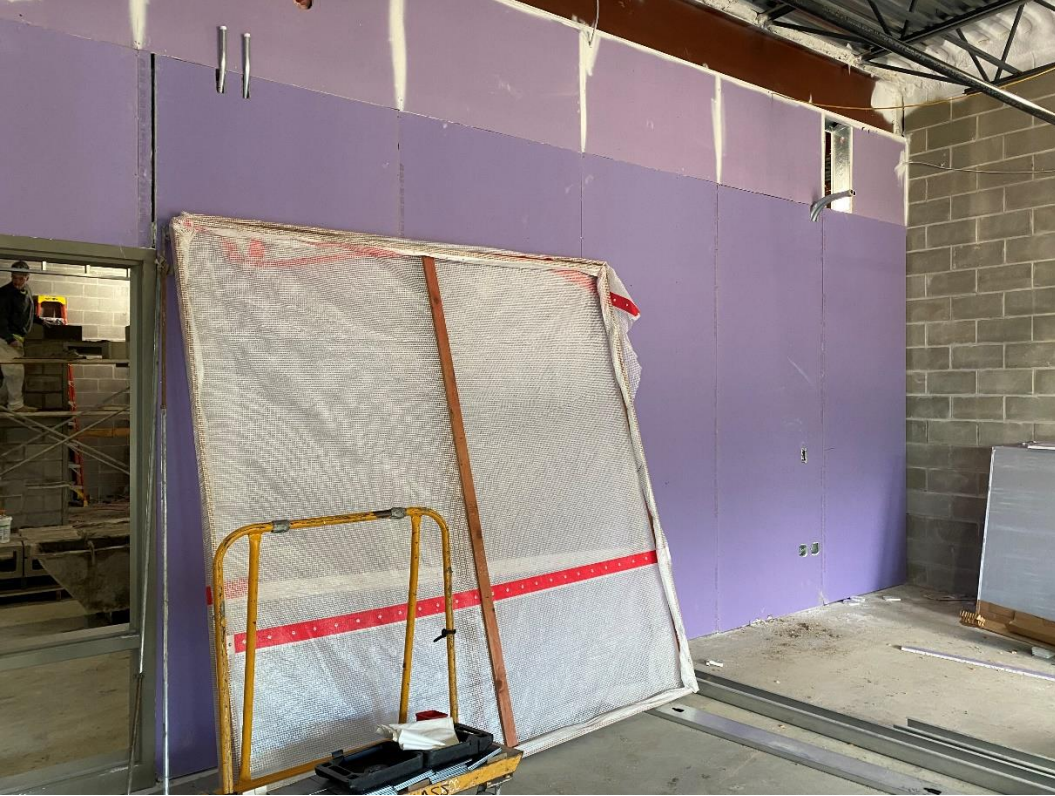
Installation of impact resistant drywall has started at the second-floor of Area D.
