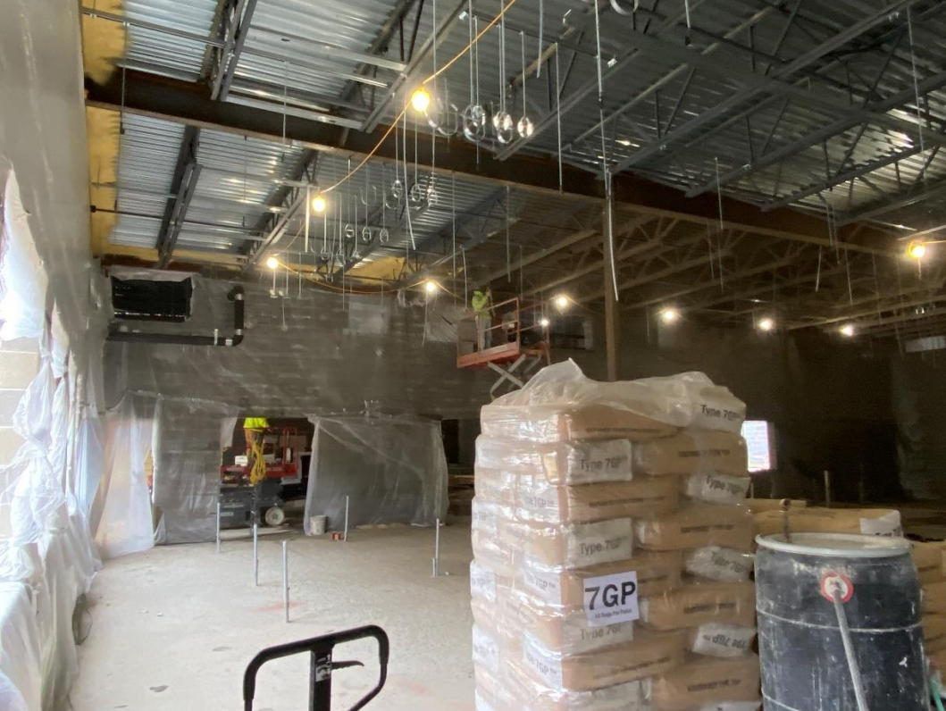
Spray-on fire-proofing continues in the Kitchen.
