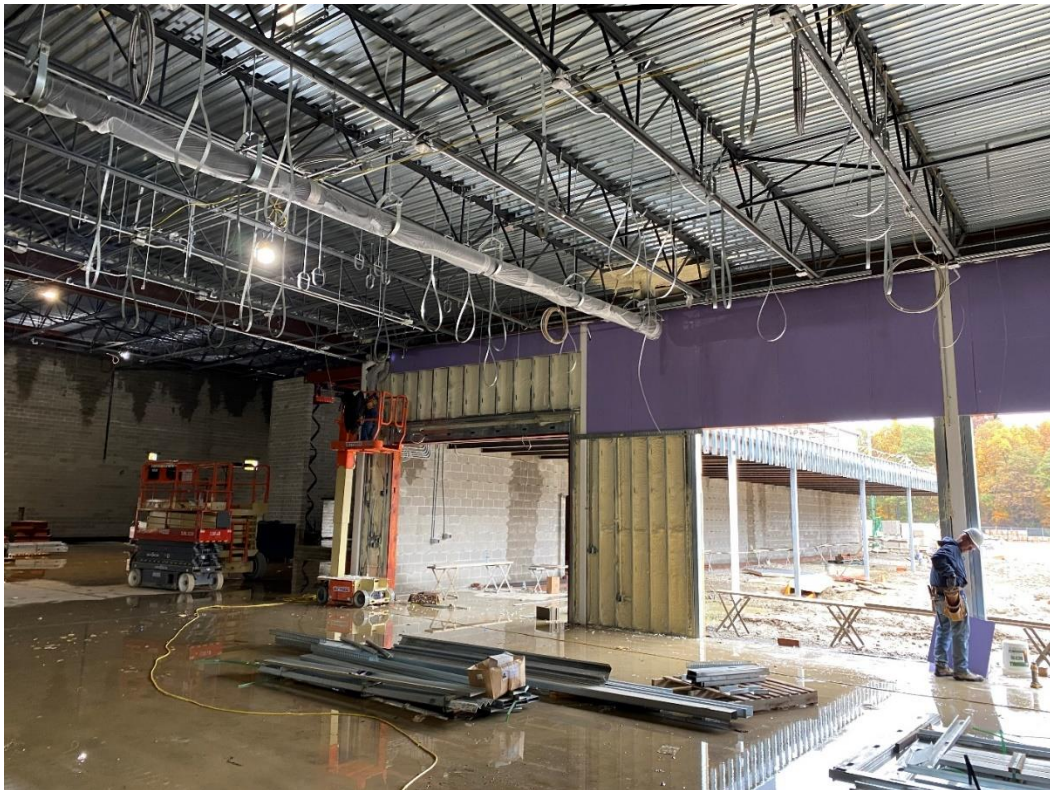
Above ceiling moisture resistant drywall is installed on the north wall of the Student Dining area.
