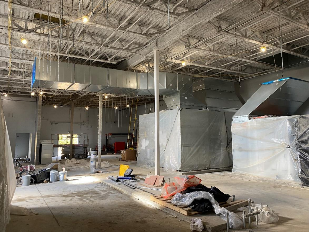
Installation of large ductwork has started in the main mechanical room. Work will progress into the Gym this week.
