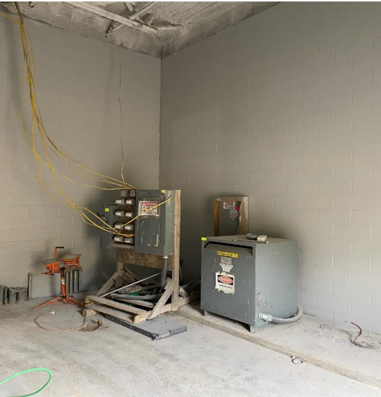
Prime painting of walls continues in mechanical rooms.
