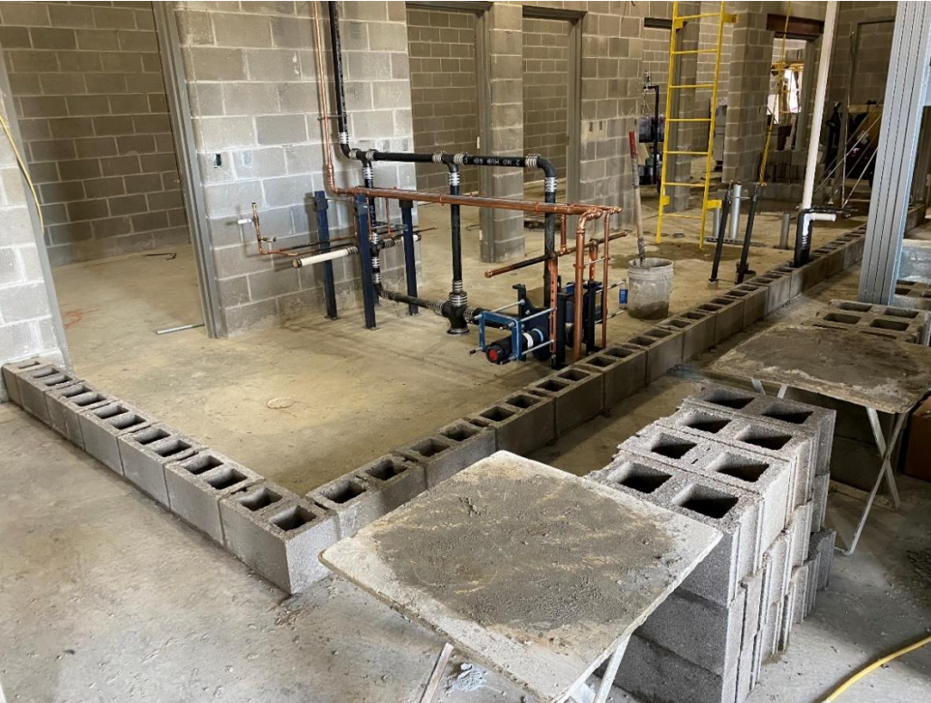
Interior masonry at the second-floor toilets at Area C is progressing.
