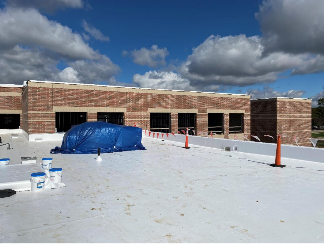
Roofing work is complete at Area B & C.
