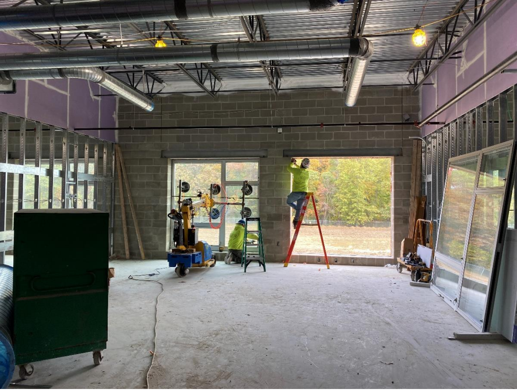
Installation of windows continues at the second-floor level of Area D. View looking north.
