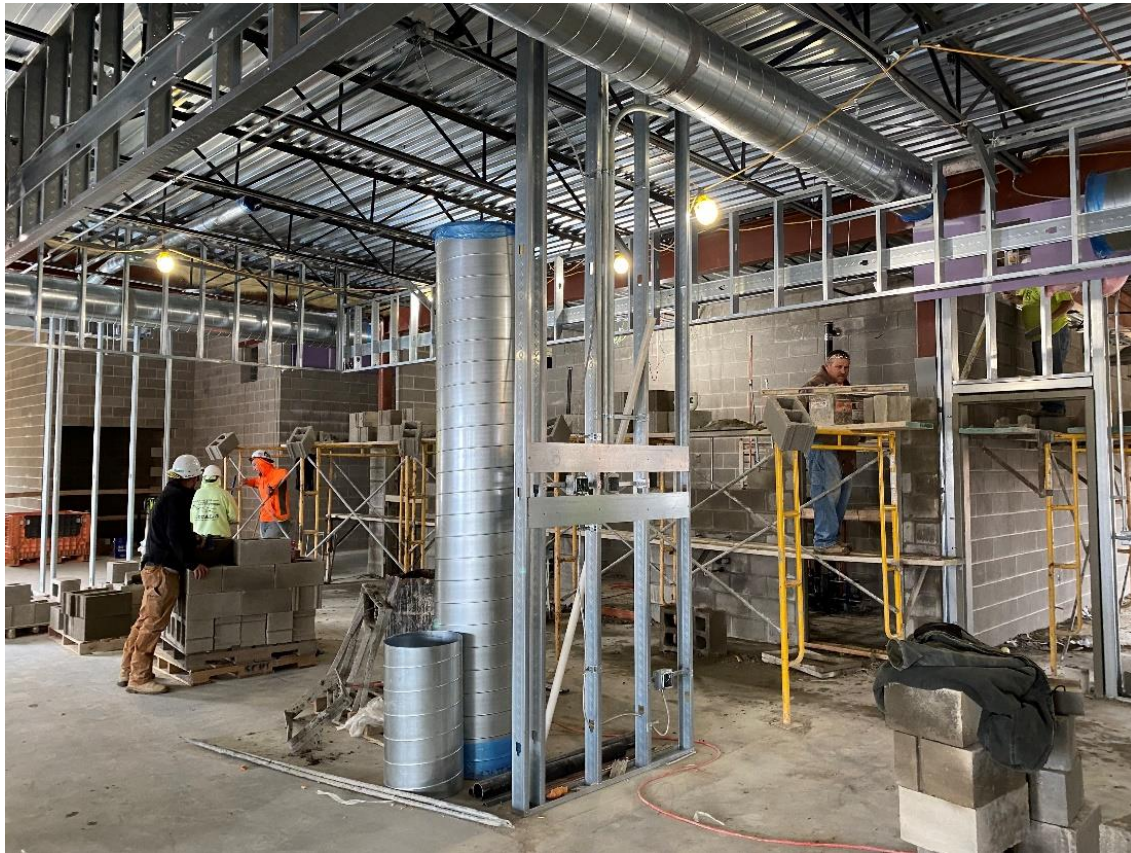
Masonry walls progressing at the individual toilet rooms on the Second-floor of Area C.
