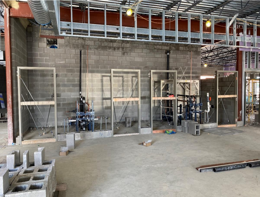
Interior toilet room walls are progressing at Area C.
