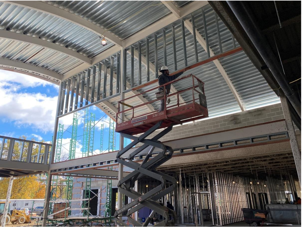
Installation of wood blocking for the aluminum storefront system is installed in the main entry.
