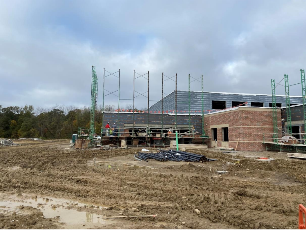
Brick veneer work is progressing at the east end of Area E, Locker Rooms.
