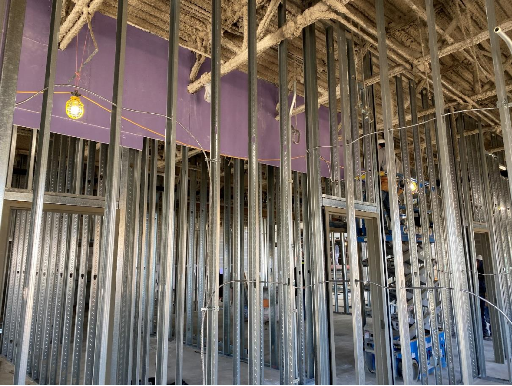
Installation of above ceiling drywall has started in the Administrative Offices.
