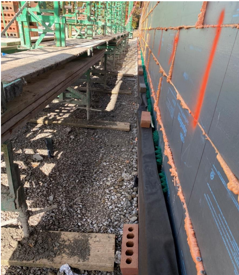
Installation of base flashing and mortar net is complete at the west side of Area C.
