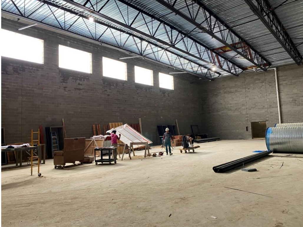
"Carpentry Shop" in the Gym. Temporary doors are being made in preparation for temporary heat in Areas C & D.
