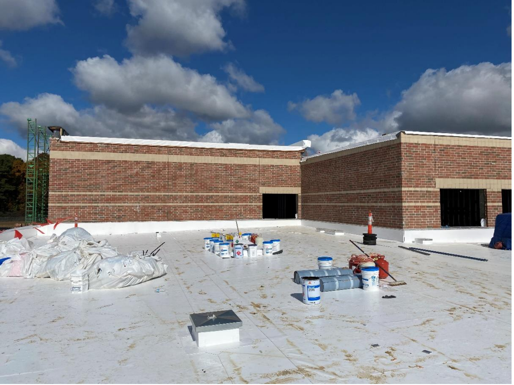
Area B & C roofing; view looking north toward the two story section of Area C.
