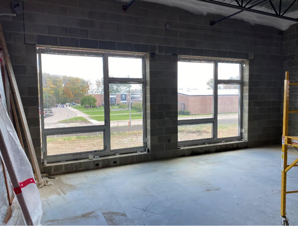
Installation of windows is progressing at the second-floor level of Area D.
