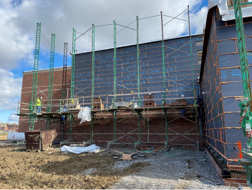
Brick veneer is progressing on the west side of Area D.
