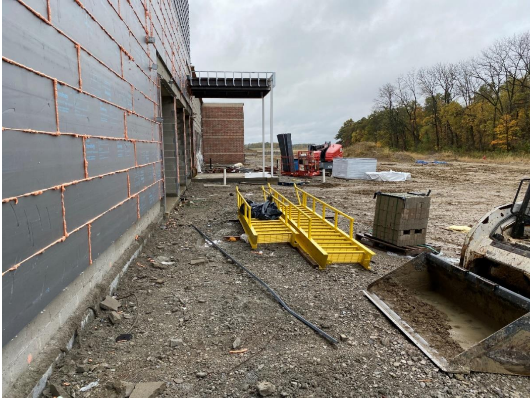
Ships ladders have arrived. These will be used for access to the control booth in the performing arts center.
