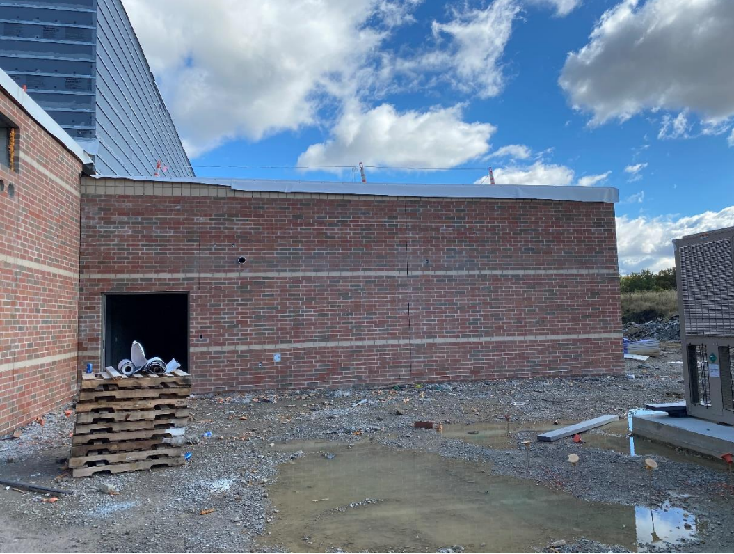
Brick veneer is complete on the west side of Area E.
