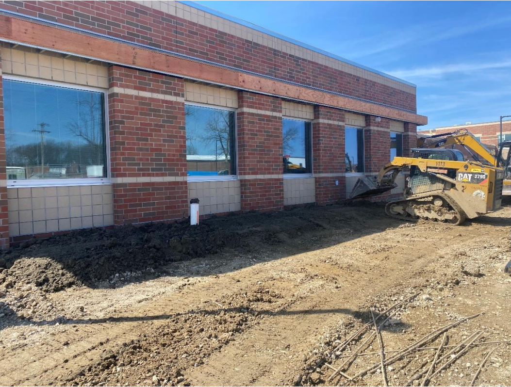
Topsoil is being installed in planted beds.
