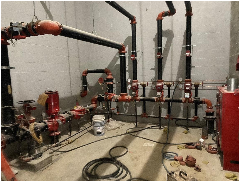
Fire protection sprinkler system main and branch lines are being air tested and then filled.
