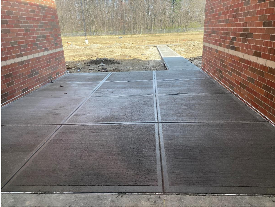
Concrete walks are being installed.
