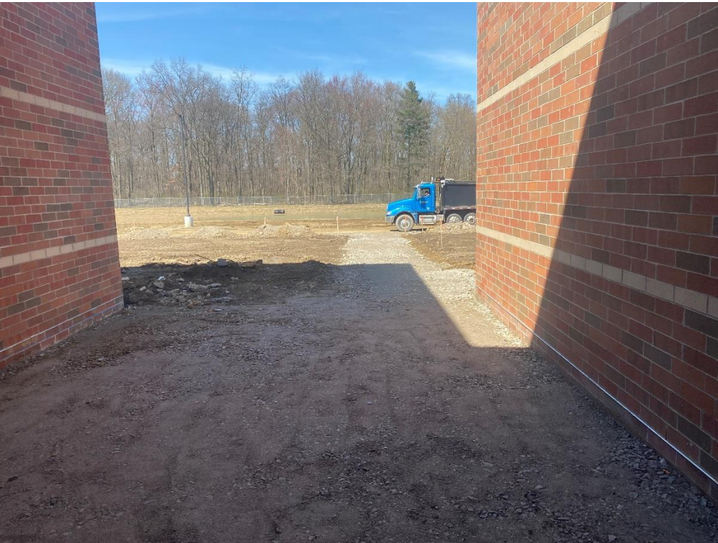
Stone base for sidewalks is being installed.
