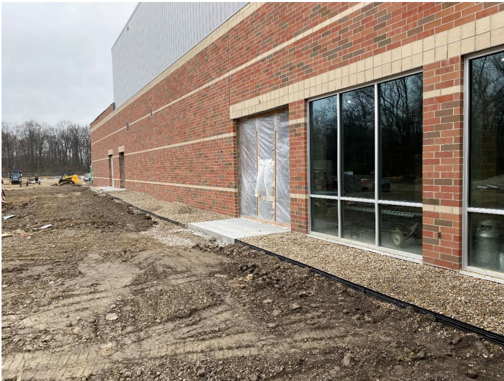
Washed river rock and landscape edging installed along the west wall.
