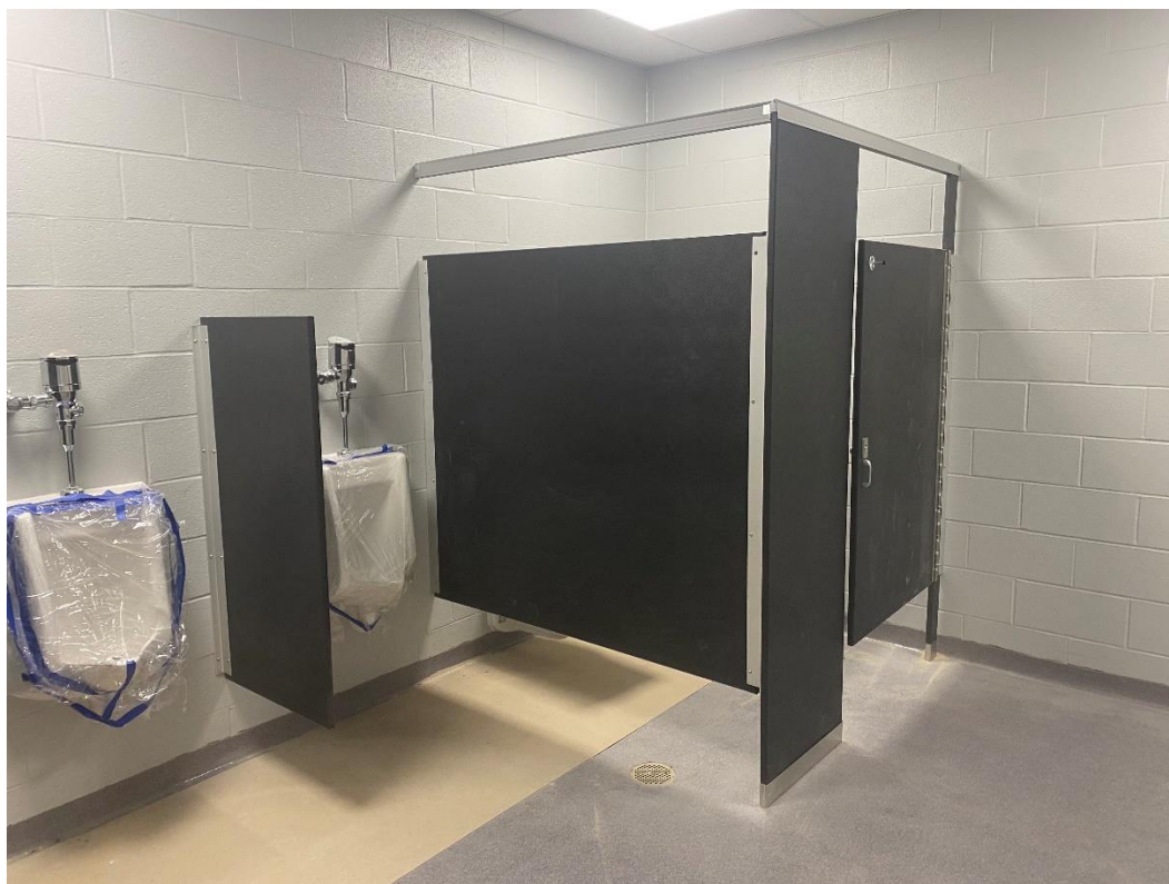
Toilet partitions are being installed.
