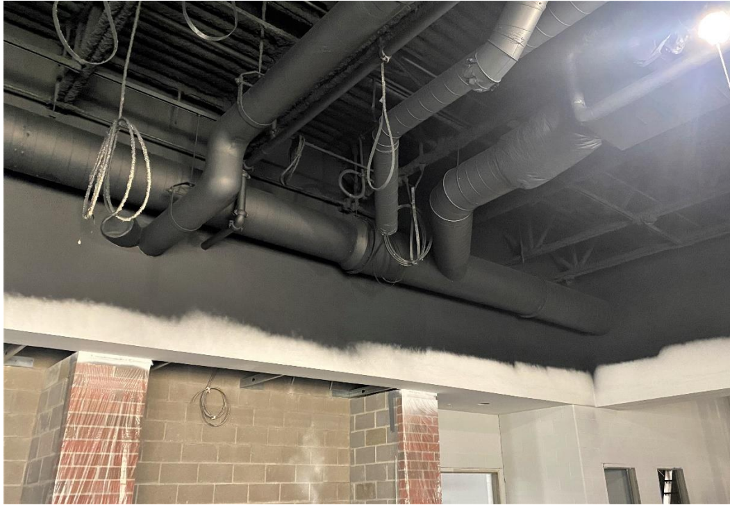
Exposed ceilings are being painted along with mechanical and electrical work in the Student Dining area.
