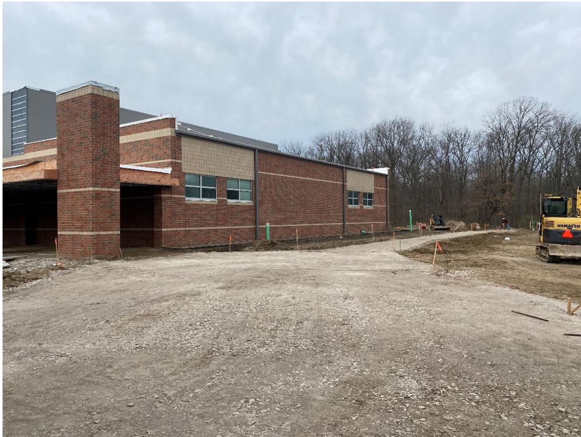
Stone base is installed for sidewalks at the north entry.
