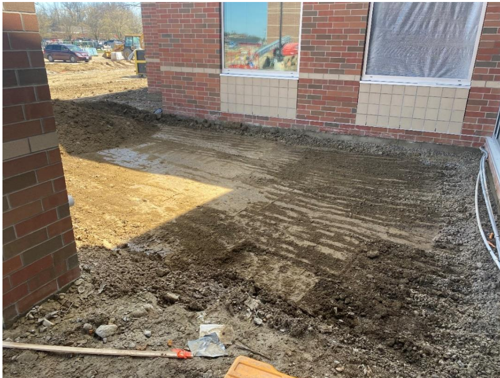
Planting beds are excavated and are being filled with topsoil.
