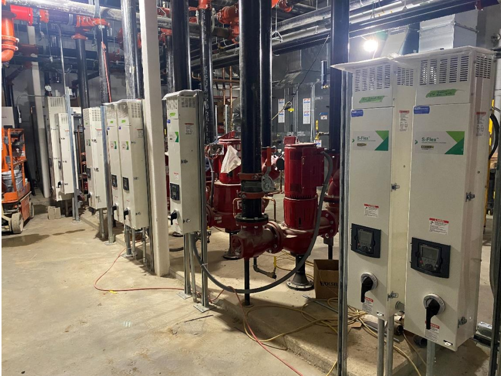
HVAC system control panels are installed.
