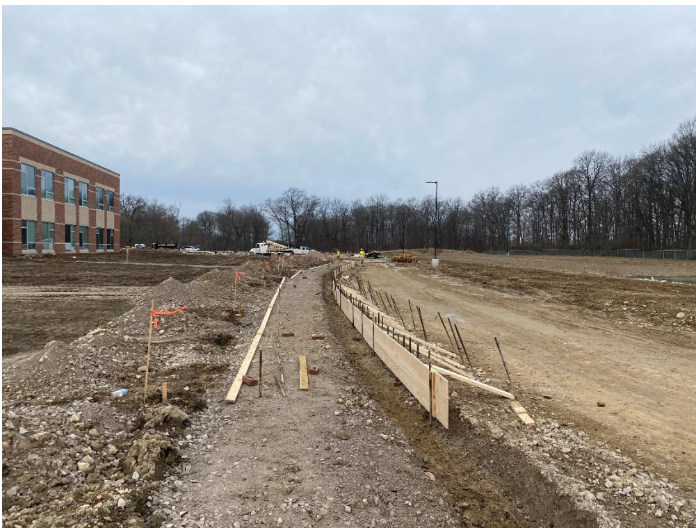
Curbs are being formed on the north side.
