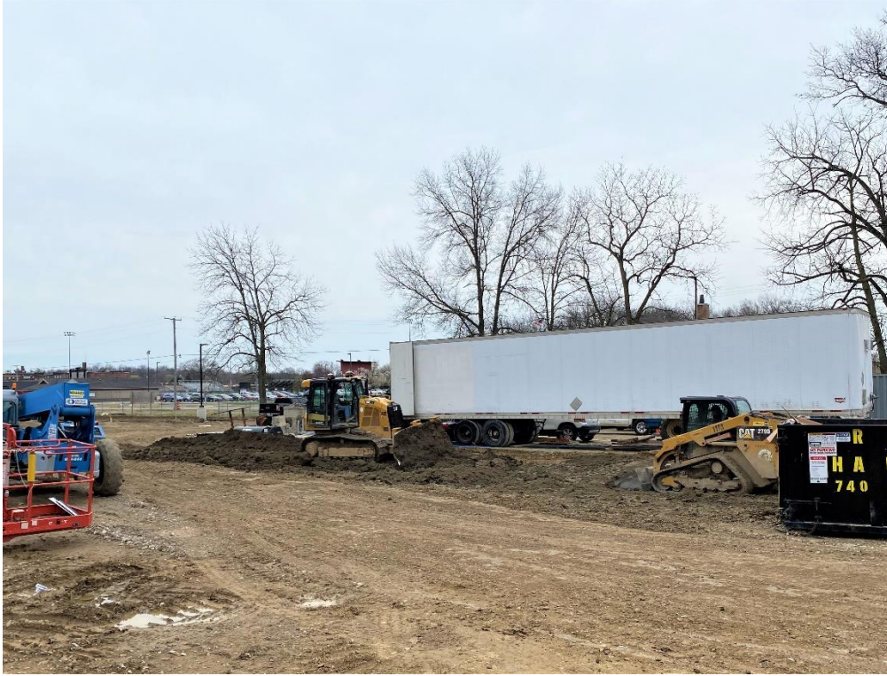
Topsoil is being placed and graded at the island, east side, visitor parking area.
