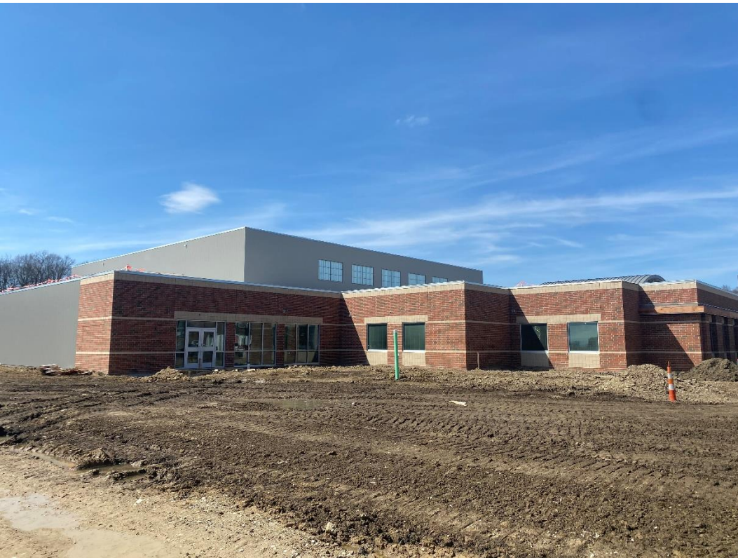
Rough grading continues in preparation for installation of the lawn.
