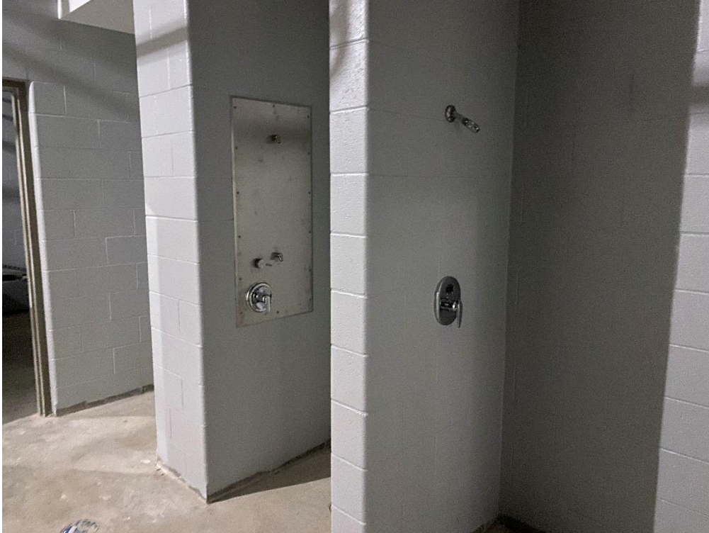
Shower fittings are installed in the Locker Rooms.
