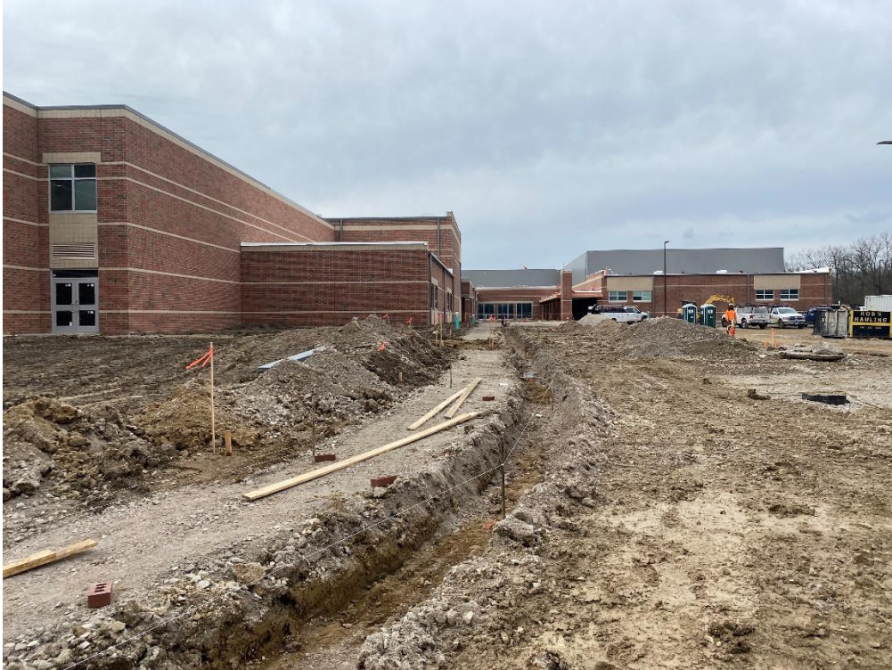
Excavation for curbs is complete and lines are site for forming on the north side.
