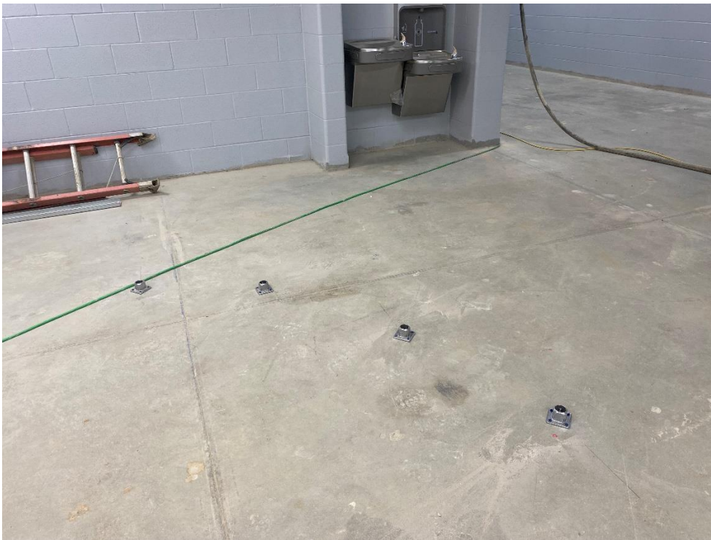
Inventionland panel bases are set for free standing display boards.
