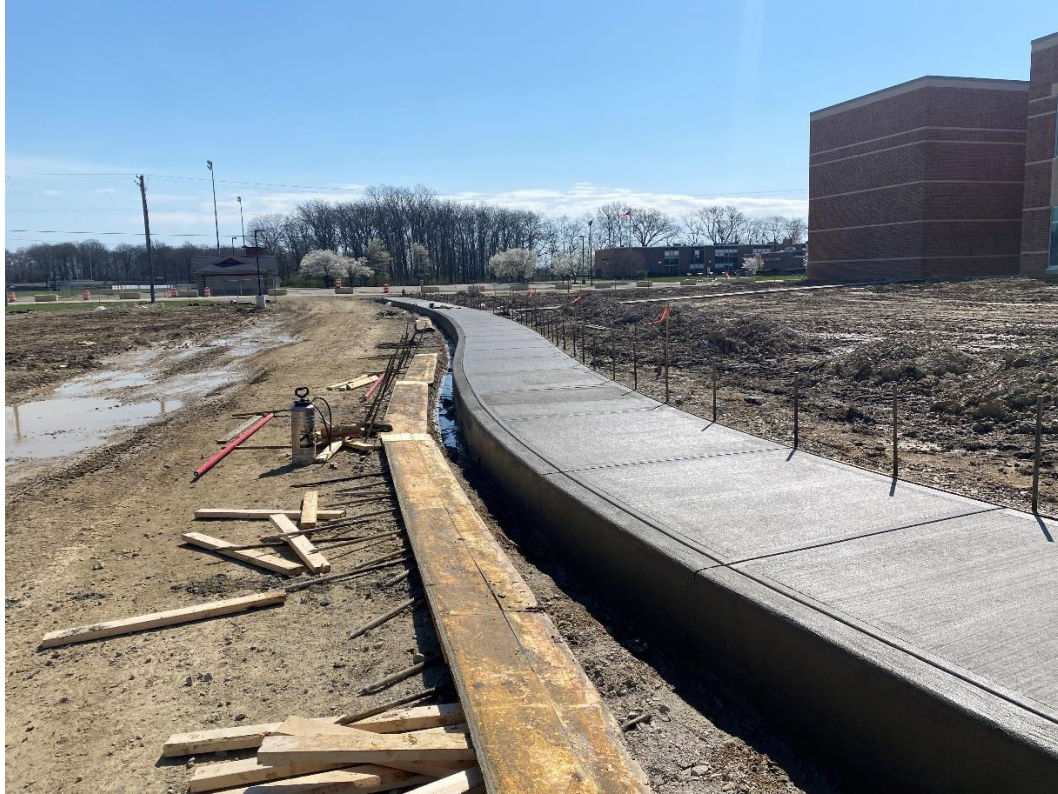
North side looking east. Forms are stripped from recently place concrete.
