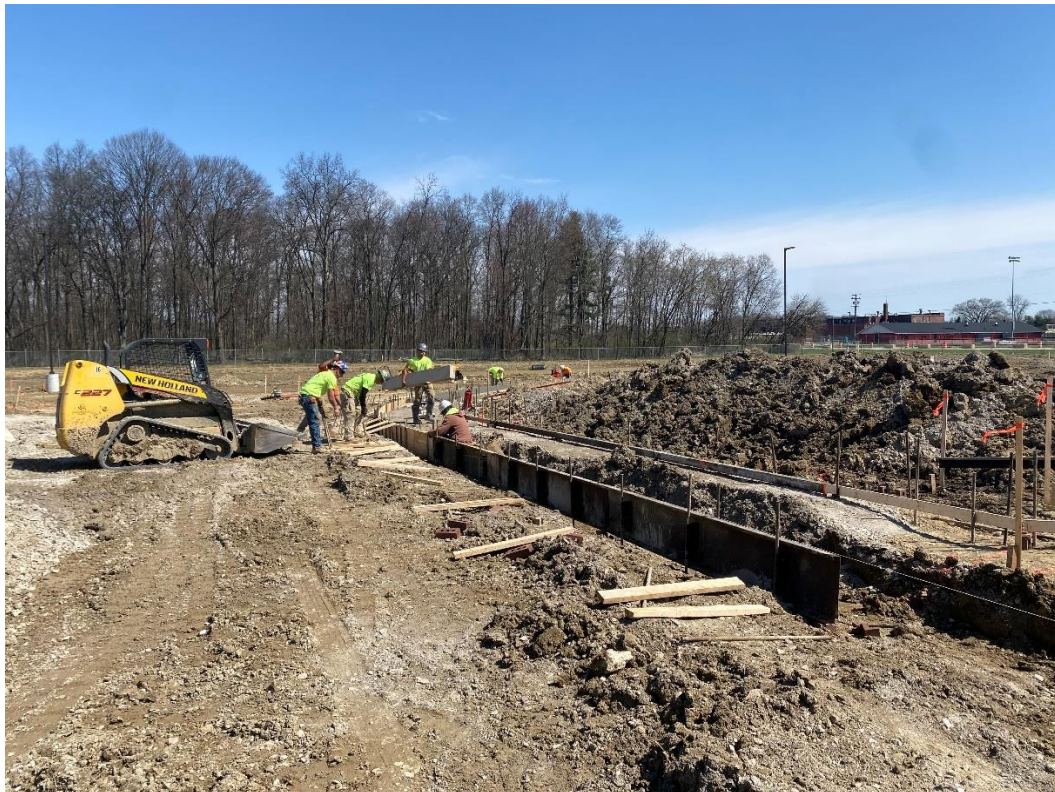
Forming of curb/walks continues on the NW side of the building.
