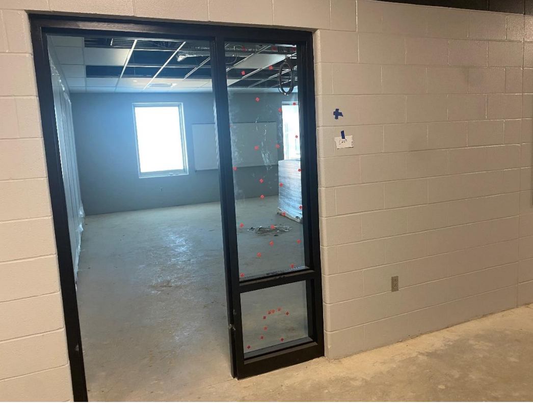
Glass is being installed in the side-lights of door frames.
