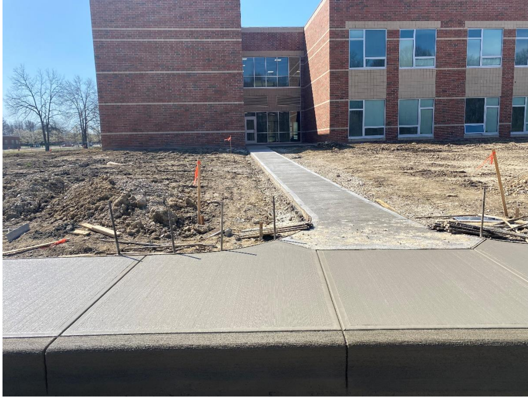
Combination curb/walk just recently installed. North elevation looking south.
