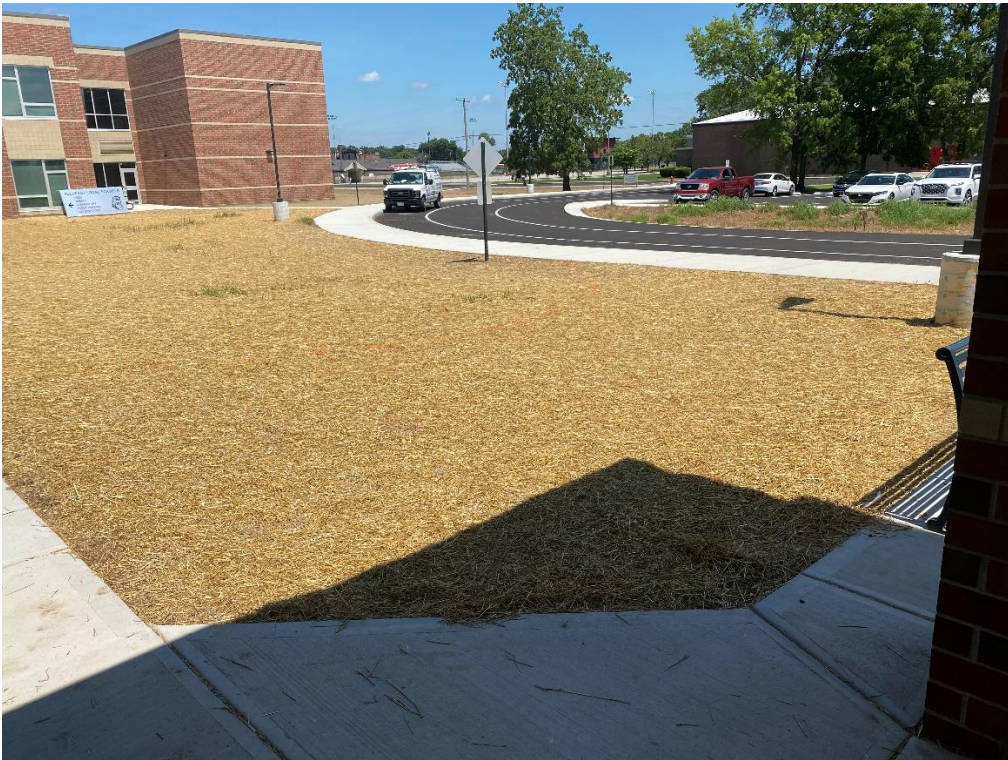
Lawn areas are being installed. Seeded areas will need to be removed at the front entry where landscape planting is planned.
