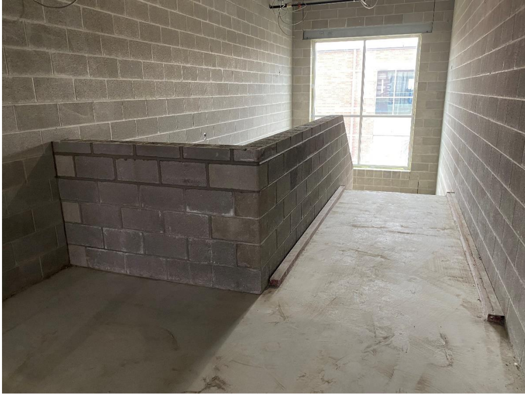
Masonry stair wall is complete at the south stair of Area D.
