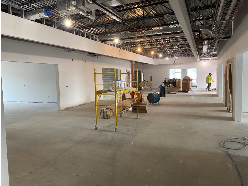
Prime painting of drywall is progressing at the second-floor of Area C.
