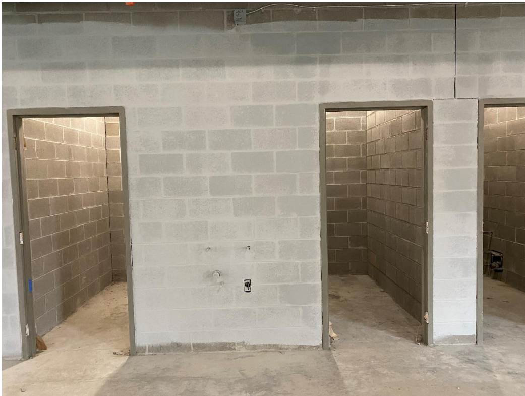
Interior masonry chase walls are complete in the toilet rooms at the second-floor, Area D. Block walls are receiving block fill primer.
