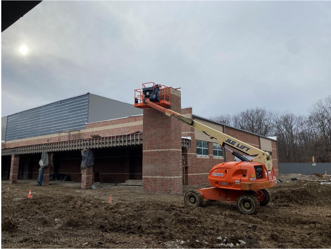
Exterior brick masonry is finished!
