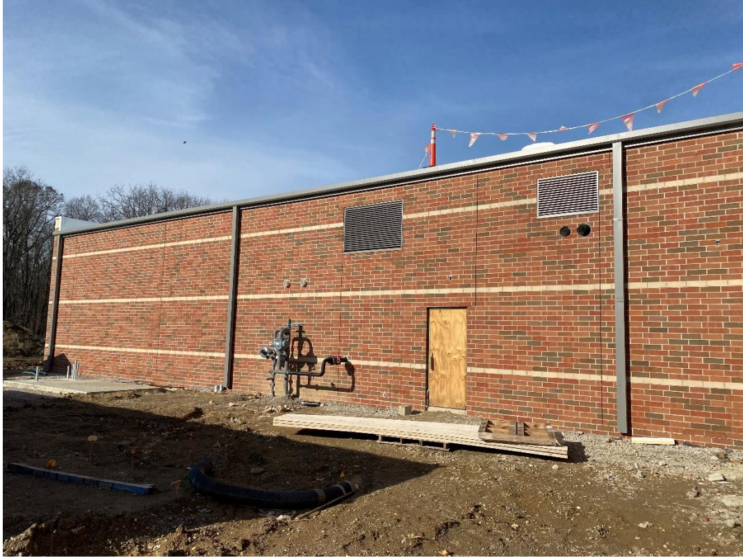
South wall of the main mechanical room. Brick is cleaned, and downspouts and louvers are installed.
