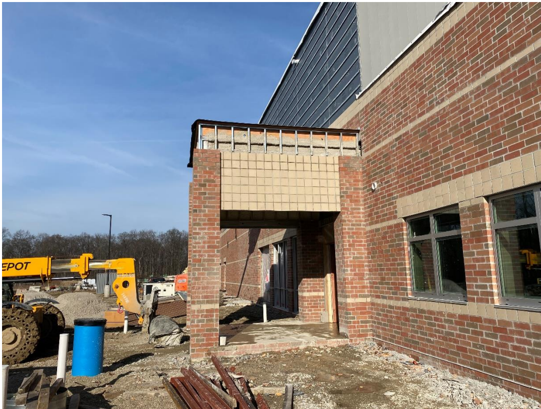
Brick masonry is complete at the west entry vestibule. Brickwork yet to be cleaned.
