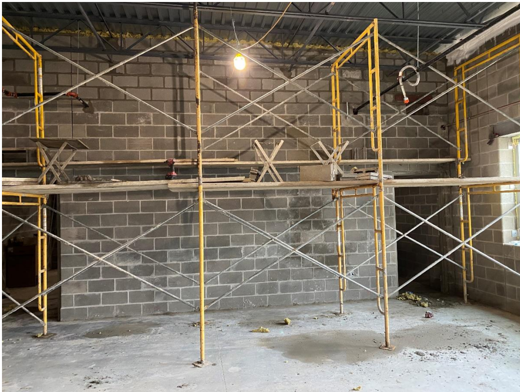
Non-load bearing interior partition walls are constructed in Area B
