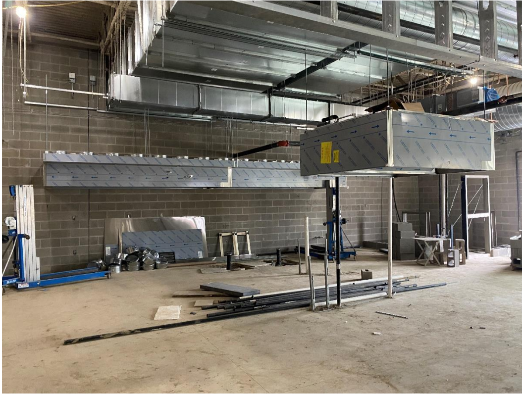
Kitchen exhaust hoods are installed.
