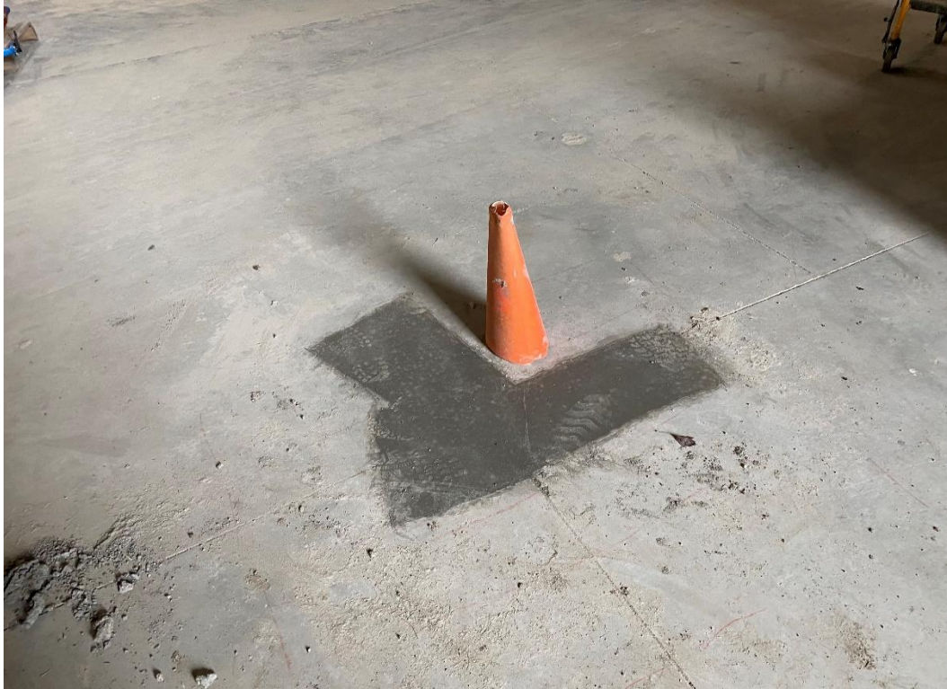
Floor is patched at the base of the main stair to the second-floor of Area C & D where an outlet was required to be removed.
