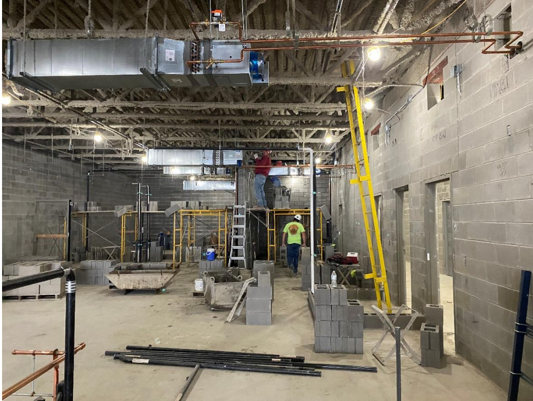
Construction of non-bearing masonry partition walls is progressing in the Locker Rooms.
