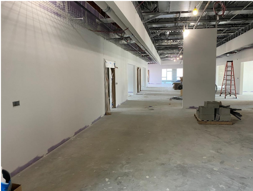
Second -Floor Area D, view looking east.
