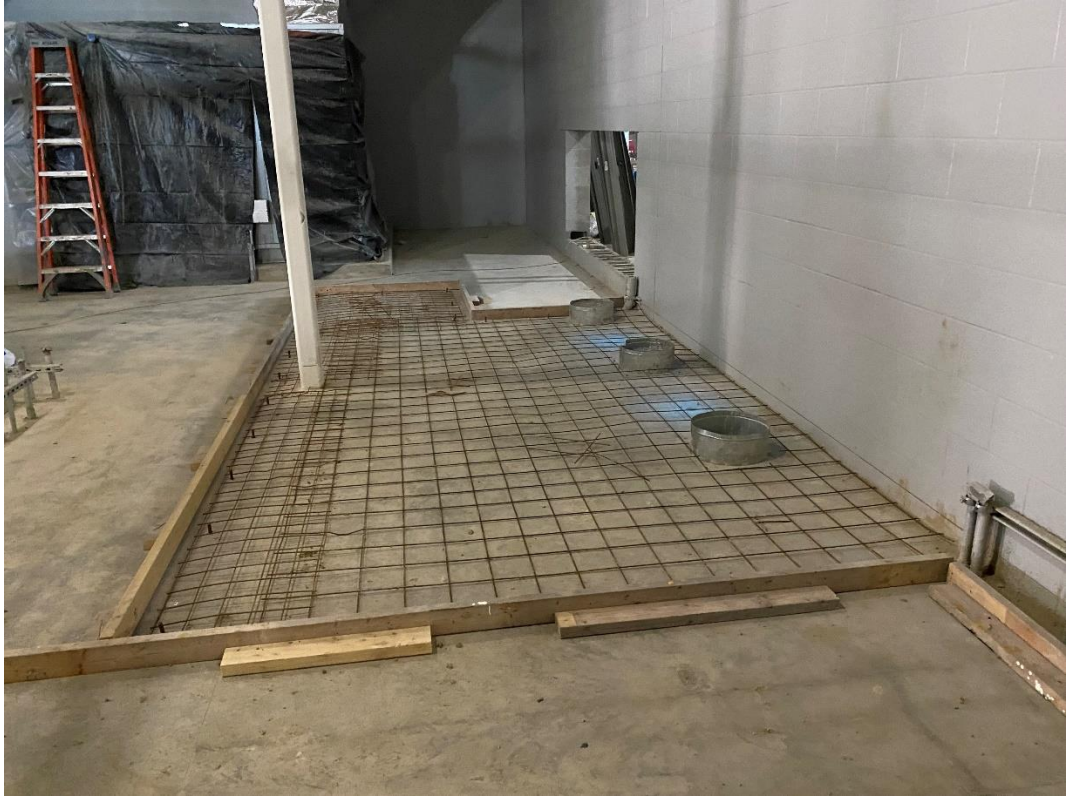
Concrete pad is formed with reinforcing installed for the HVAC Boilers.
