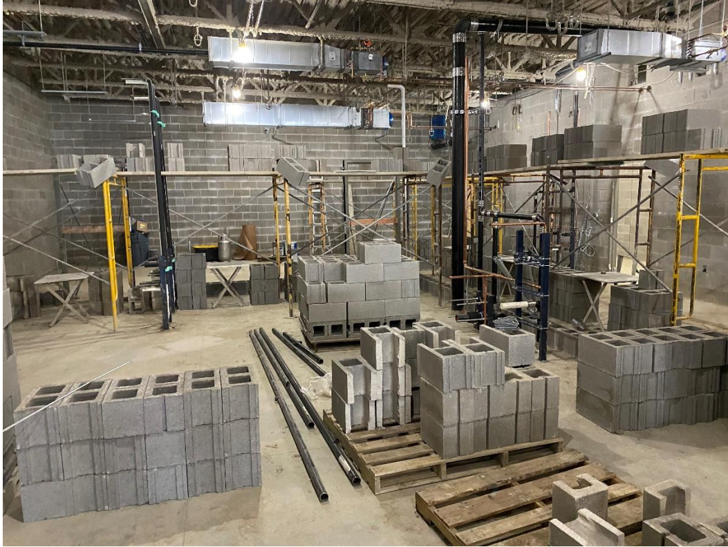
Concrete masonry walls progress in the main toilet rooms of Area C, first-floor.
