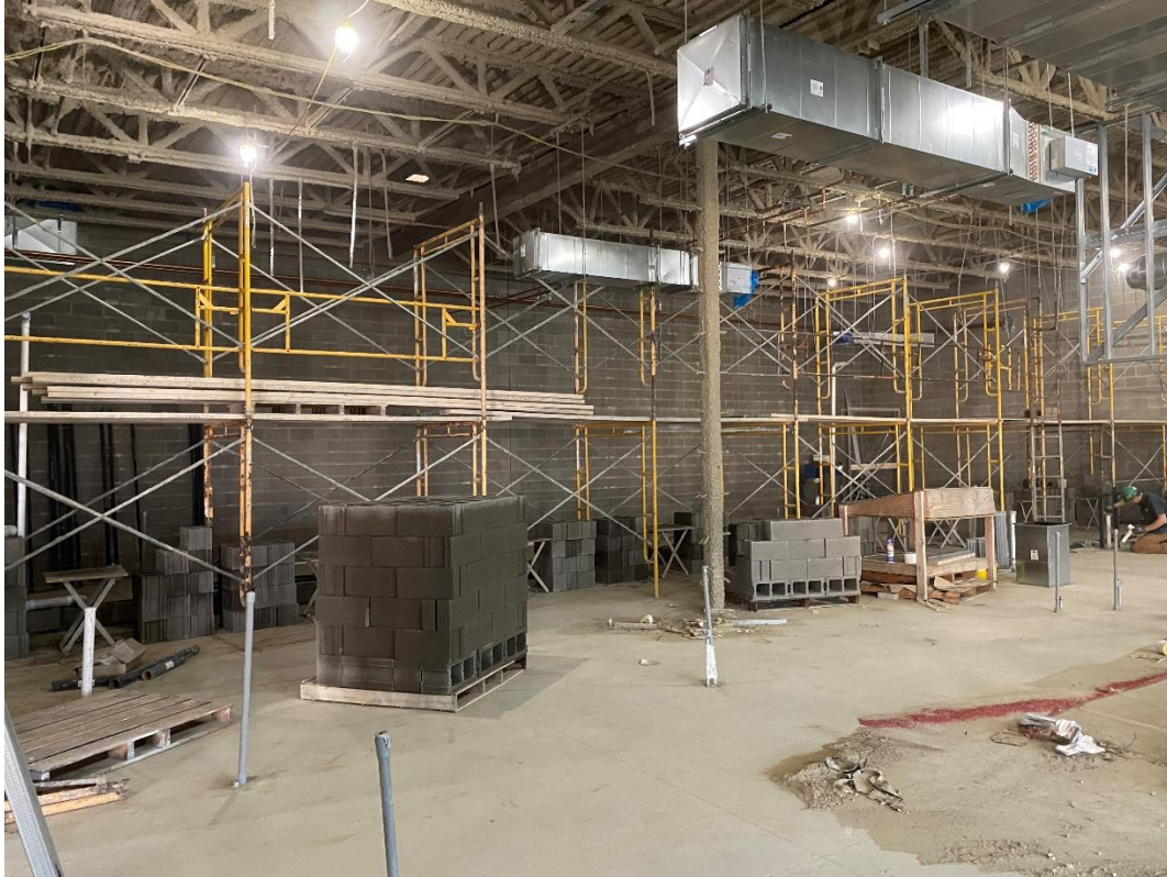
Scaffolding is erected for construction of the masonry wall at the freezer/cooler in the Kitchen.
