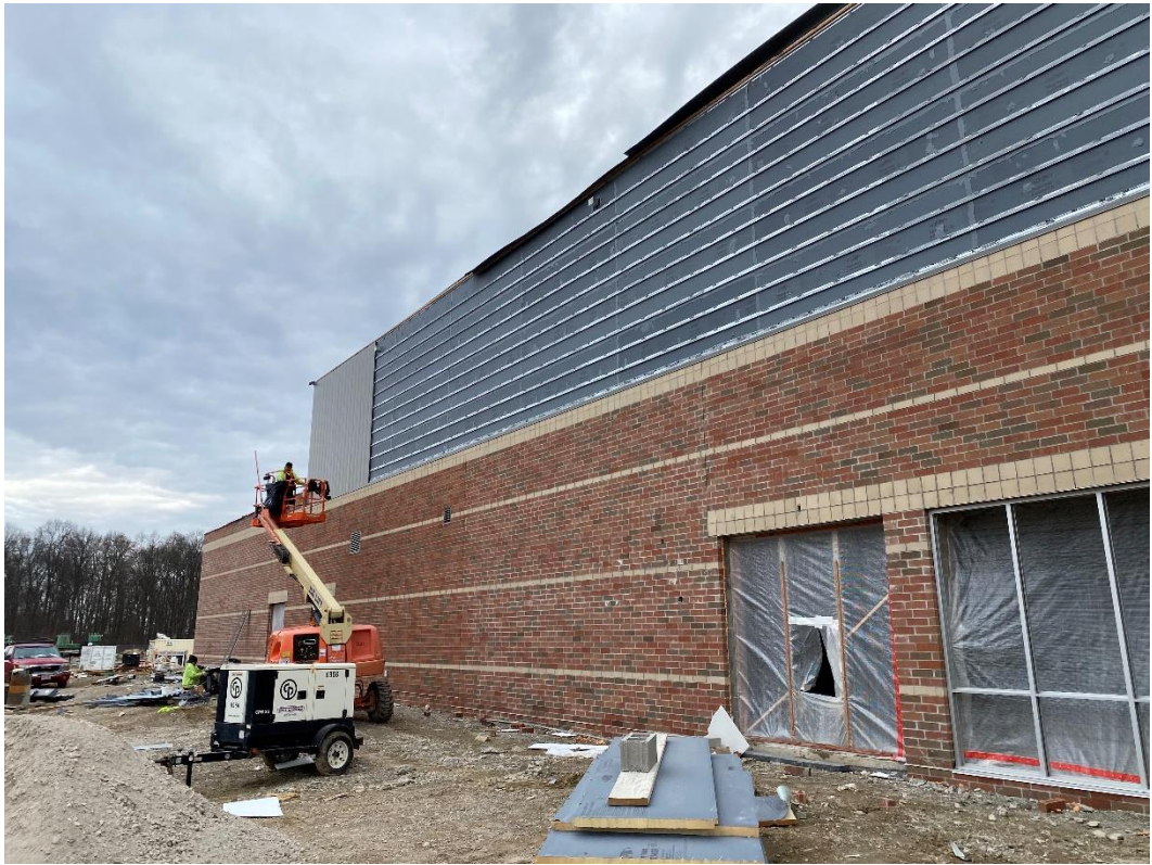
Installation of metal siding panels continues on the west side of the performing arts center.
