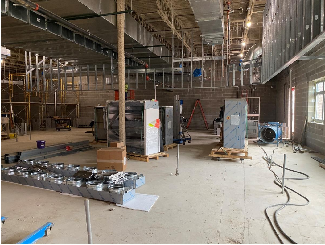
Sections of kitchen exhaust hood are staged for installation.
