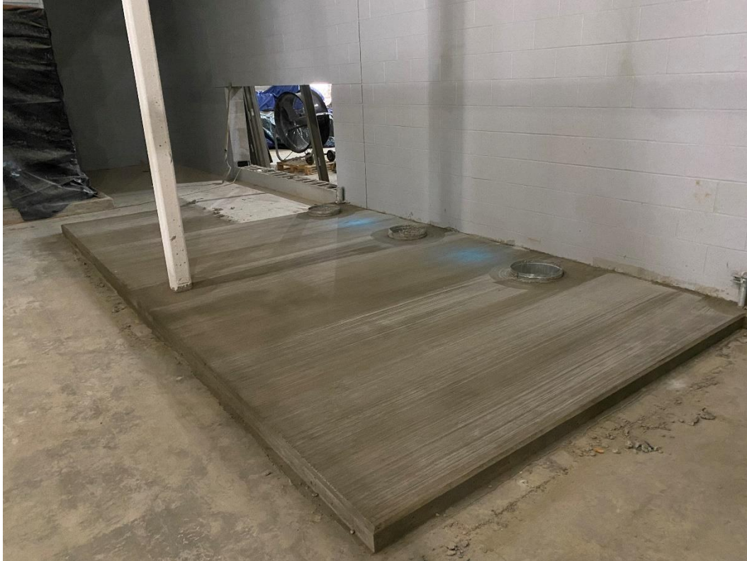
Housekeeping pad for the HVAC boilers is installed.
