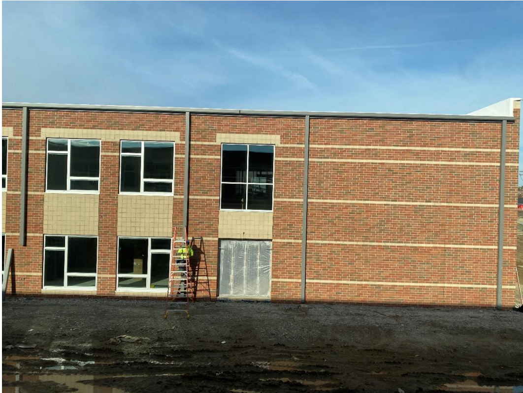
Work on gutters and downspouts continues at Classroom Area D.
