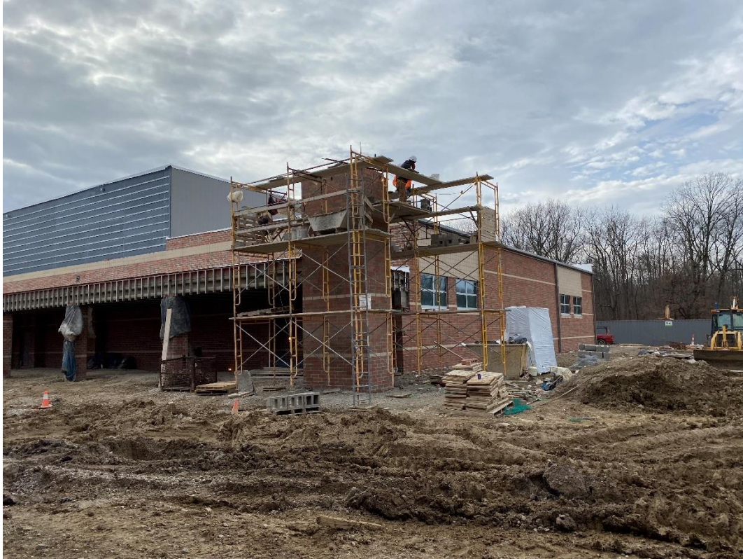
Brick masonry continues at the NE corner of the north entry canopy. When finished, all exterior brickwork will be complete.
