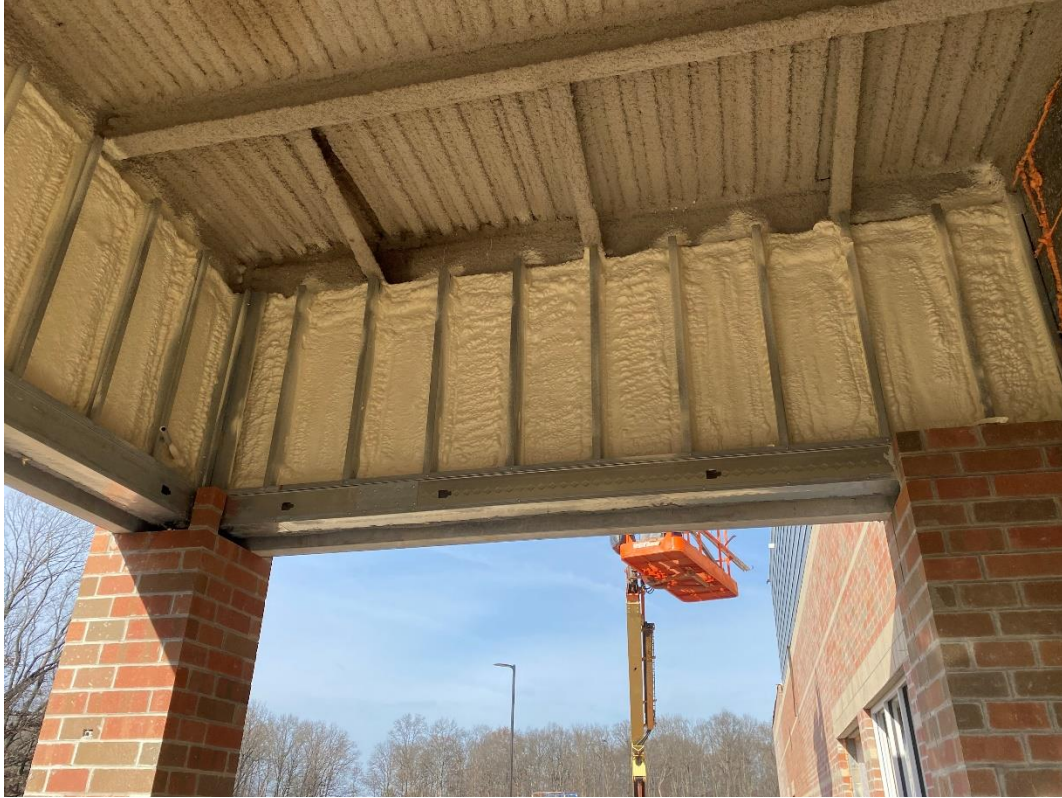
Fireproofing and spray foam insulation is complete at the west entry vestibule.
