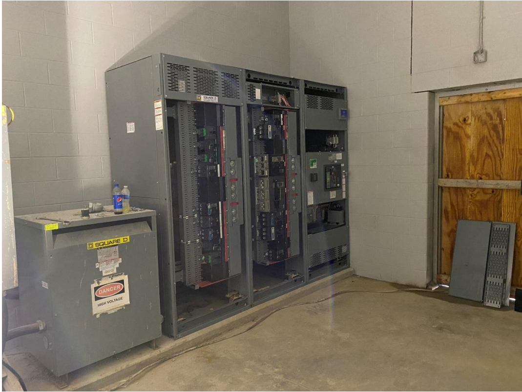
Sections of main electrical switchgear are installed.
