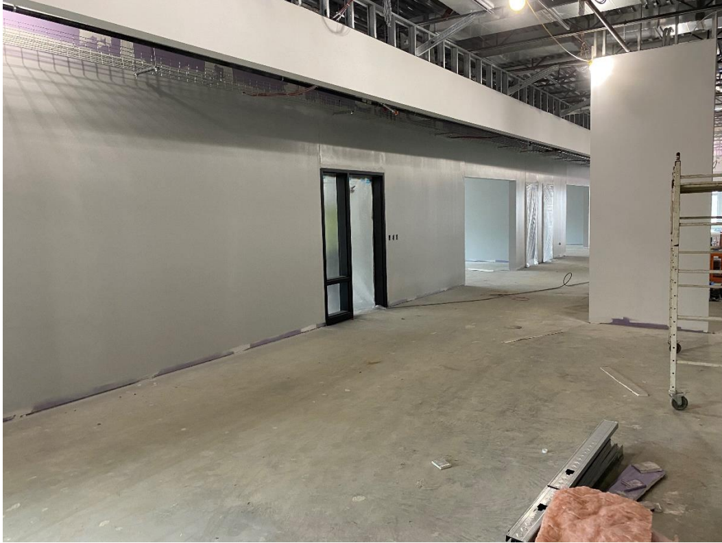
The first finish coat of paint on drywall has started in Area D, second-floor.
