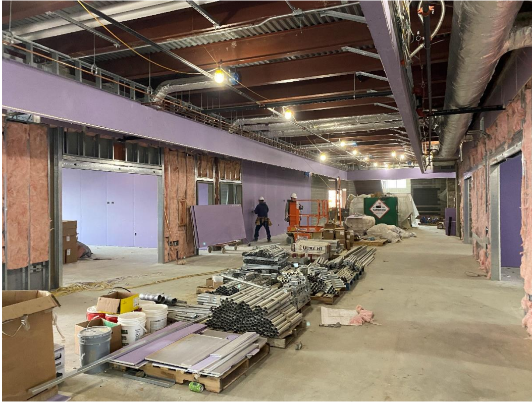
Drywall installation is 60% complete at the first-floor of Area C.
