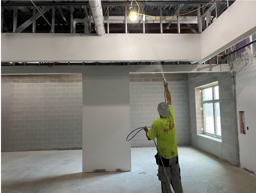
Prime painting of drywall continues at the second-floor, Area D.
