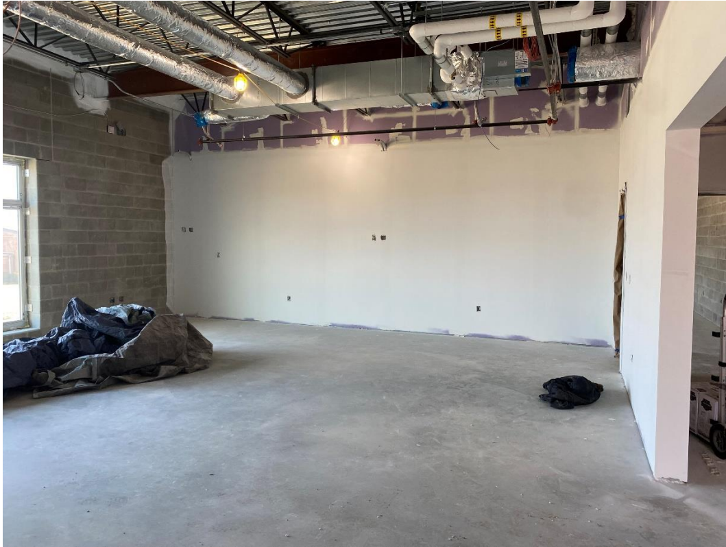
Prime painting of drywall is progressing at the Second-Floor of Area D.
