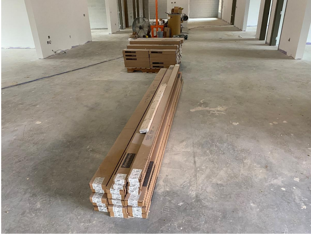
Suspended ceiling grid is staged for installation at the second-floor of Area D.
