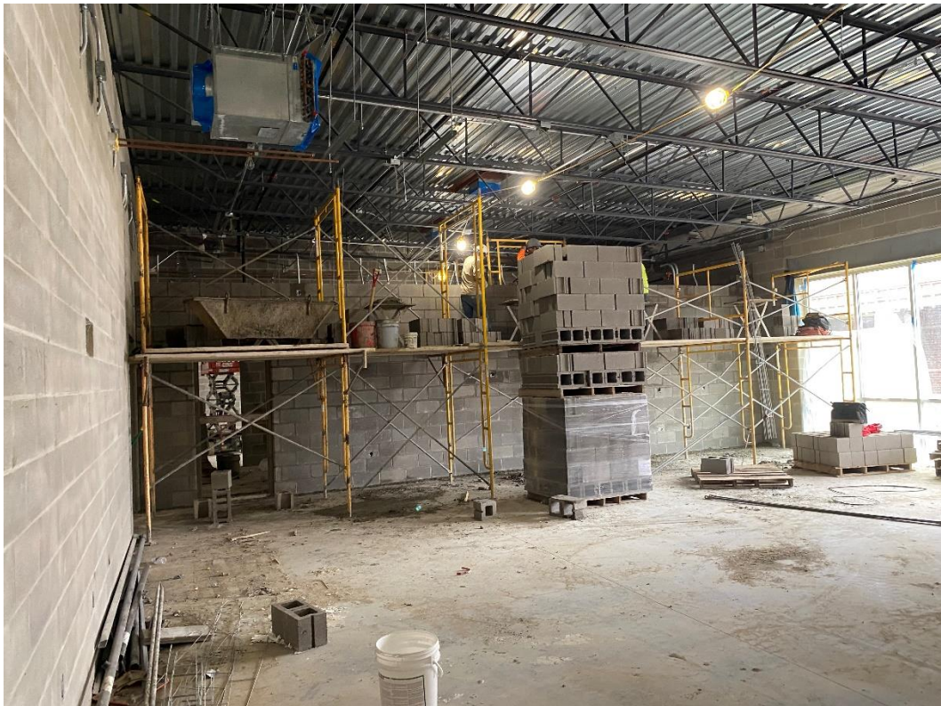
Interior masonry walls at the Art classrooms is nearly complete.
