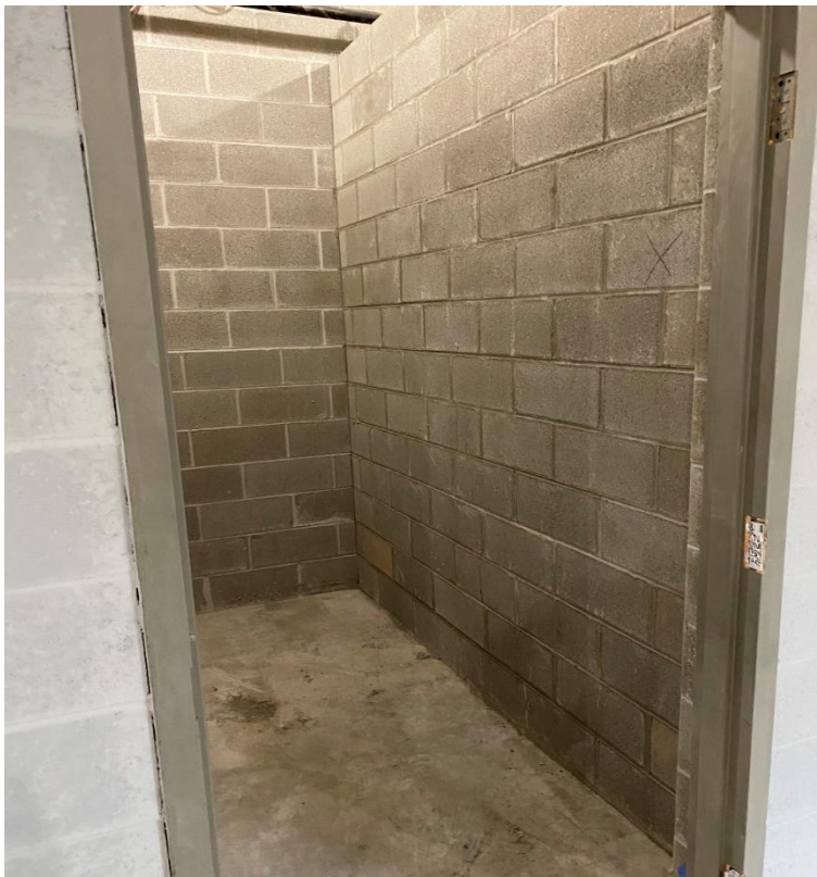
Masonry chase walls are complete in Area D toilet rooms.
