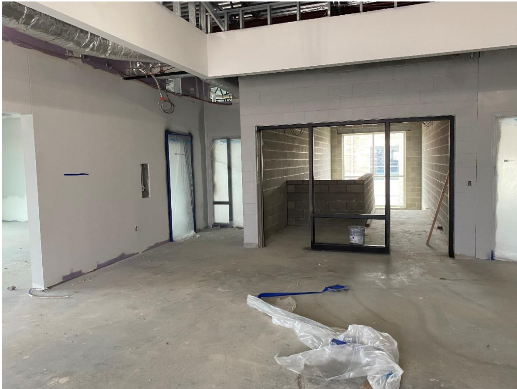
Painting of metal door frames has started in Area D.
