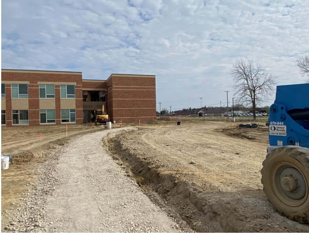
Curbs and walks are being prepared for concrete forming.
