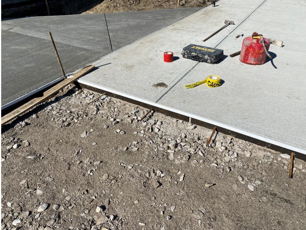
Sidewalk slabs are doweled at expansion joints.
