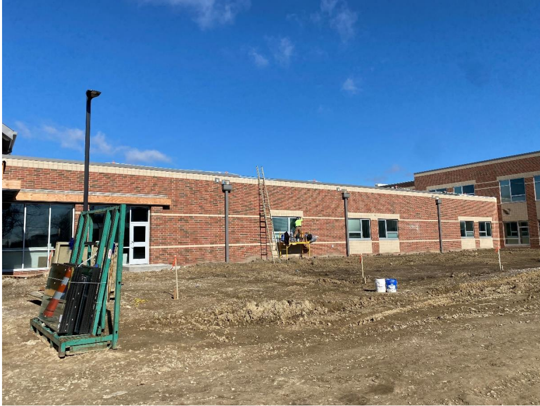
Caulking and sealants are being completed at window openings.
