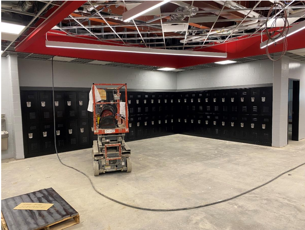
Locker installation is nearly complete in Areas C & D.
