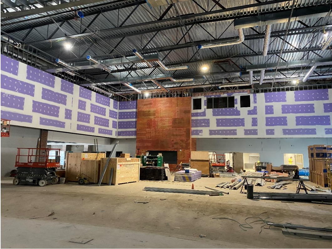
Drywall is being taped and finished in the performing Arts Center.
