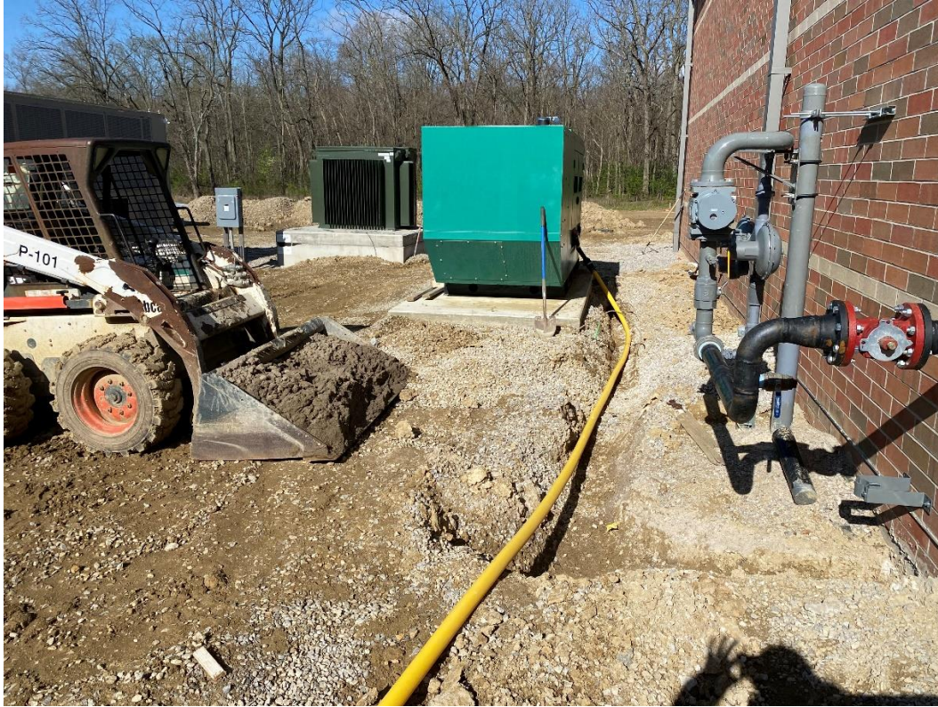
Gas line to the emergency generator is being installed.
