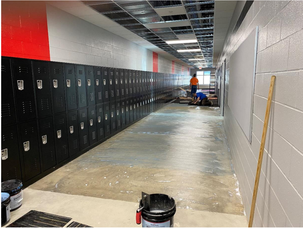
Carpet is being installed in the second-floor, Area C/D main corridor.
