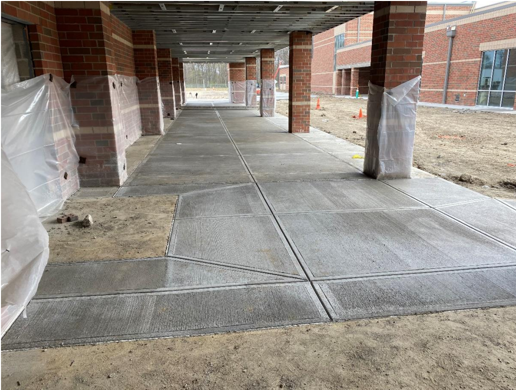
Concrete walks at the north event entrance are complete.
