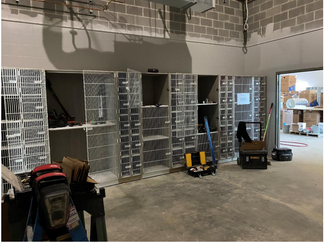
Instrument locker installation at the Instrument Storage room.
