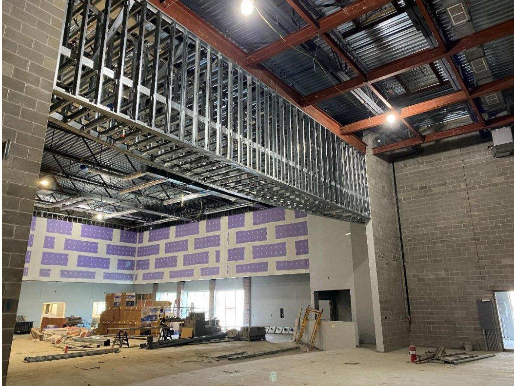
View of soffit at stage level looking SW.
