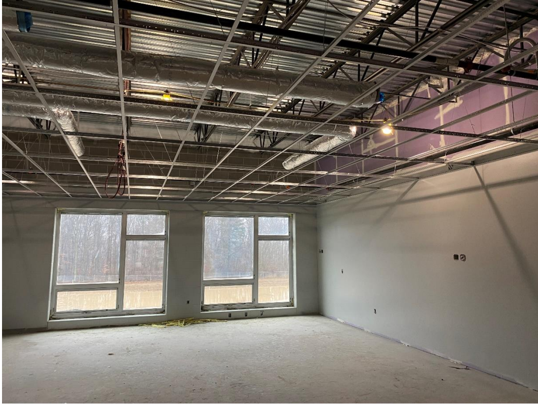
Suspended ceiling grid is installed in all the second-floor classrooms of Area D.
