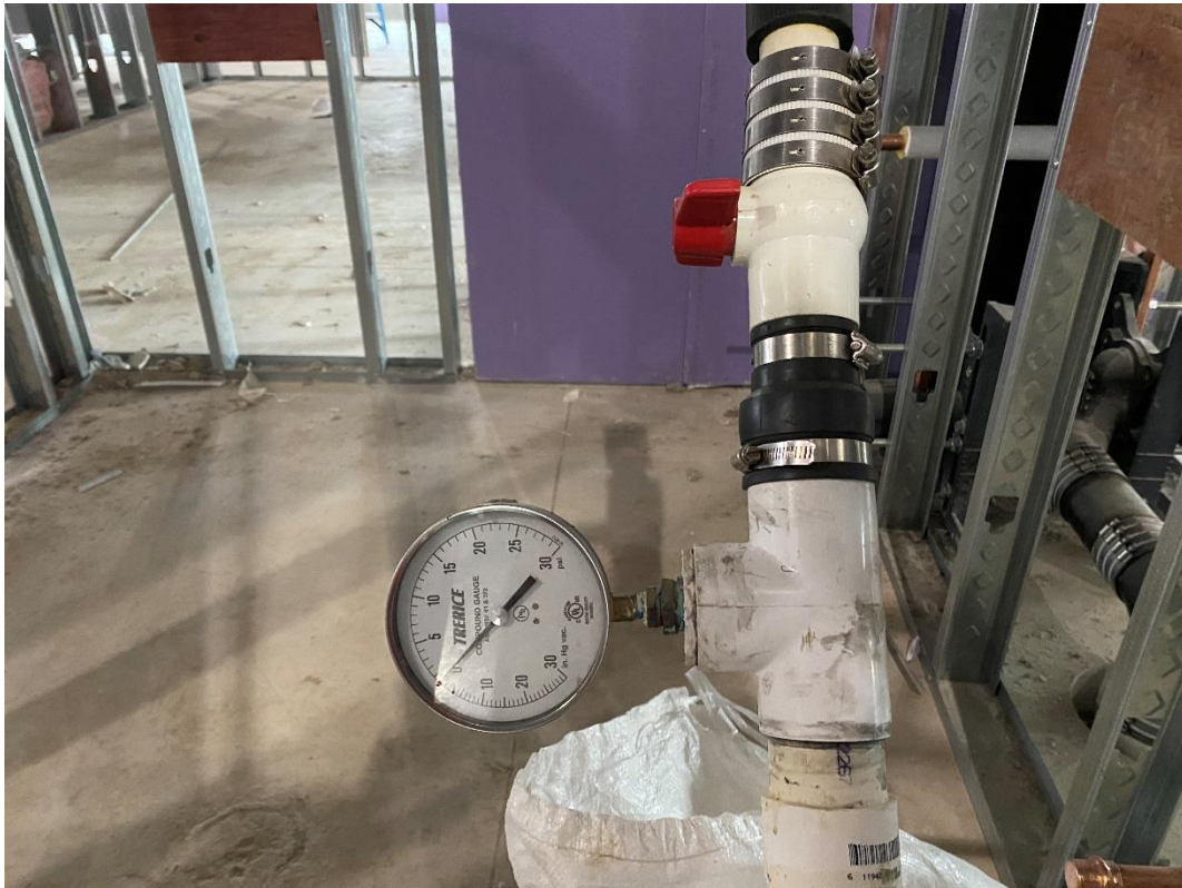
Air test on plumbing lines in the Administrative Offices.
