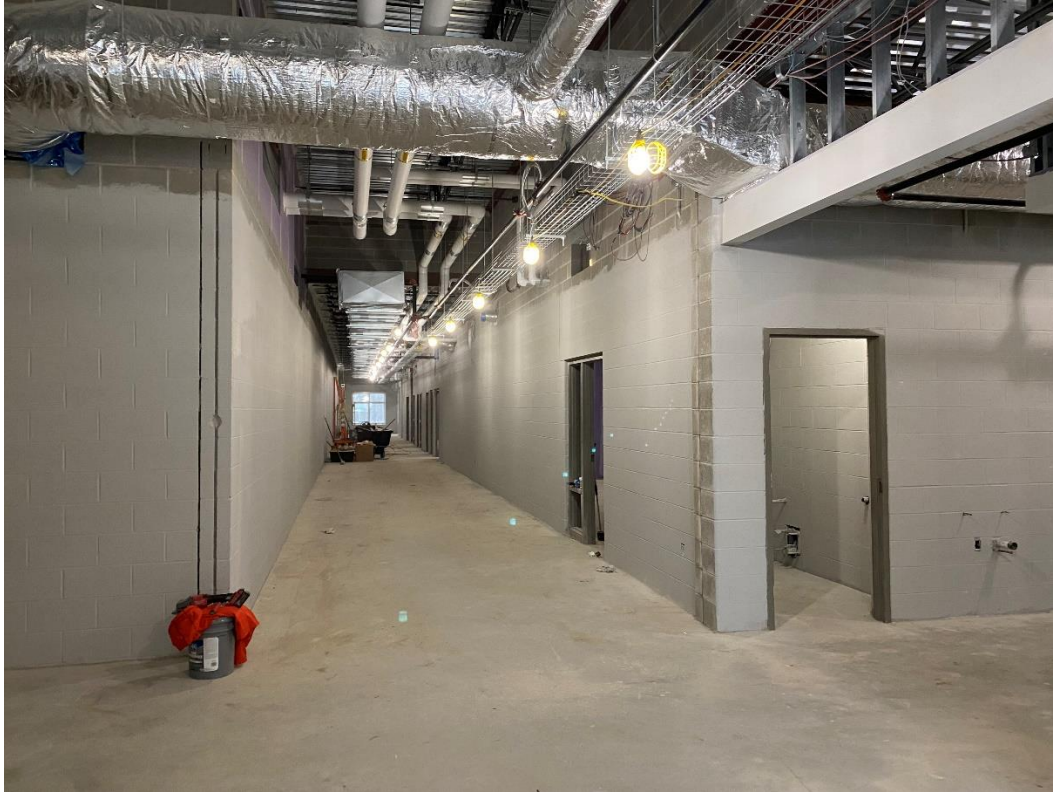
Main corridor at Area C is prime painted.
