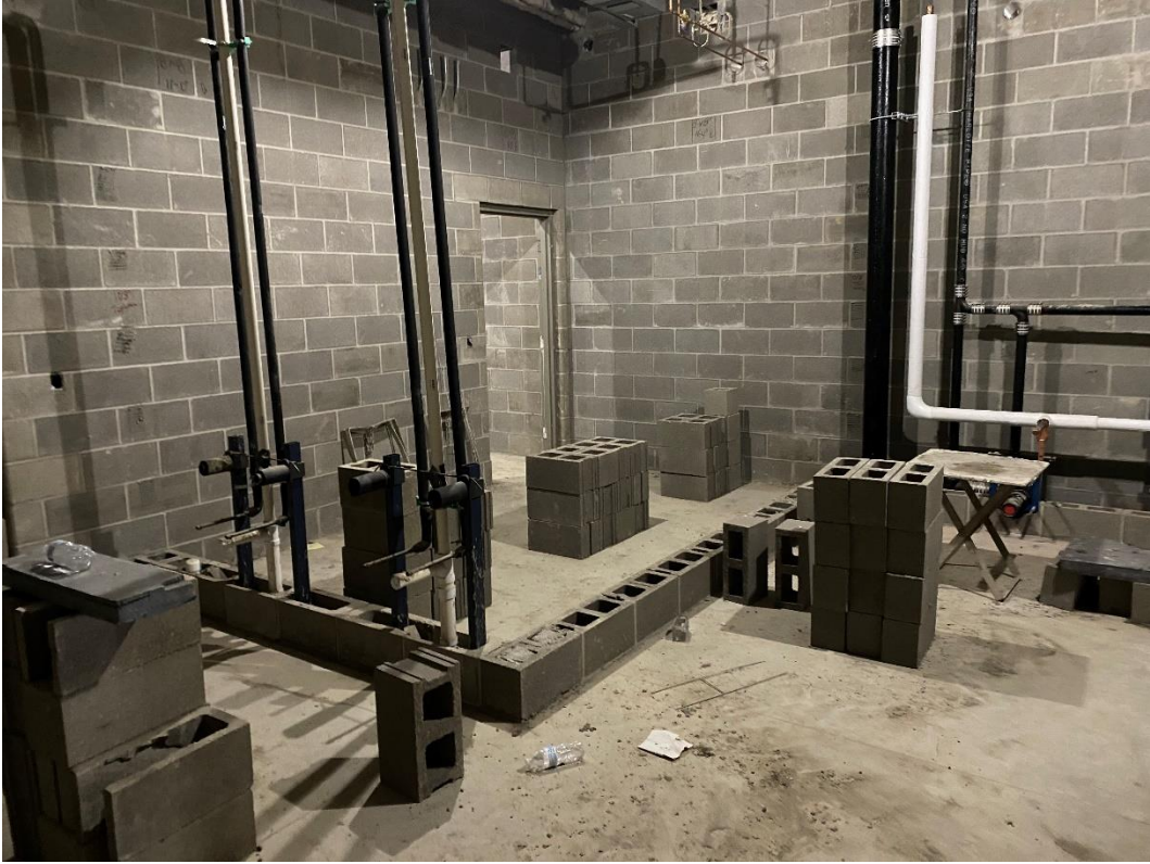
Construction of interior masonry walls is progressing in the Locker Rooms.
