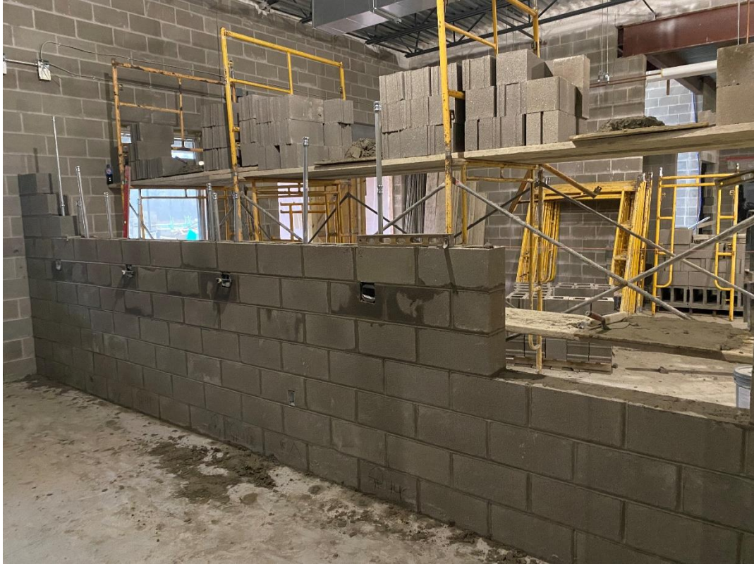
Interior masonry walls at the Technology Workroom, Area C, are progressing.
