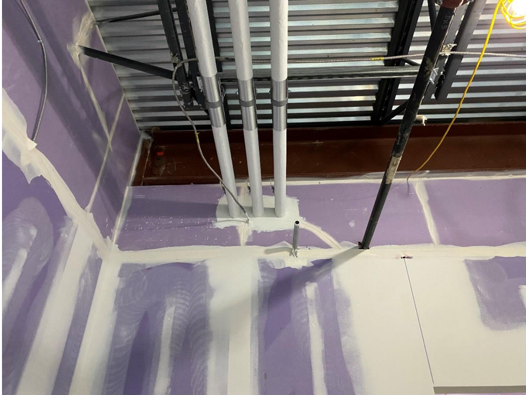
Pipe penetrations are being sealed where passing through drywall partition walls.
