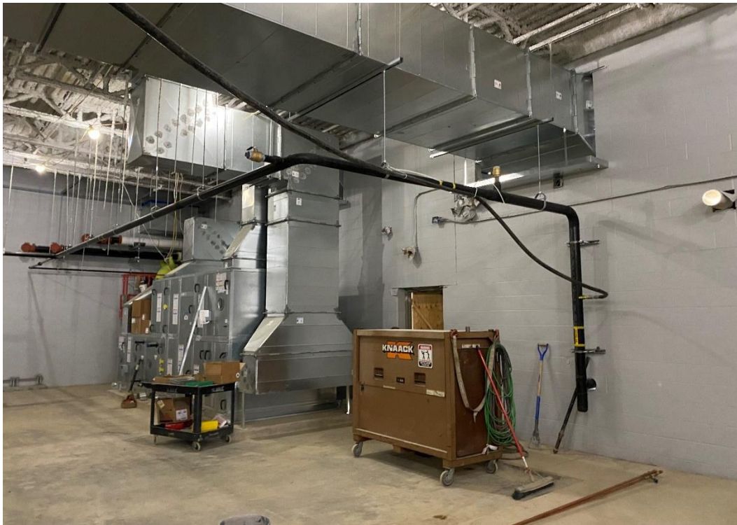
Installation of gas lines is progressing in the main mechanical room.
