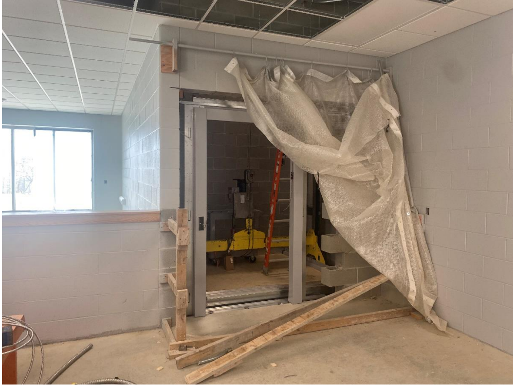
Elevator doors are being installed at both levels.
