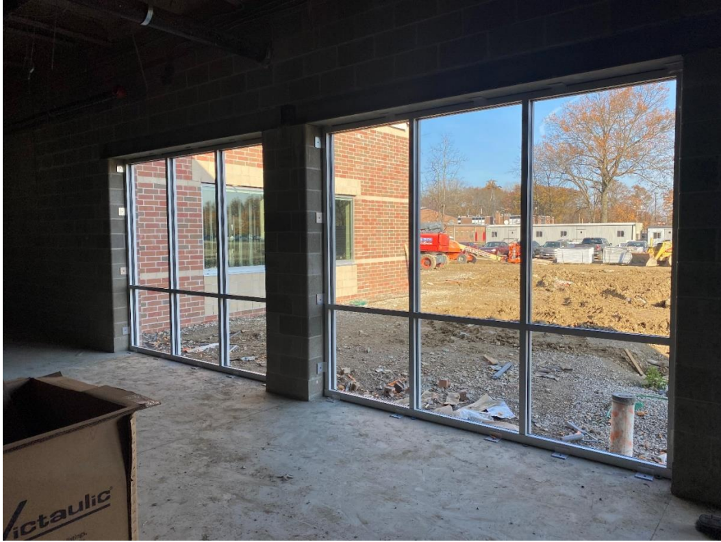
View looking east from the east corridor at the Locker Rooms.
