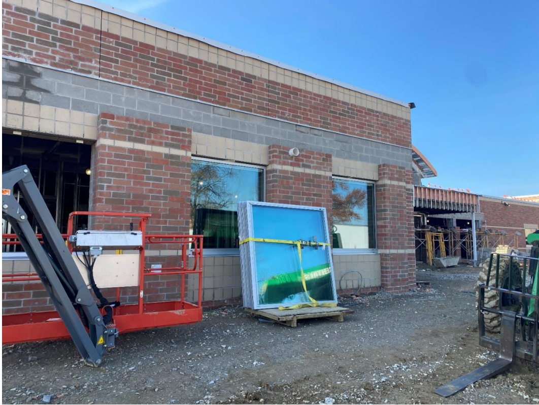
Windows are being installed on the east side of the Administrative Offices, Area A.
