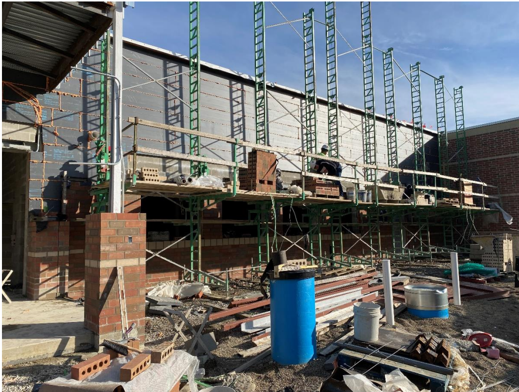
Brick veneer at the west wall of the kitchen is 25% complete.
