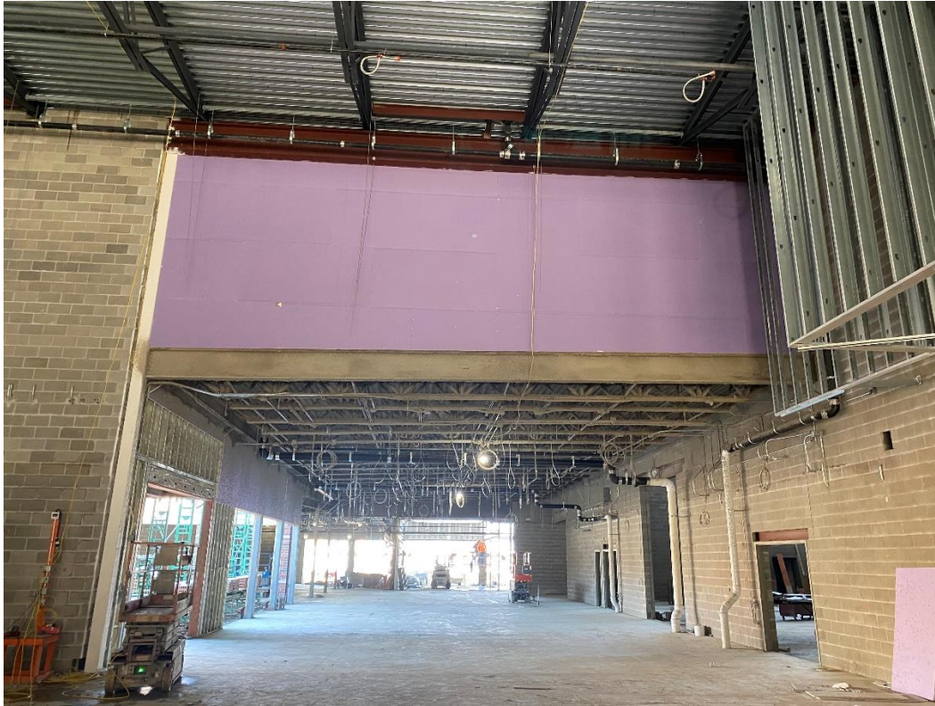
Moisture resistant drywall is installed on the upper east wall of the Performing Arts Center.
