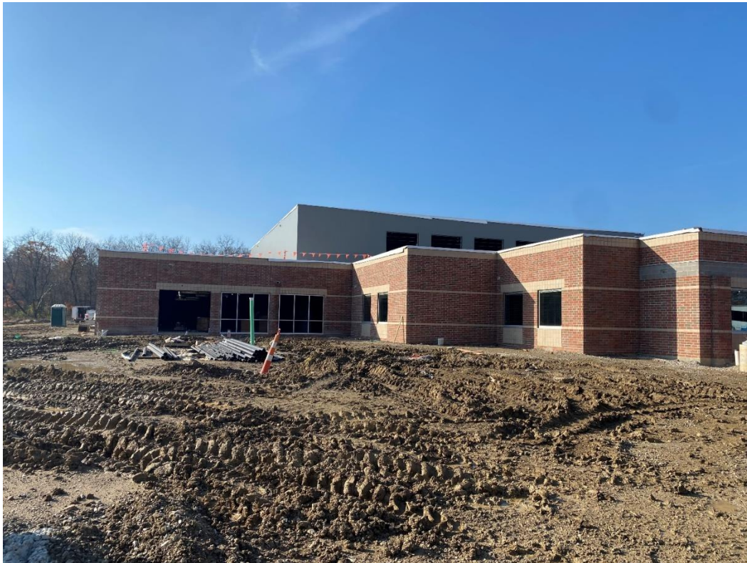
Installation of windows continues on from Area A to the east corridor wall at the Locker Rooms.
