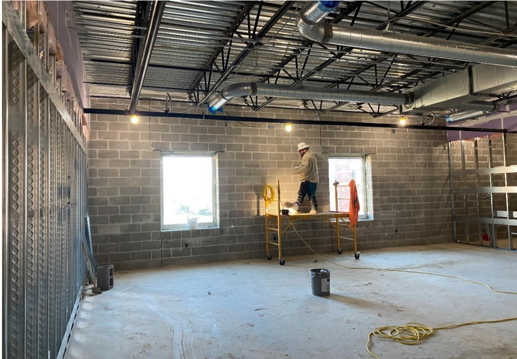
Masonry walls are being cleaned and minor imperfections pointed in preparation for painting.
