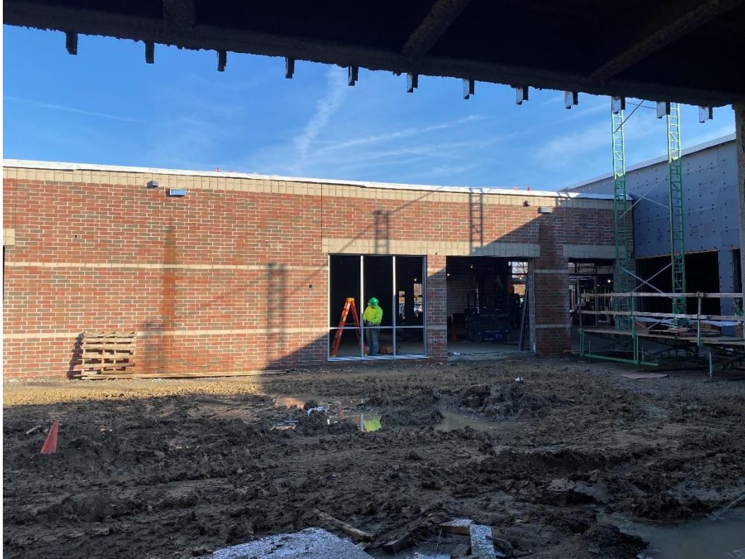
Windows are being installed at the Engineering Lab, Area B.
