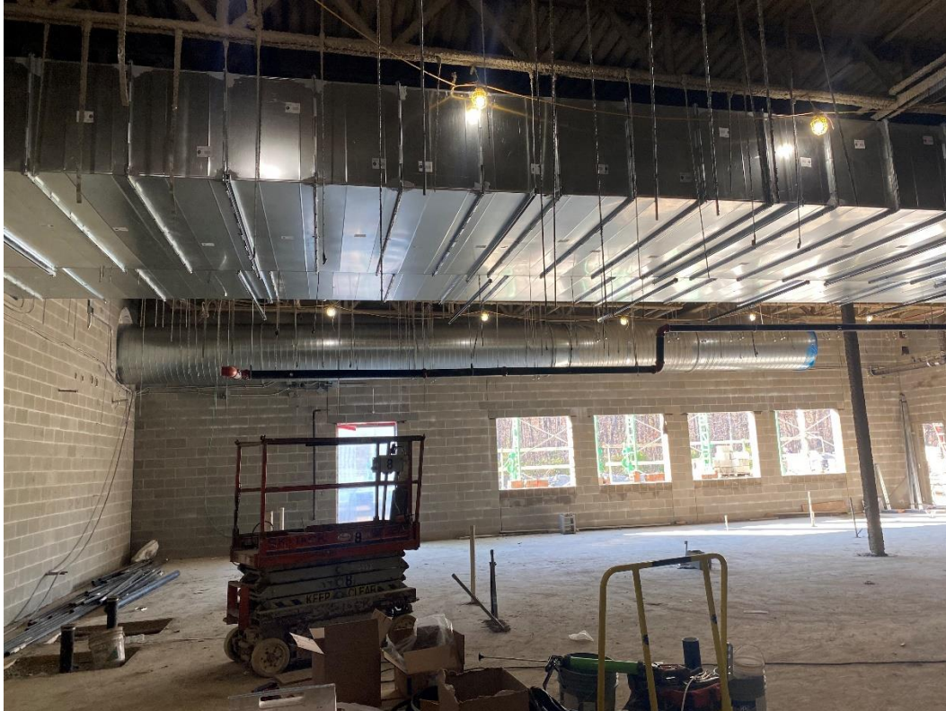
Large main ducts are extended through the Kitchen into the Performing Arts Center.
