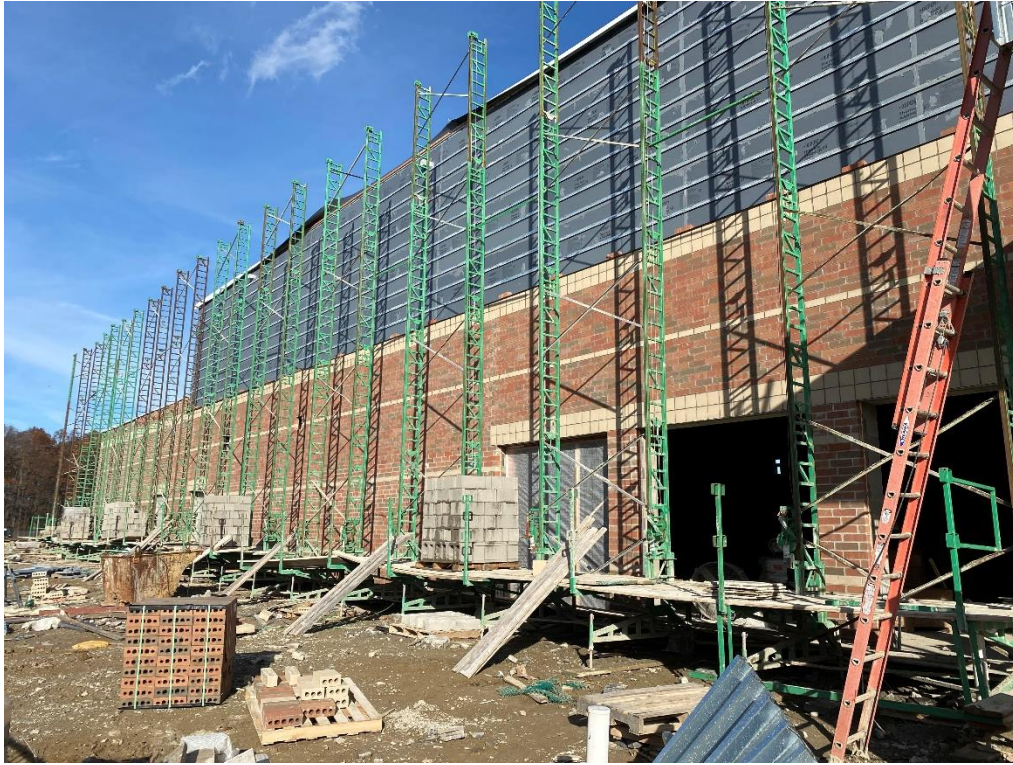
Brick veneer at the west wall of the performing arts center is complete. Metal siding panels will be installed on the upper wall area.
