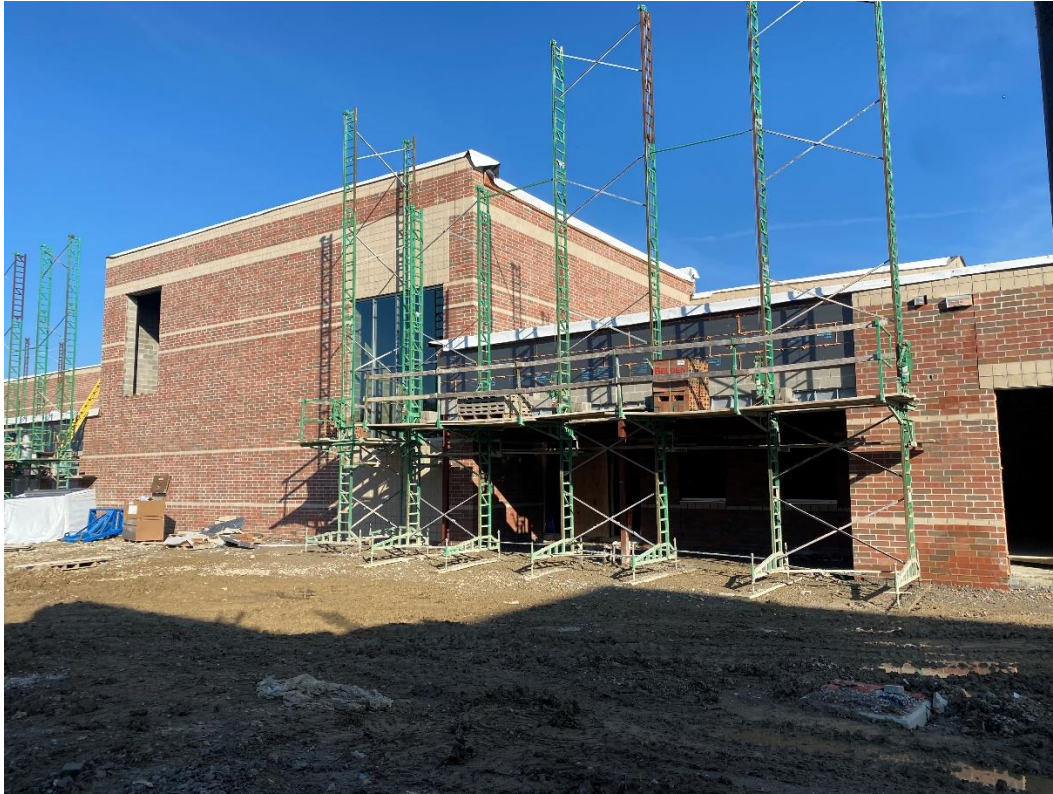
Brickwork is nearly complete at the west entry into Classroom Area C.
