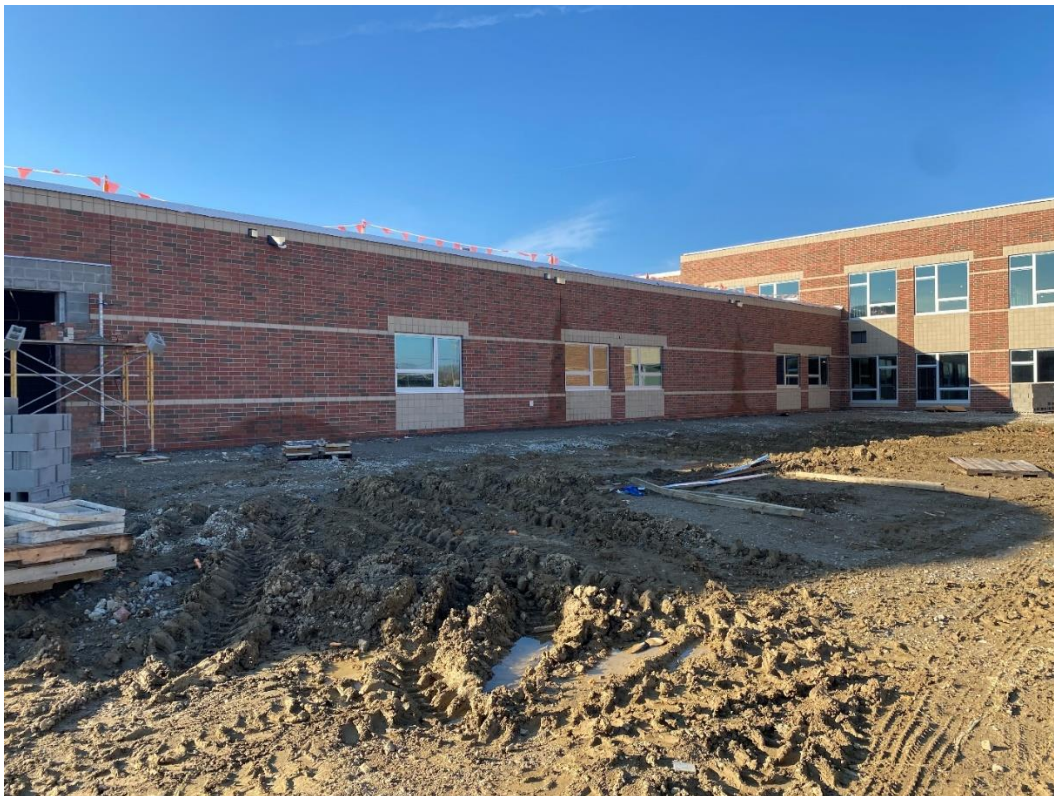
Windows are installed on the east side of Classroom Area B.
