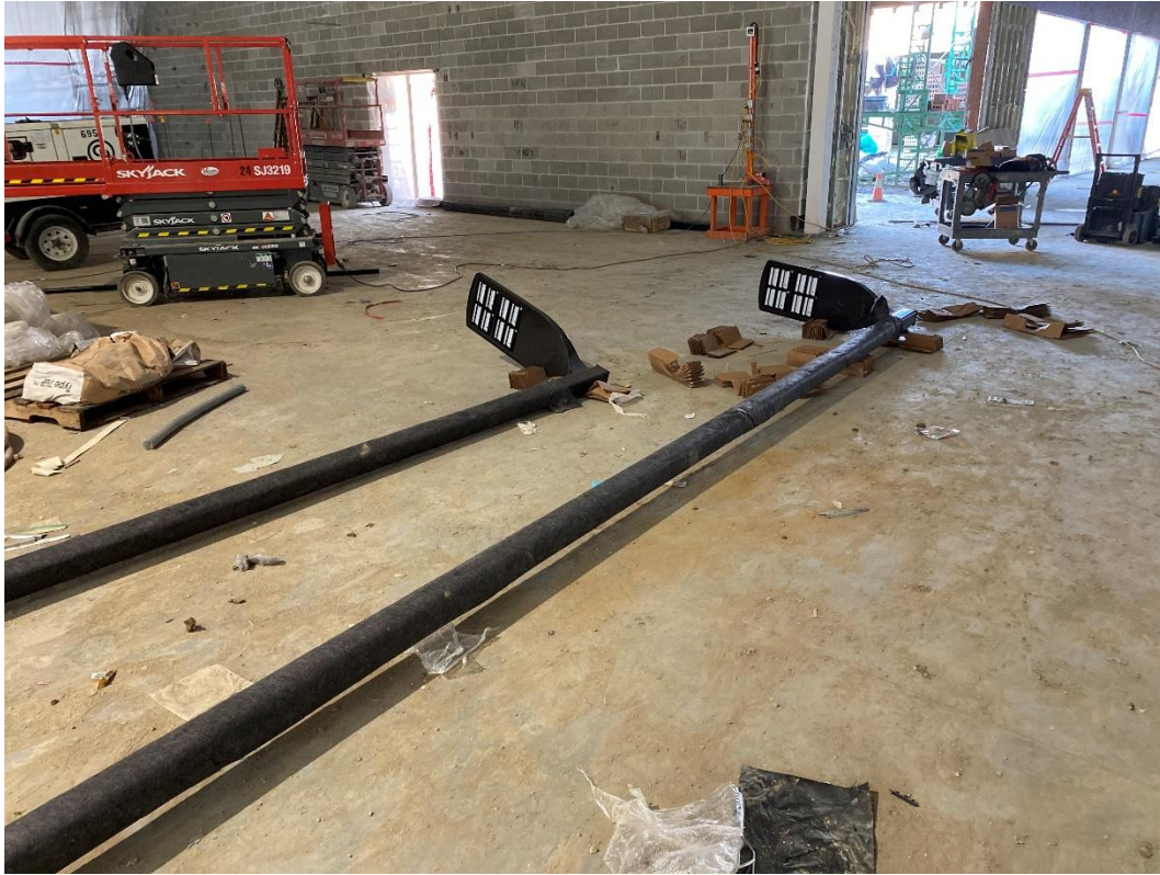
LED site lighting poles and fixtures are readied for installation.
