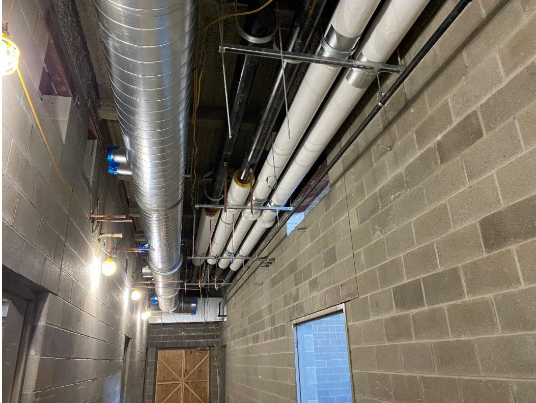
Pipe insulation work is progressing in the Locker Room corridor.
