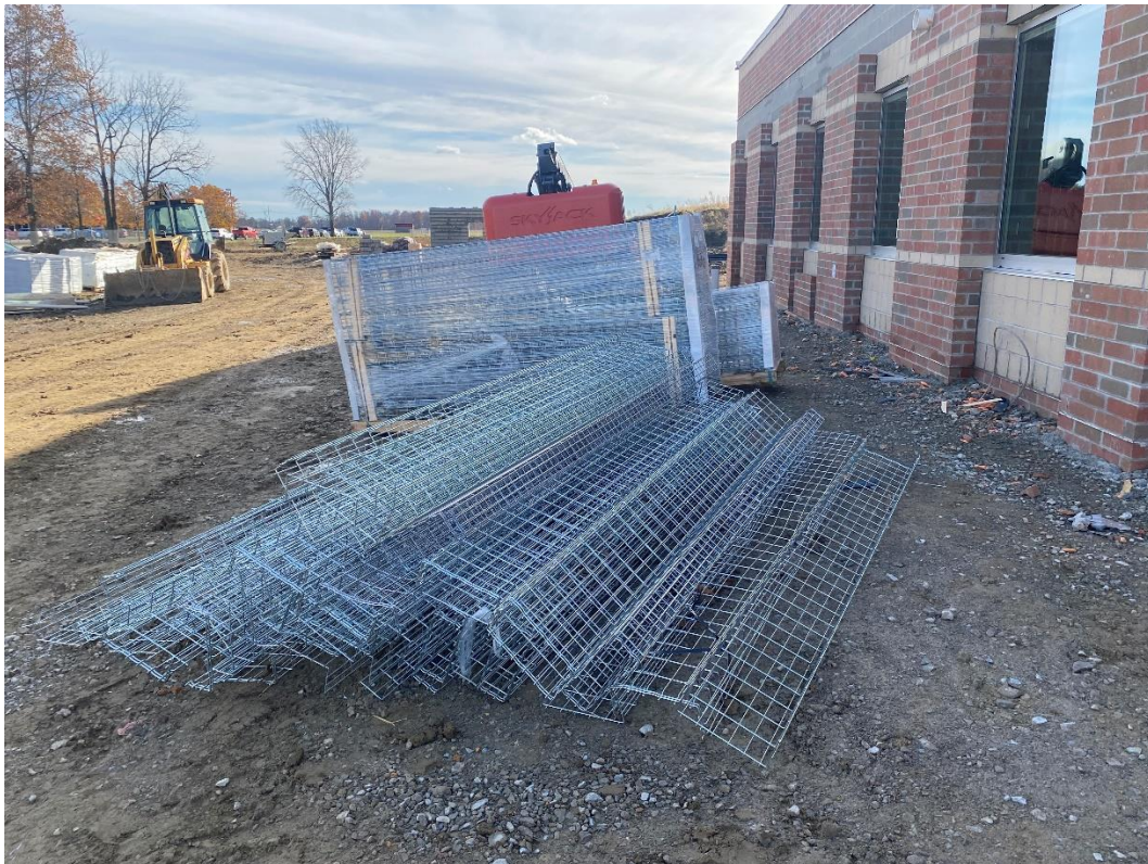
Delivery of cable trays for data wiring have been received.
