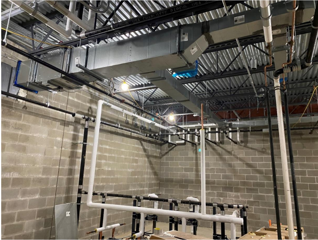
Installation of exhaust ductwork is nearly complete at the main toilet rooms, first-floor, Area C.
