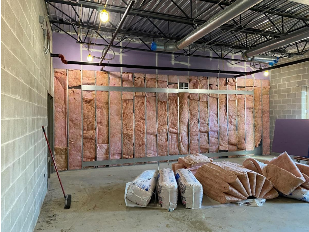
Installation of acoustical wall insulation is progressing at the second-floor level of Area C.
