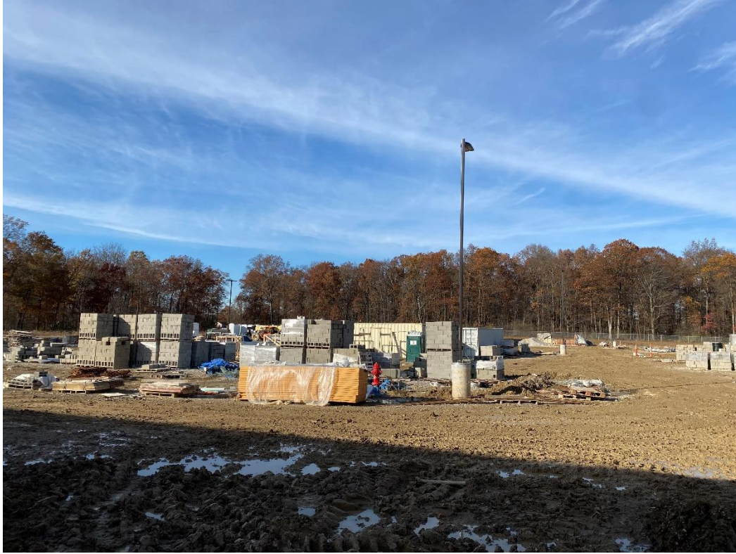
Light poles are installed in the north lot.
