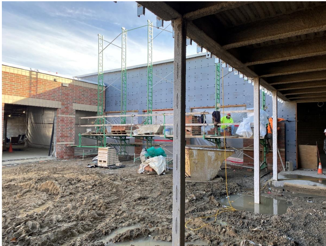
Brick veneer installation on the north wall of the Student Dining area is progressing.
