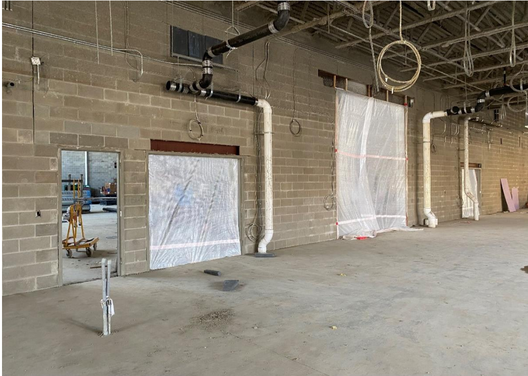
Installation of air barriers will isolate Area F. Temporary heat in this area will allow installation of spray-on fireproofing to continue.
