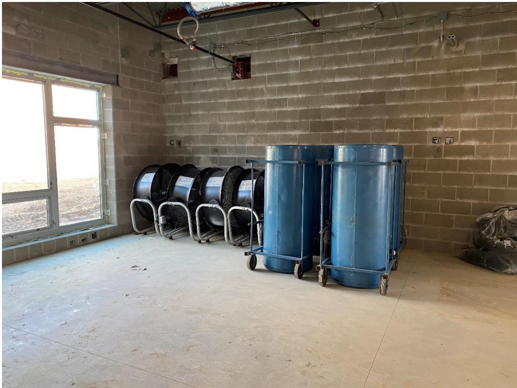
Temporary heating units and fans ready for installation.
