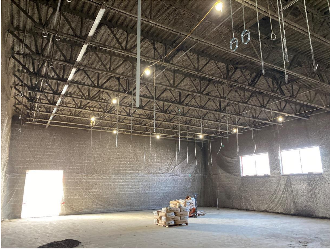
Spray-on fireproofing in the music classrooms is 50% complete.
