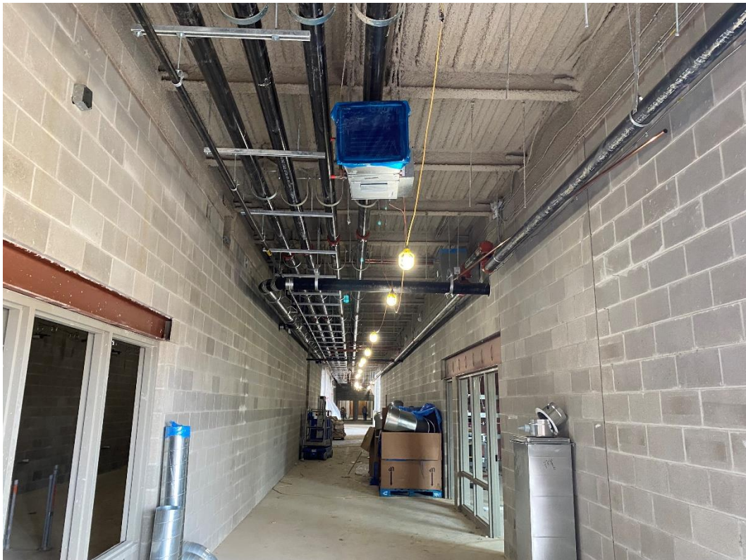
Installation of VAV boxes in the main corridor east of the Gym has begun.
