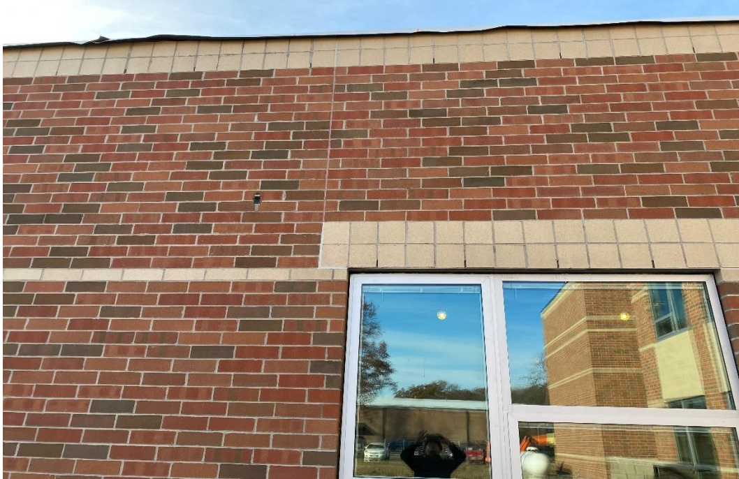
Installation of sealants at masonry control joint is progressing after the brick is cleaned.
