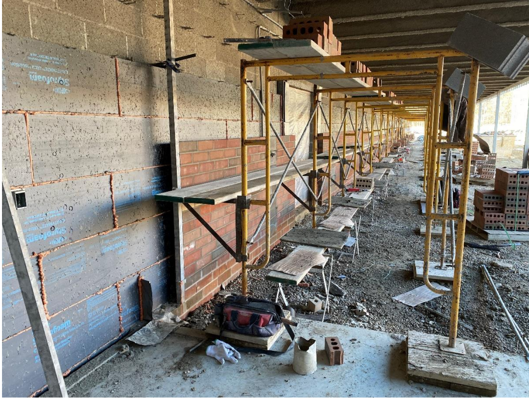
Brick veneer at the north entry canopy is 50% complete.
