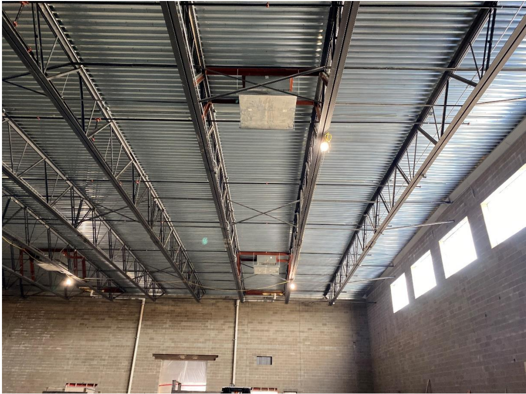
Installation of roof ventilators in the Gym.
