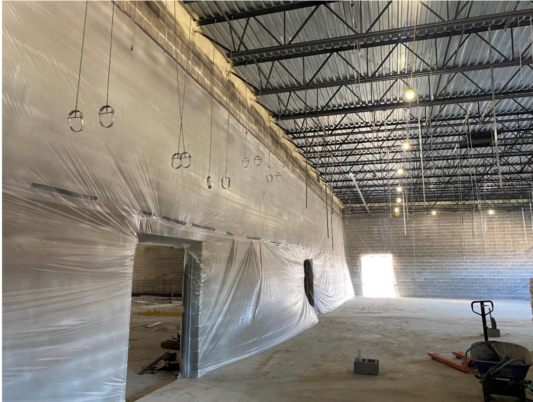
Walls are draped for installation of spray-on fireproofing in the Music Classrooms.
