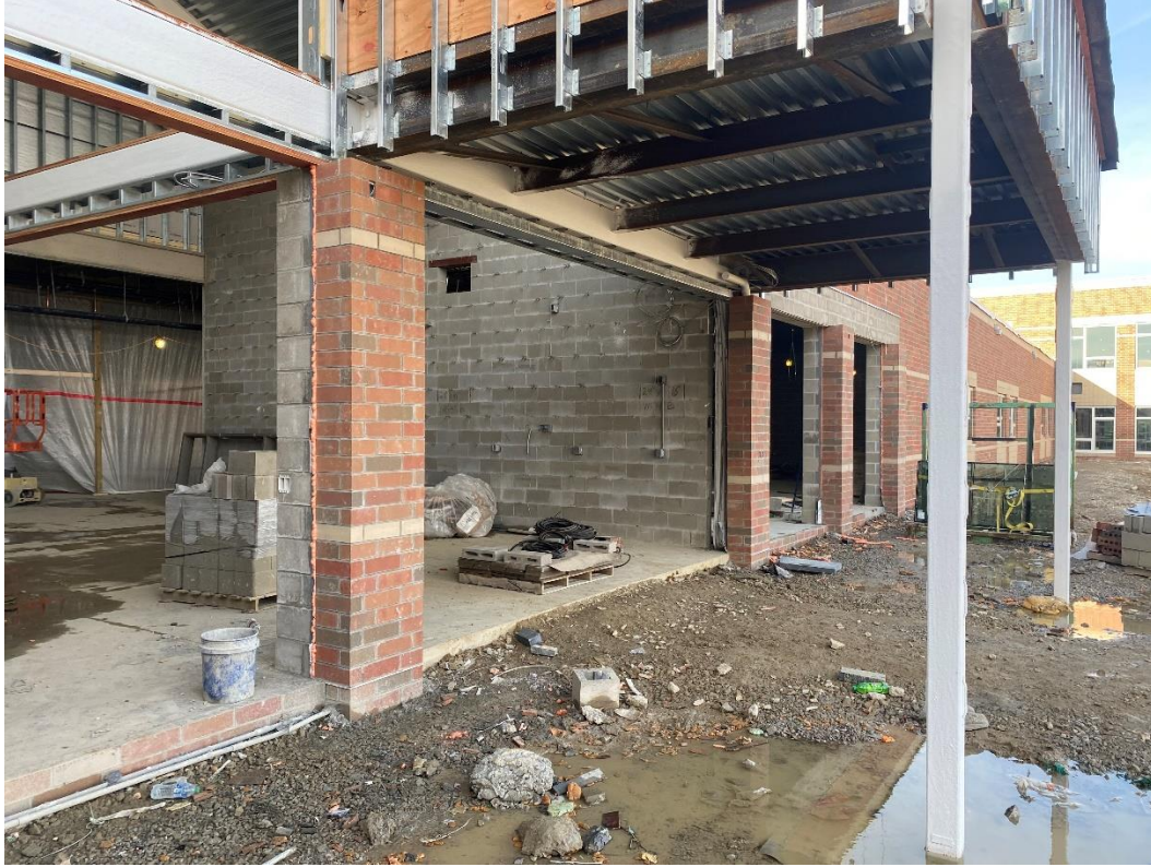
Brick veneer work is progressing at the main entry.
