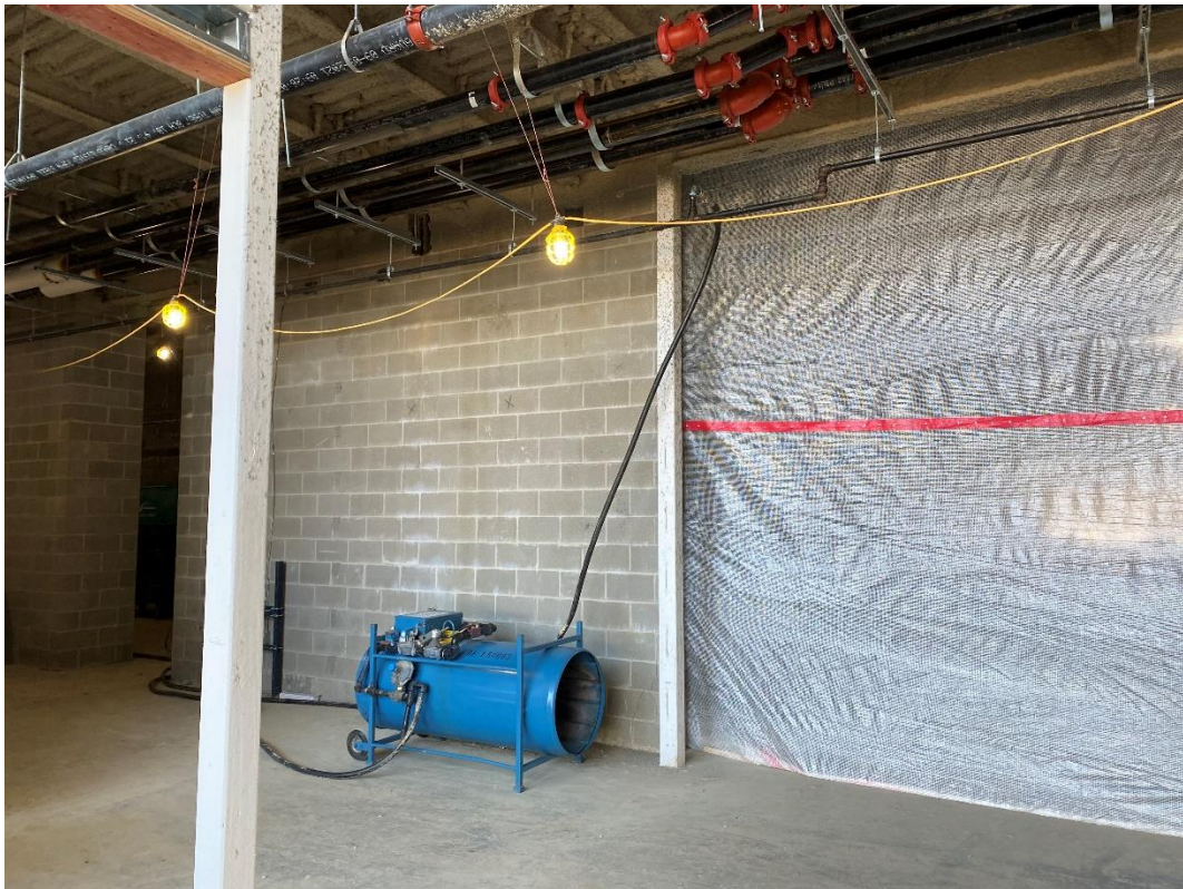
Temporary heaters are being connected to the gas piping system throughout the building.
