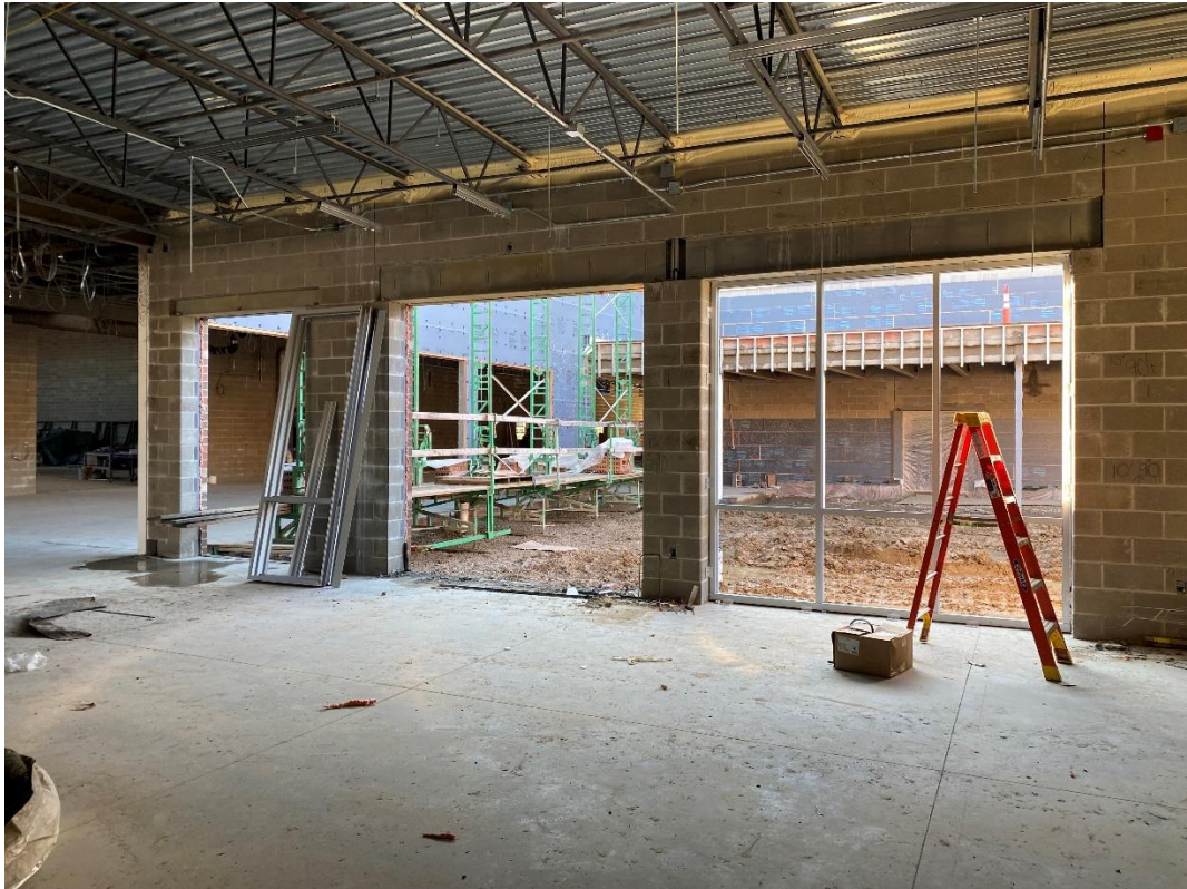
View looking west into the north entry courtyard from the Engineering Lab.
