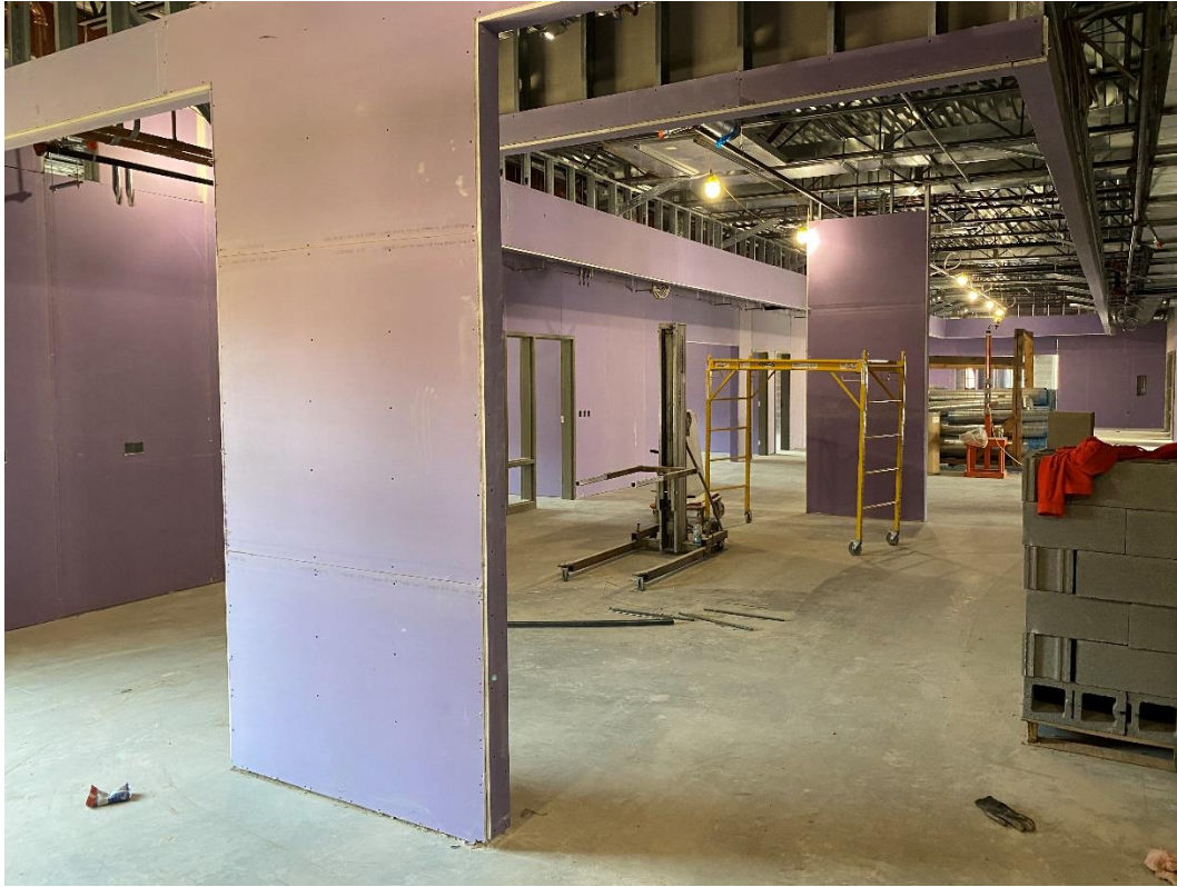
Impact resistant drywall is completed at the second-floor level of Classroom Area D.
