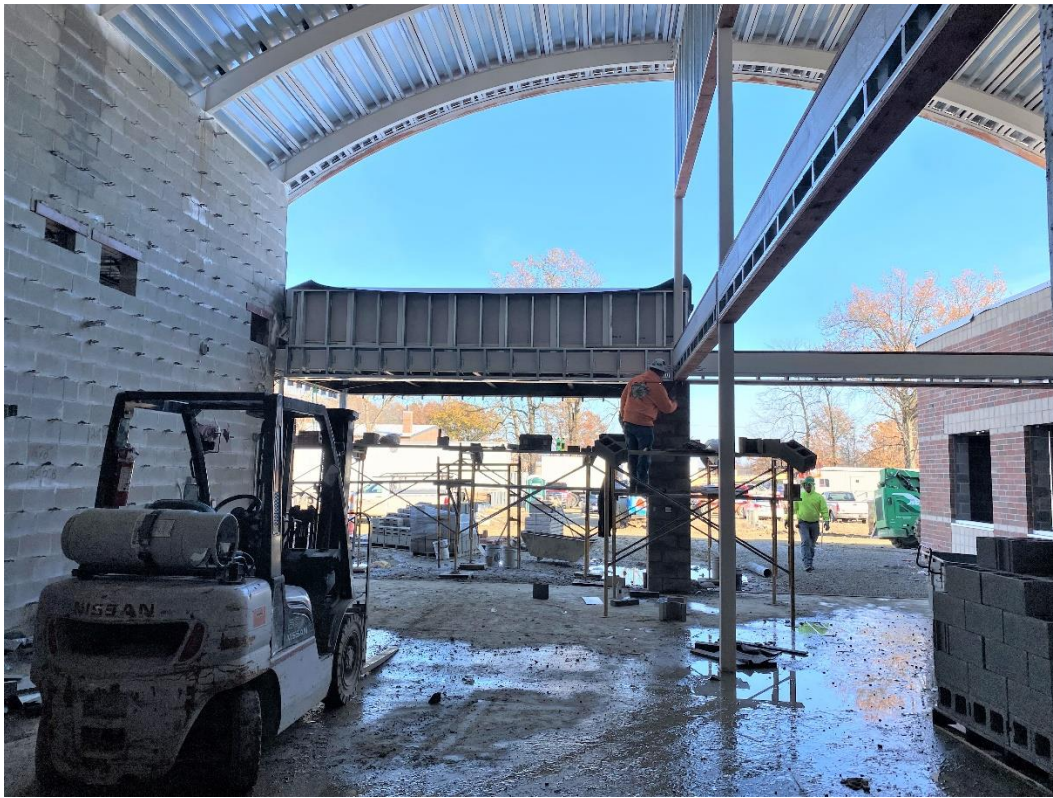
Brick masonry work is progressing at the main east entry.
