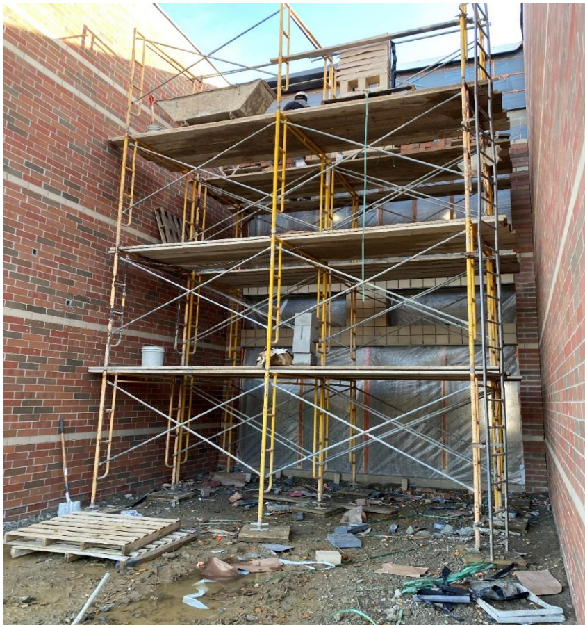
Brick veneer is being completed at the north exit of Area D.
