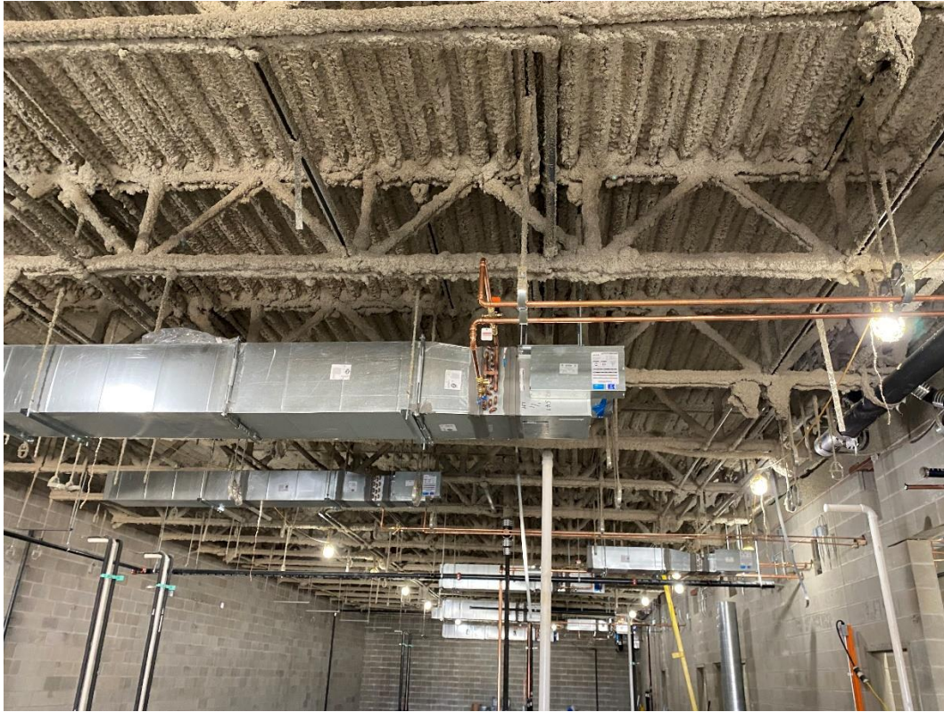
Installation of copper supply and return piping to the VAV boxes in the locker rooms is progressing.
