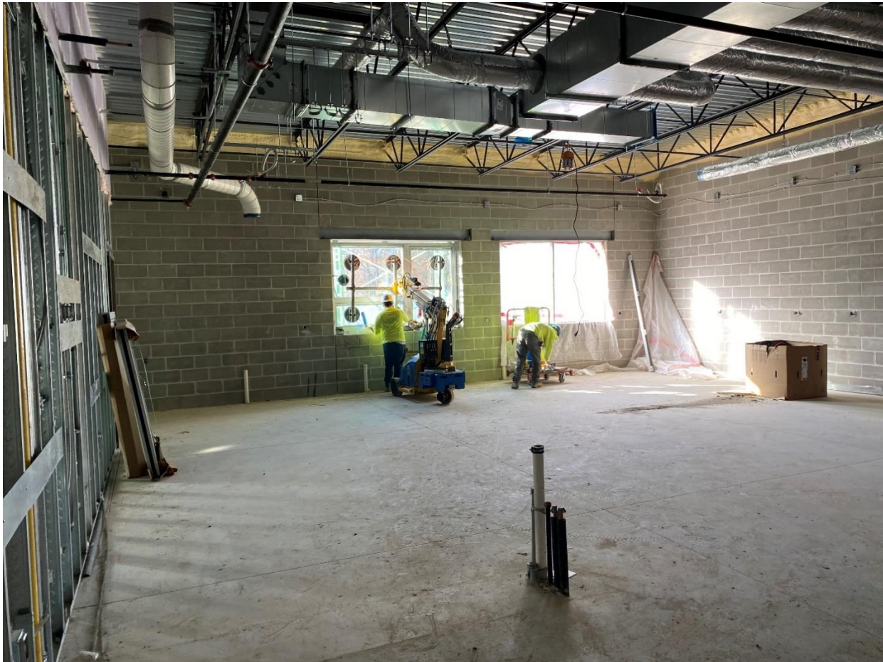
Installation of windows continues in Area D, Science Rooms.
