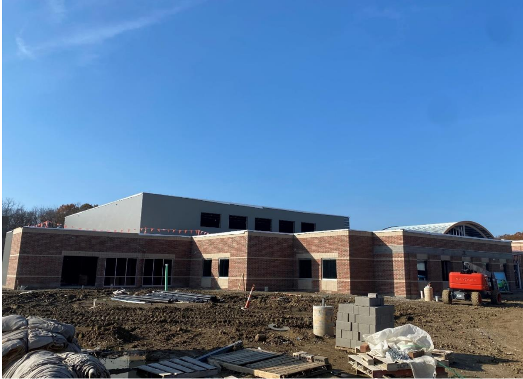
Metal wall panels are 95$ installed on the upper east side of the Gym.
