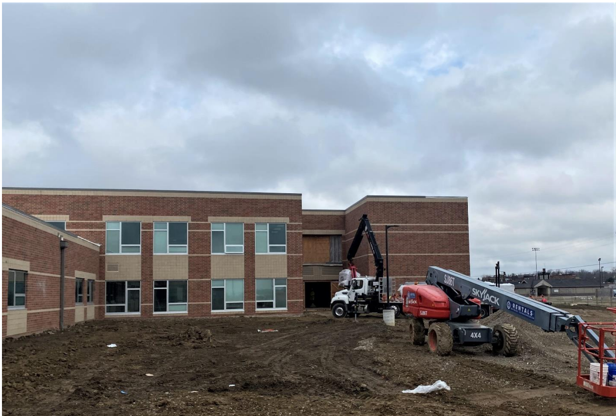
Delivery of carpet tiles to classroom Areas C & D.
