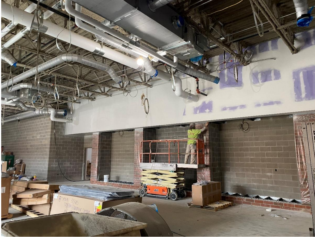
Drywall finishing continues in Area E Student Dining.
