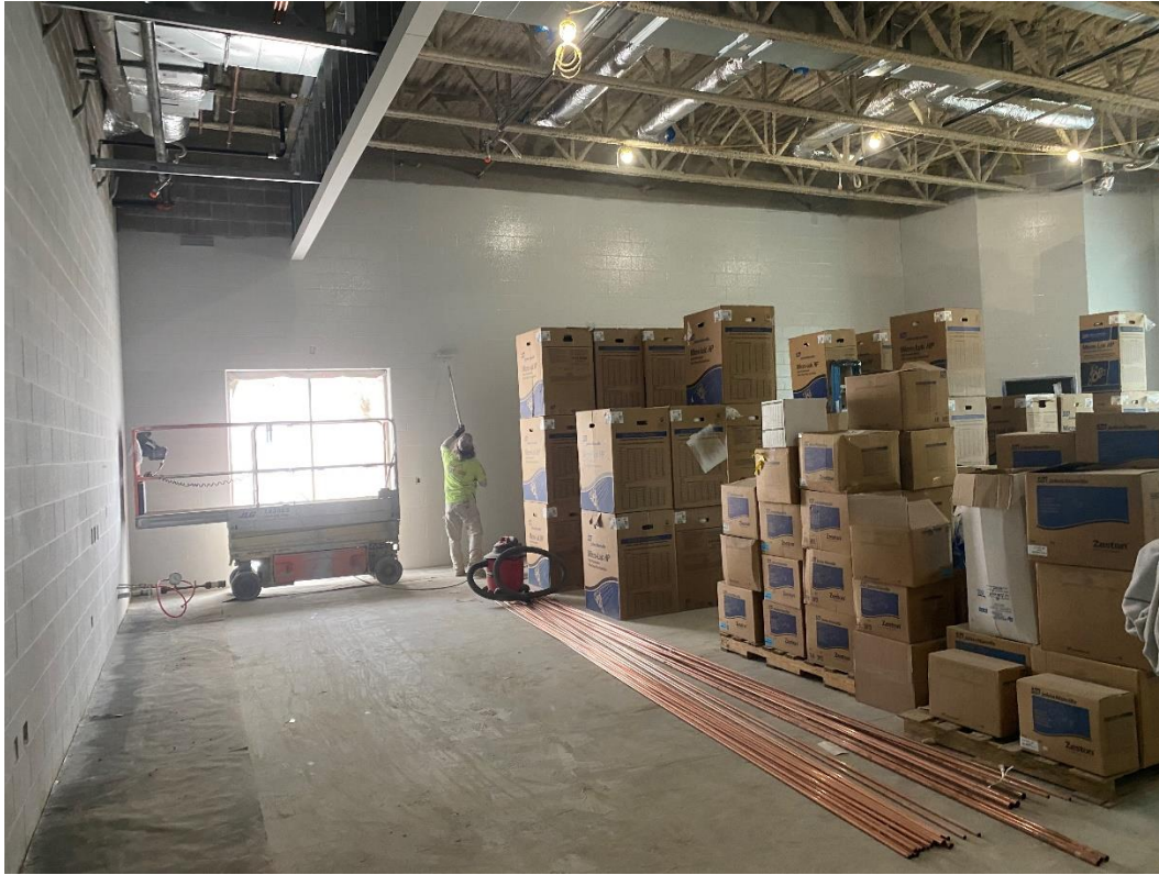
Painting is being completed in the Instrumental Music classroom.
