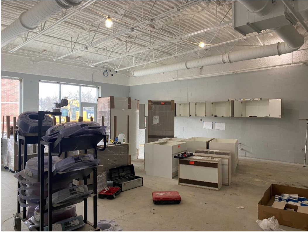
Cabinetry is installed in Art classrooms.
