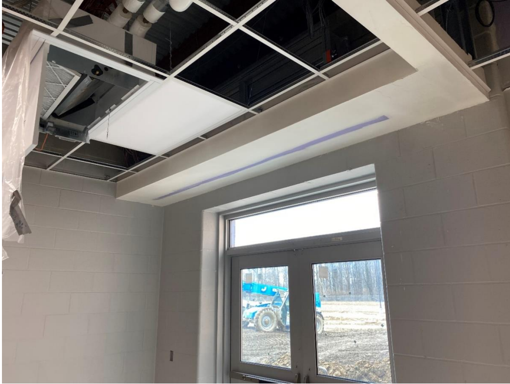
Drywall bulkhead is installed at the north exit, Area D.
