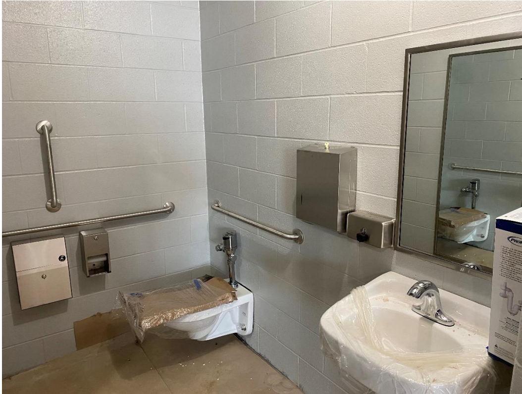
Toilet accessories are installed in Area C & D second-floor toilets.
