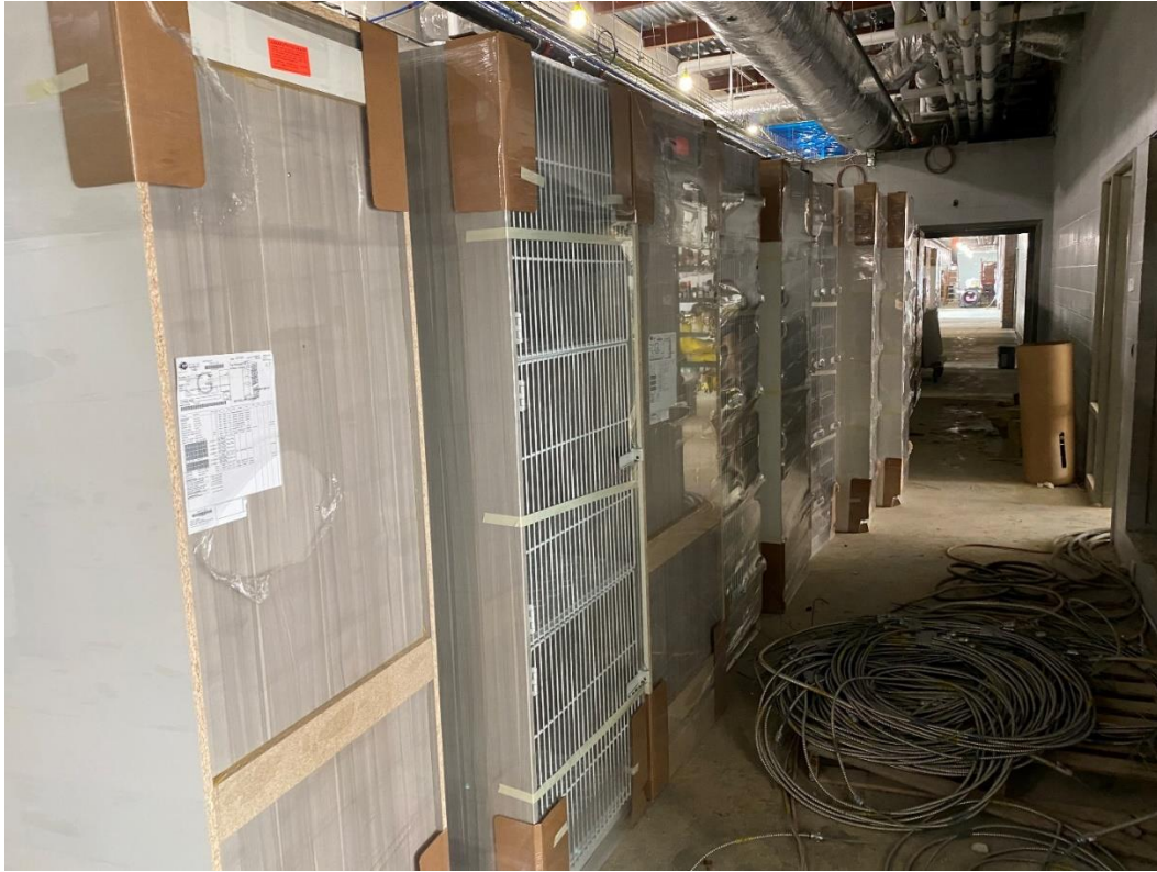
Art classroom project storage cabinetry has arrived.
