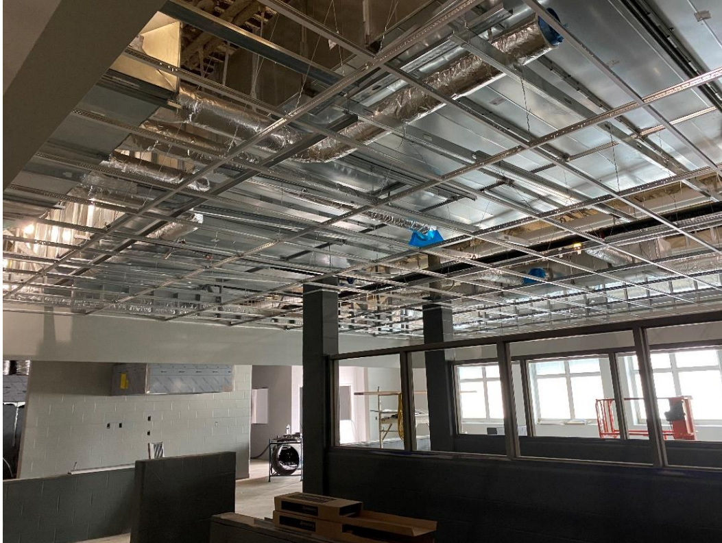
Ceiling grid is installed in the Kitchen.
