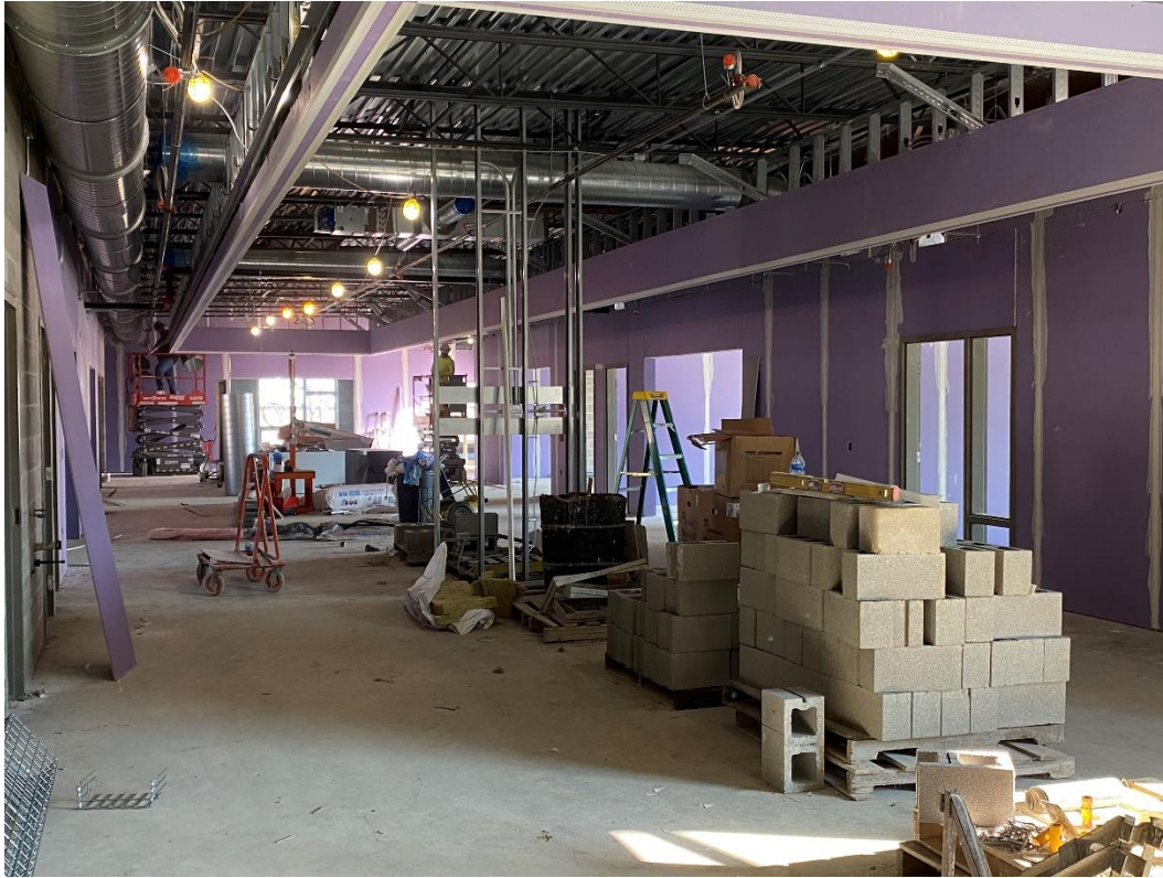
Drywall taping and finishing has started at the second-floor level of Area C.
