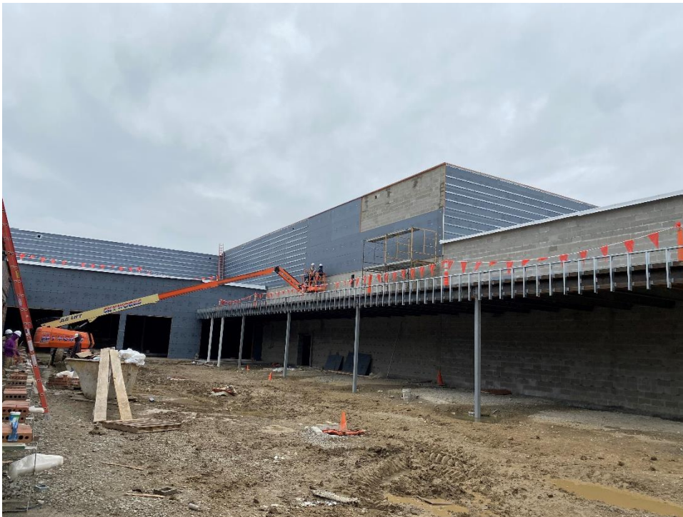
The air barrier and 'Z' furring for metal siding is nearly complete at the upper walls of the performing arts center. Siding installation will start next week.
