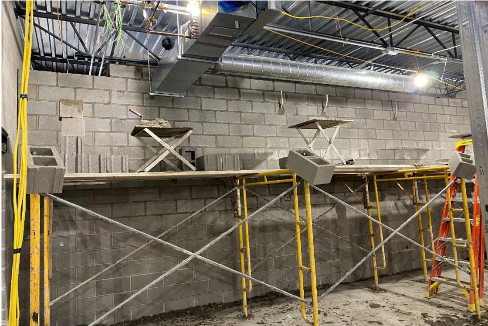
Interior masonry work continues in Areas C & D.
