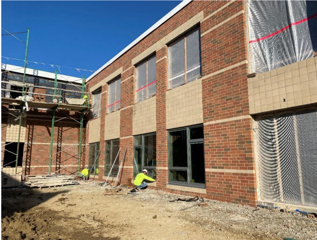
Window installation on the first-floor level of Area D is nearly complete. Work will move to the second-floor level.
