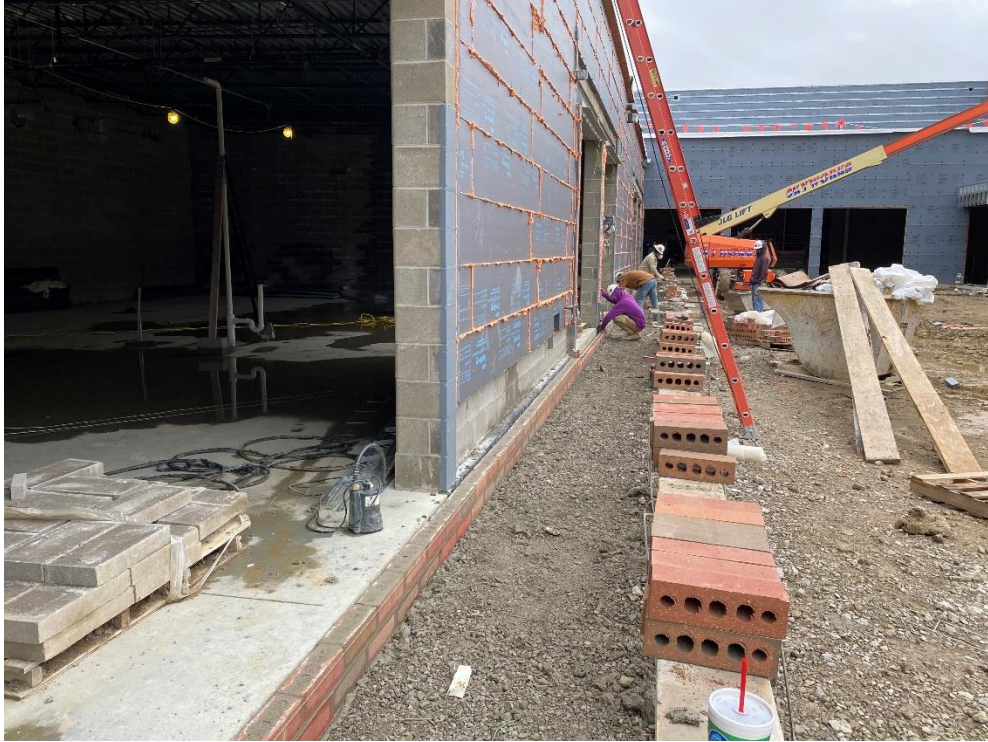
Installation of brick base flashing should also be complete today.
