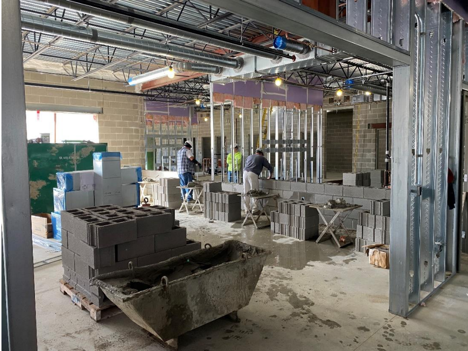
Interior masonry walls are progressing at the small toilet rooms at the second-floor level of Area D.
