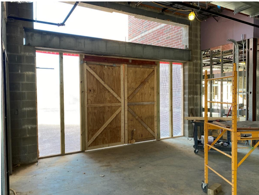
Temporary doors installed at the first-floor, Area C.
