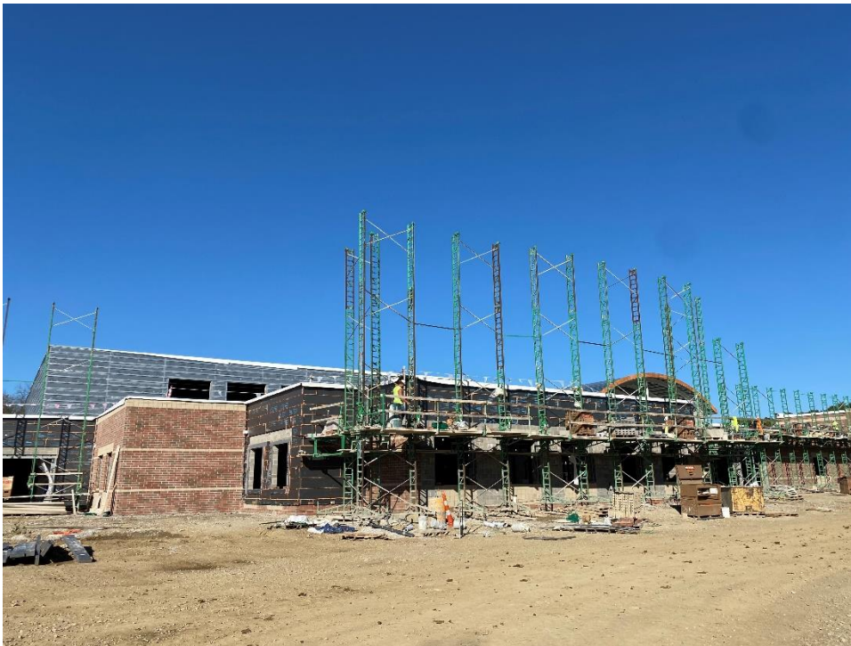
Brickwork is 50% complete on the east front walls of Area A.
