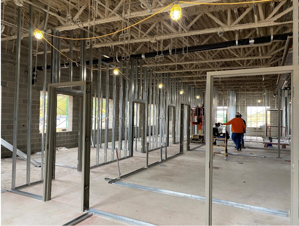
Light gauge metal framing in the Administrative Offices is 60% complete.
