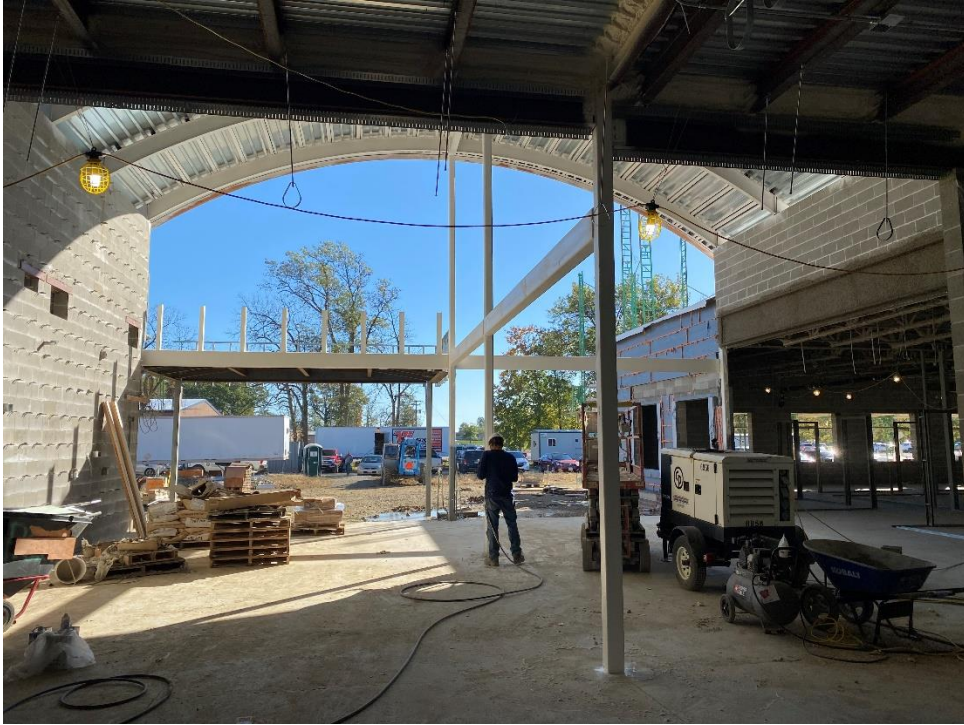
Installation of intumescent paint on structural steel framing at the main entry.
