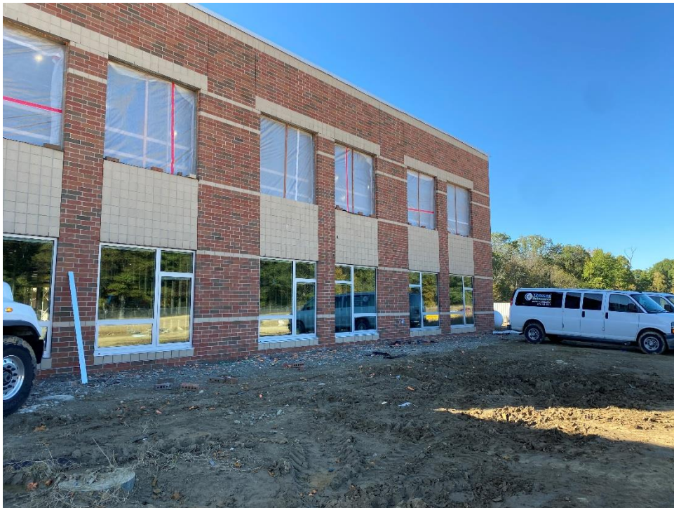
Window installation is complete at the first-floor level and north side of Area D.
