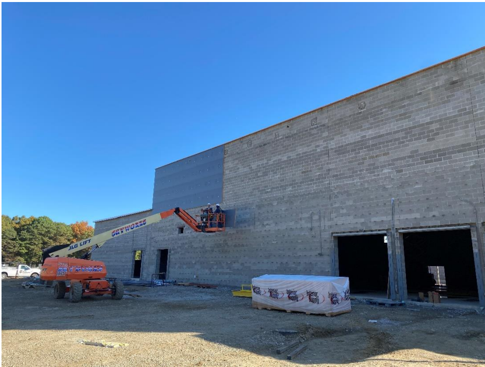
Installation of the air barrier continues on the west side of the performing arts area. Installation of metal wall panels will start next week.
