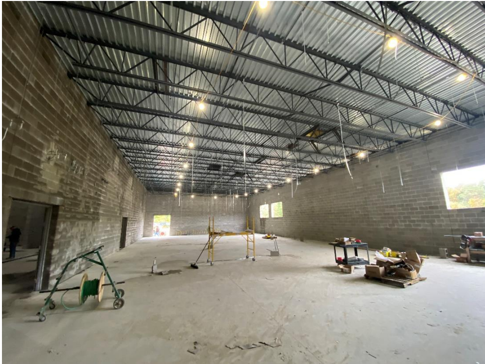
Pipe hangers are being installed in the Area E Music classrooms.
