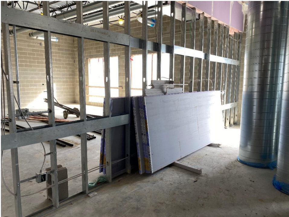
Drywall has been delivered and is stockpiled on the second floor of Area D. Installation will begin once all the windows are installed.
