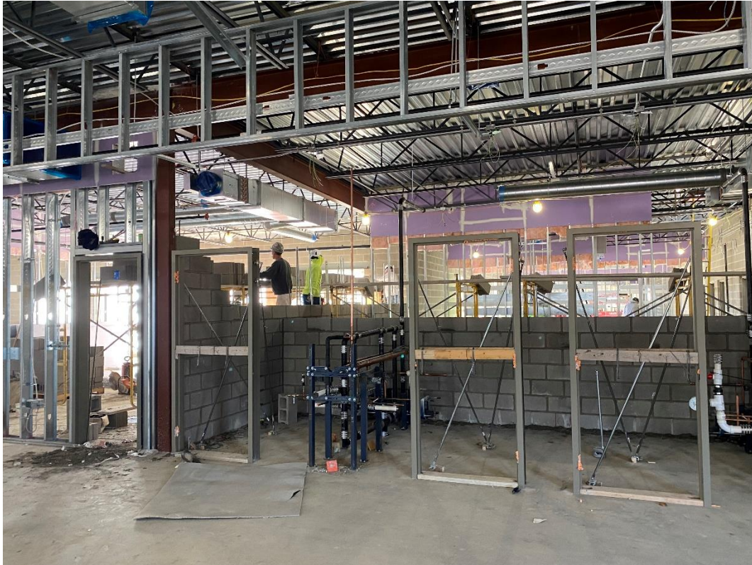
Door frames installed and interior masonry walls progressing at the Area D second-floor toilet rooms.
