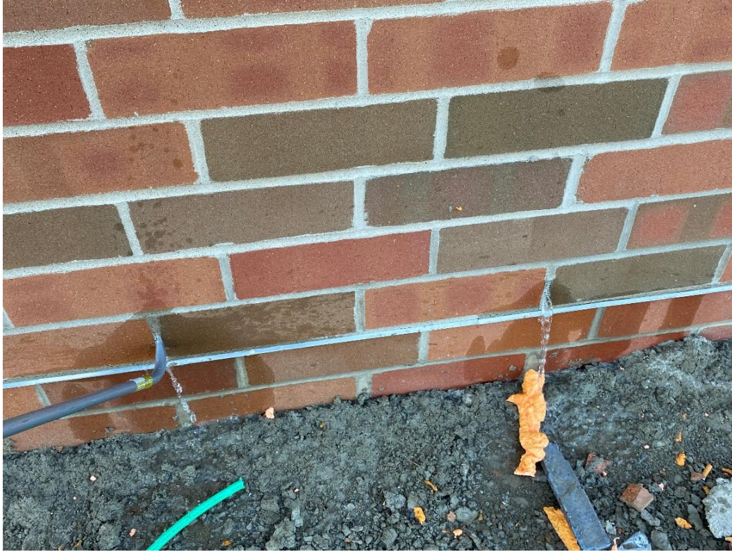
Water is free-flowing from the weep vents.
