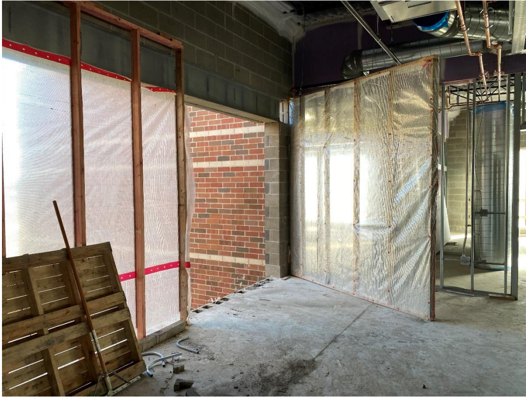
Installation of temporary weather barriers at the second-floor of Area D.
