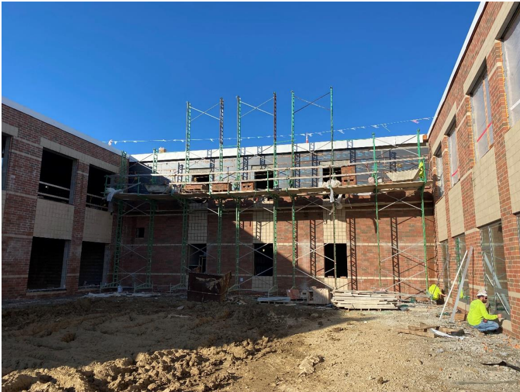
Brickwork on the interior east wall of Area D should finish this week, pending weather.
