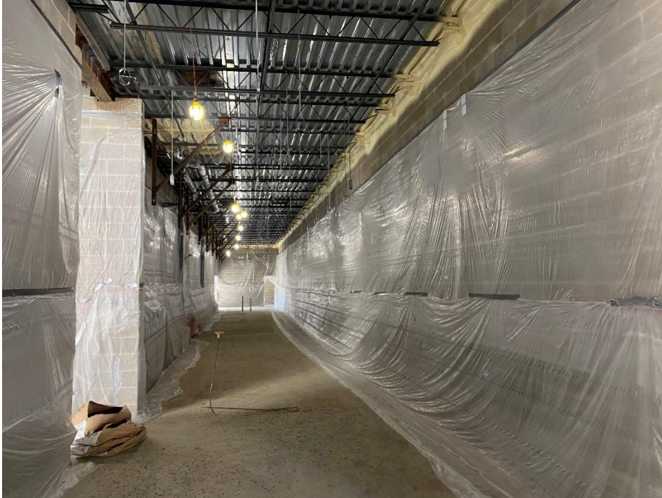
The main corridor west of the administrative offices is draped for installation of spray on fire proofing.
