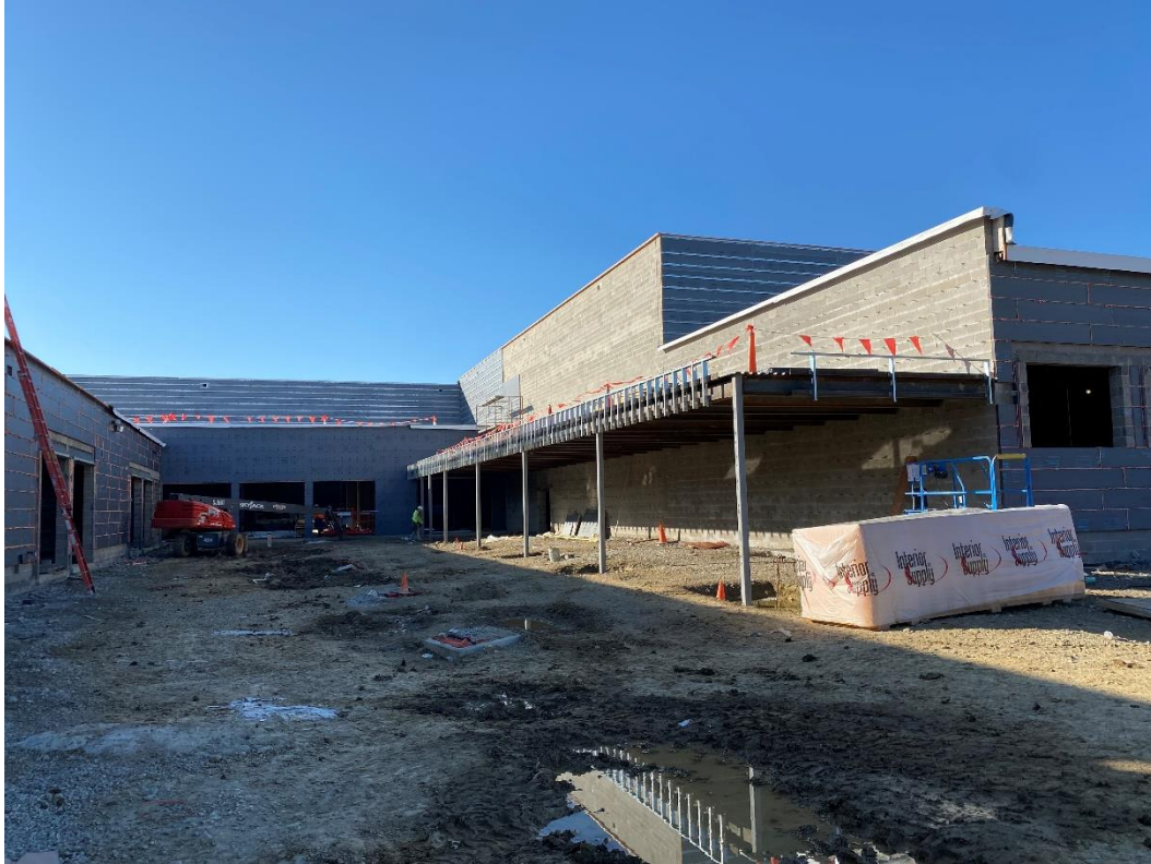
The air barrier installation continues on the east wall of the performing arts, Area F.
