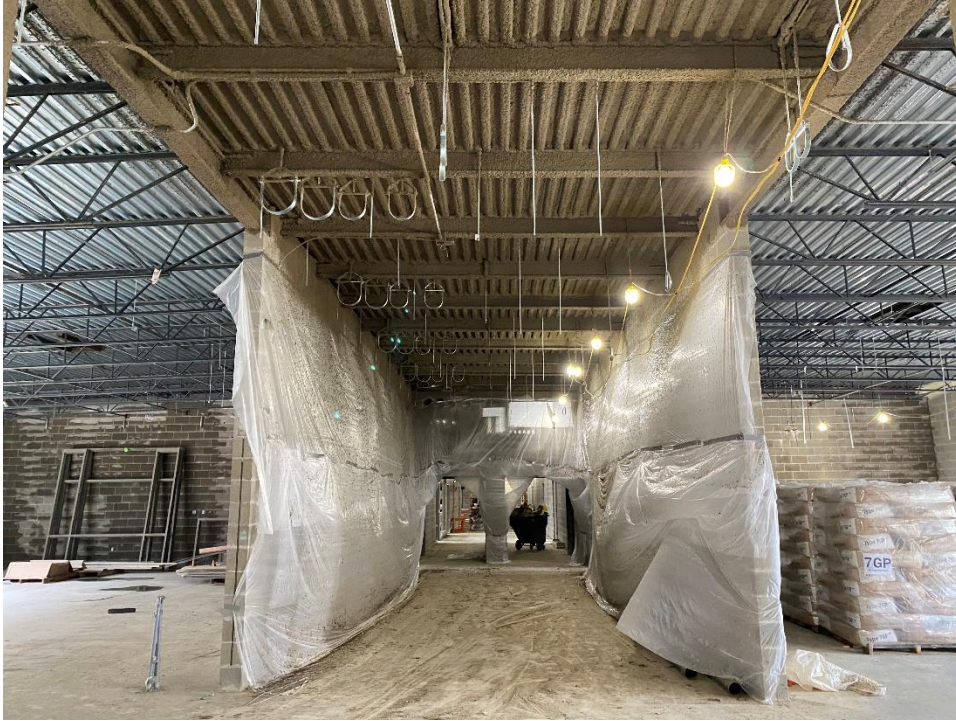
Fireproofing in the main corridor to the fire wall at Area B is complete. View looking north.
