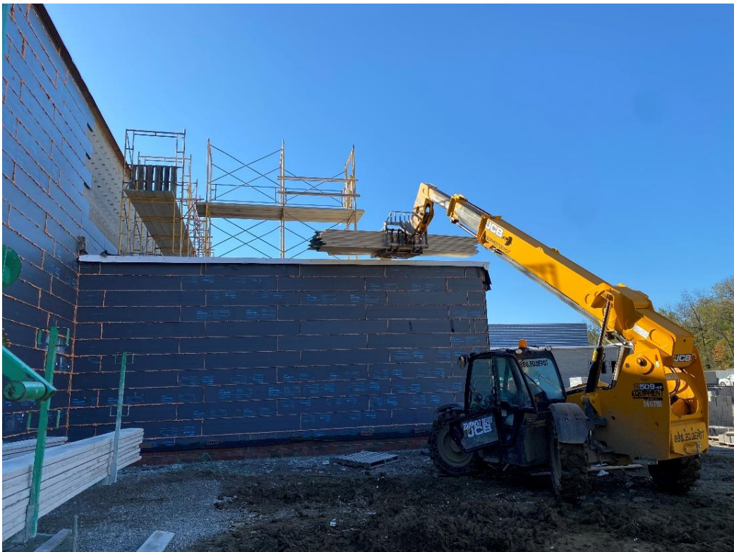
Scaffolding is erected for brick installation on the west wall of Area D above the Science rooms.
