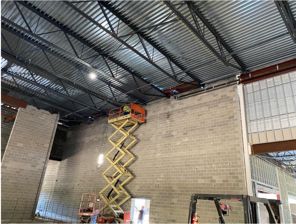
Installation of roof drains and storm drainage piping in the performin arts center.
