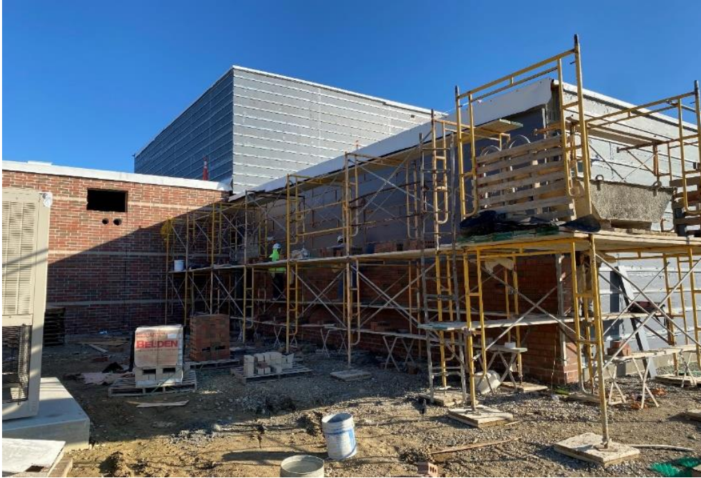
Brick veneer on the west side of the Area E Locker rooms will finish this week.
