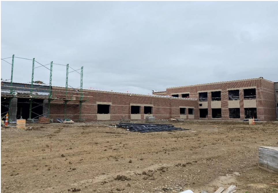
Brickwork is complete and scaffolding is removed at Area B.
