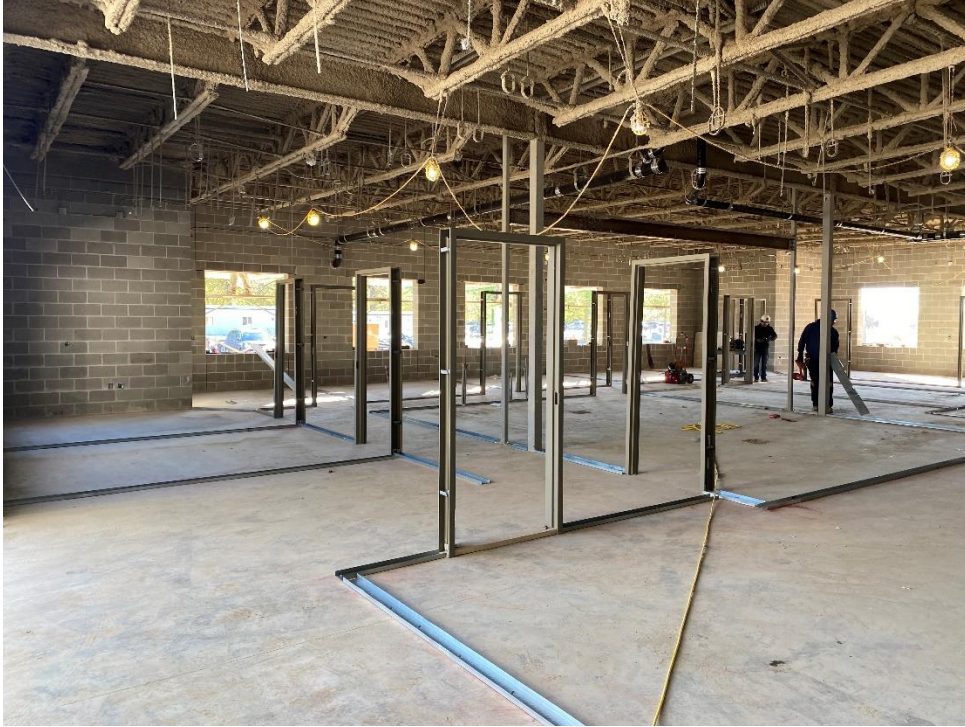
Installation of metal track for the light gauge metal wall framing and HM door frames has started in the Administrative Offices.
