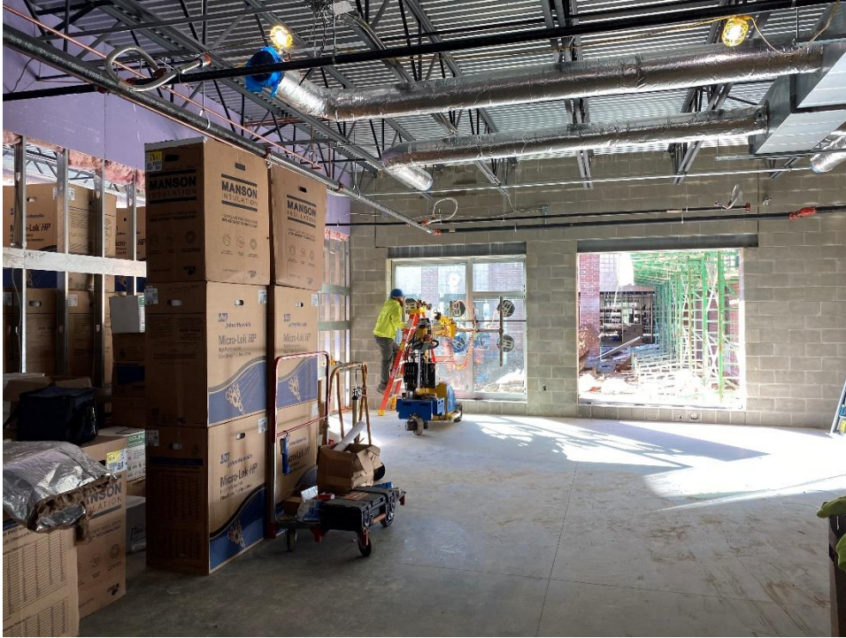
Installation of windows on the south side of Area D.
