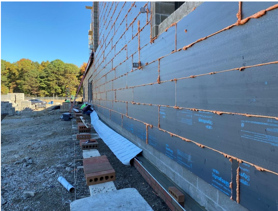
Installation of masonry base flashing on the west wall of Areas C & D.
