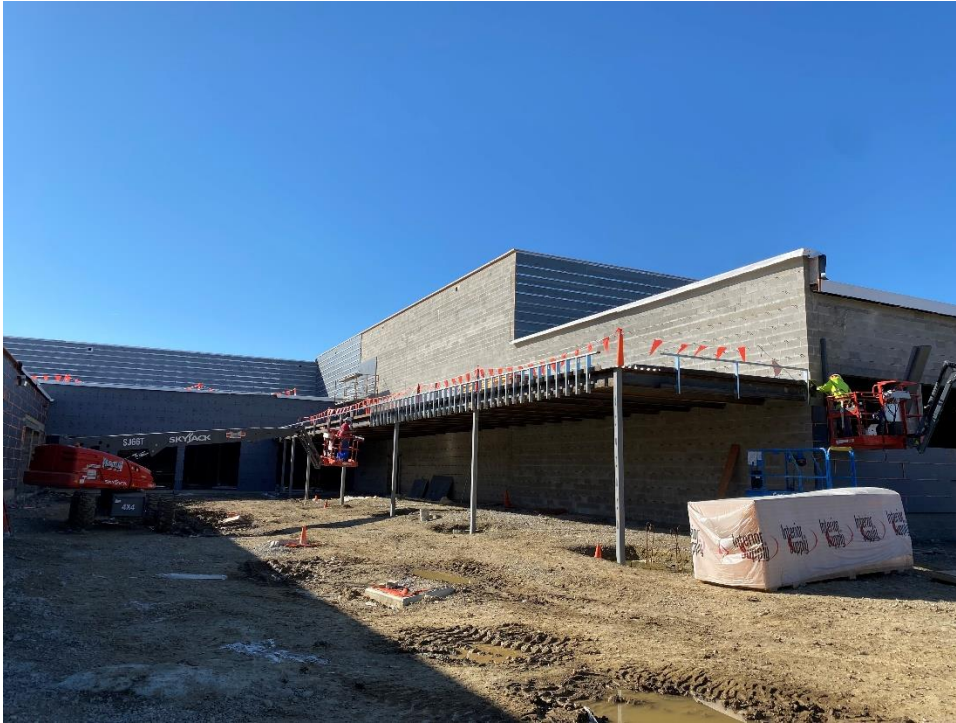
Light gauge metal framing is nearly complete on the parapet wall of the north entry canopy.
