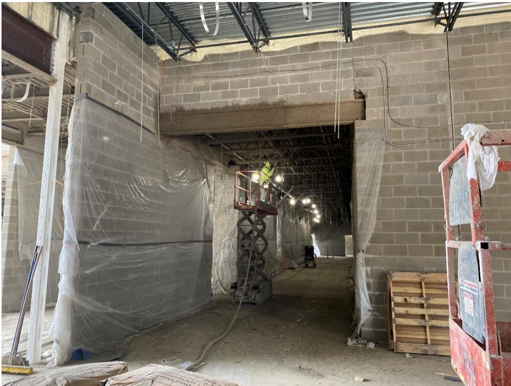
Fireproofing in the main toilet rooms west of the administrative offices is nearly complete.
