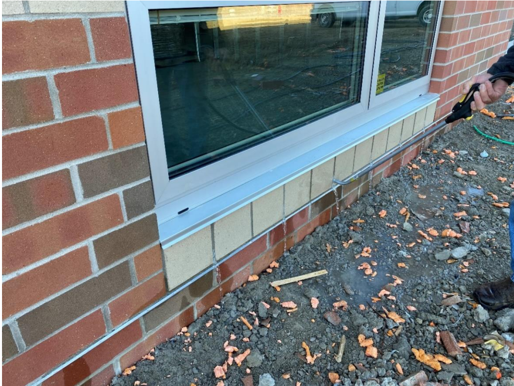
Base flashing and weeps are water tested on Area D.
