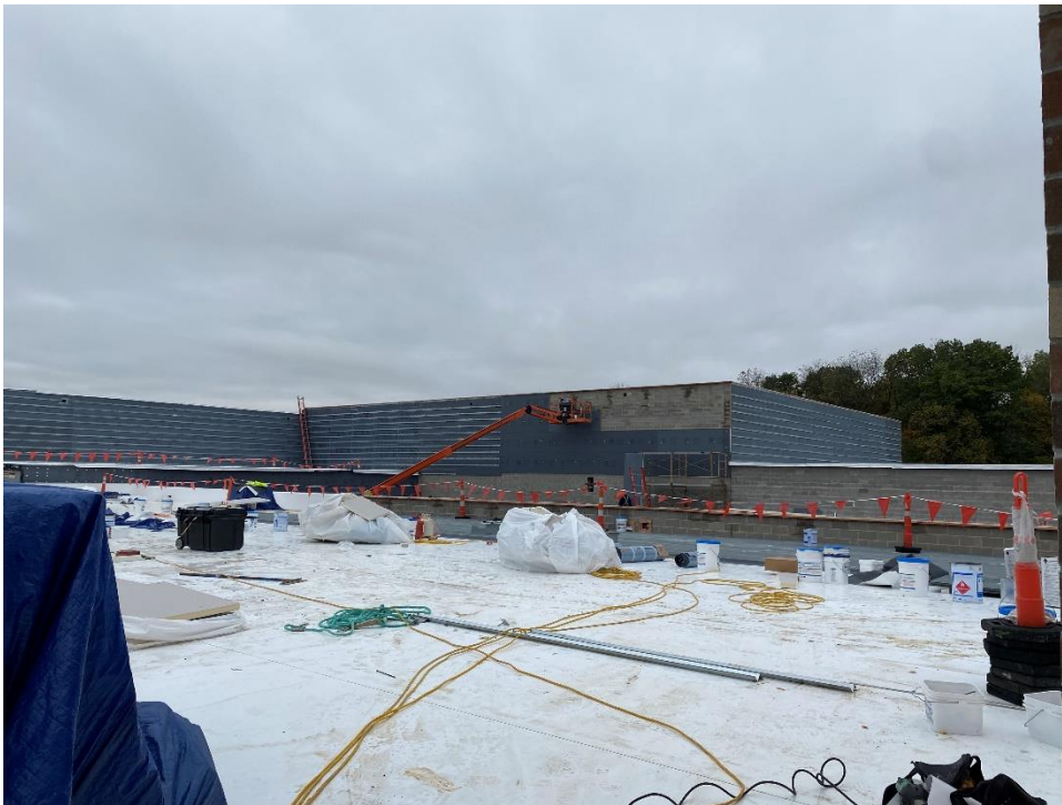
Single story Areas C & B roofing is 80% complete.
