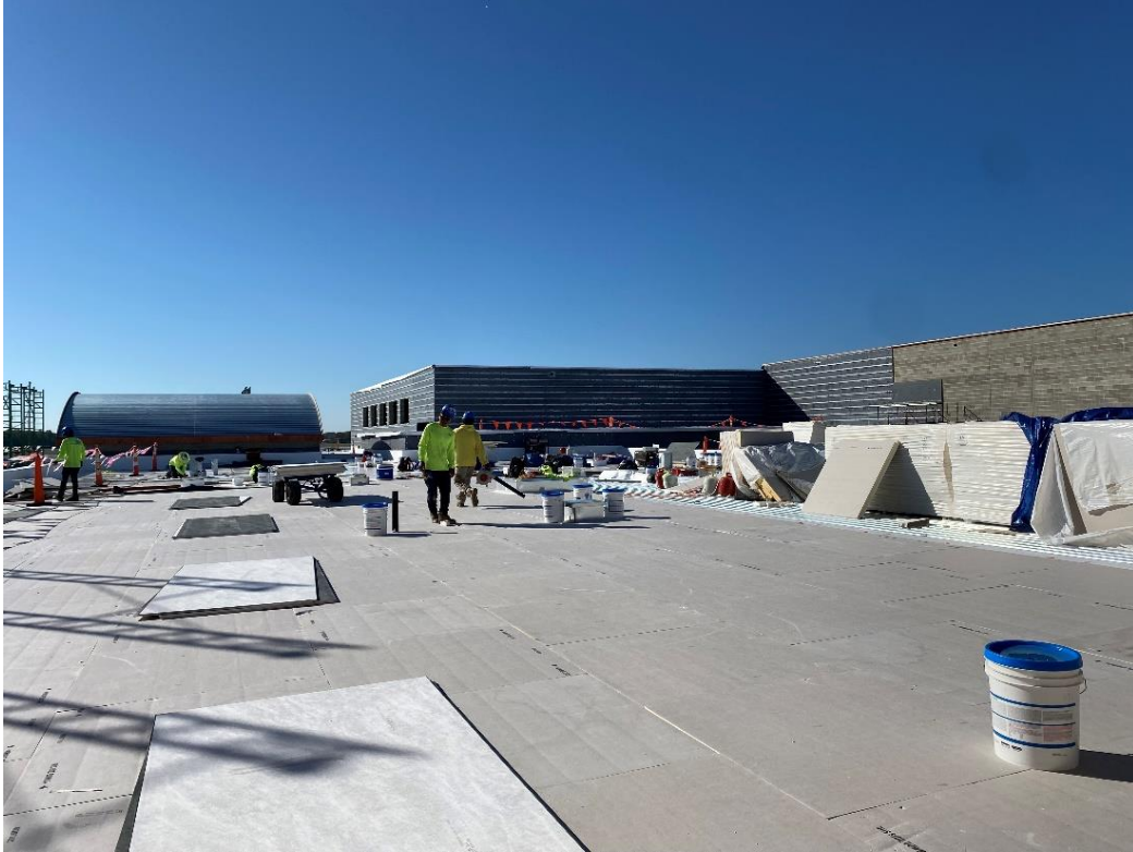
Roofing work is progressing on Area B and should finish here next week.
