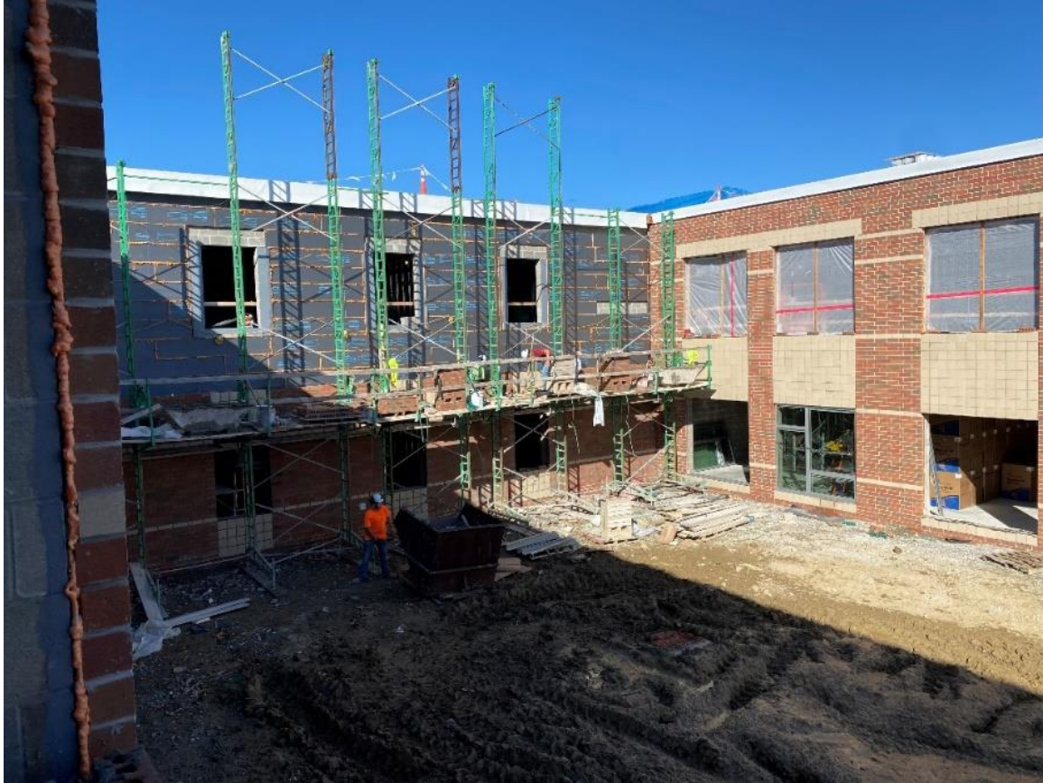
Brickwork is 50% complete on the east joining wall between Area C & D.
