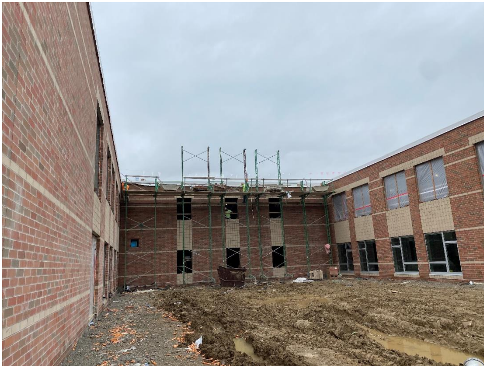
Brickwork on the east interior wall between Areas C & D should finish today.
