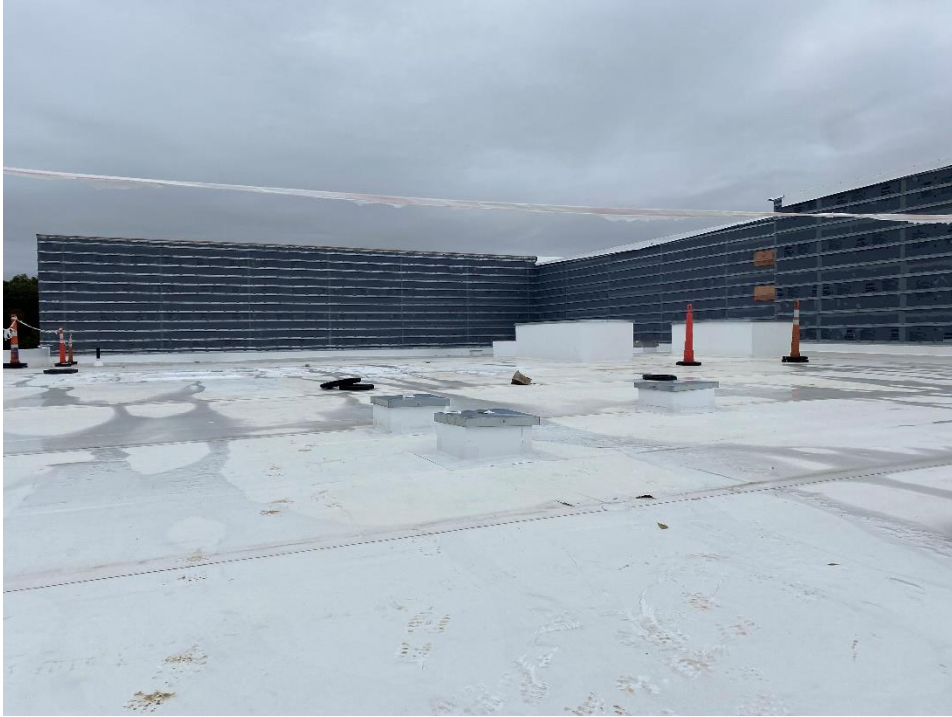
Base flashings for mechanical equipment curbs is complete above the main Area E Mechanical Room.
