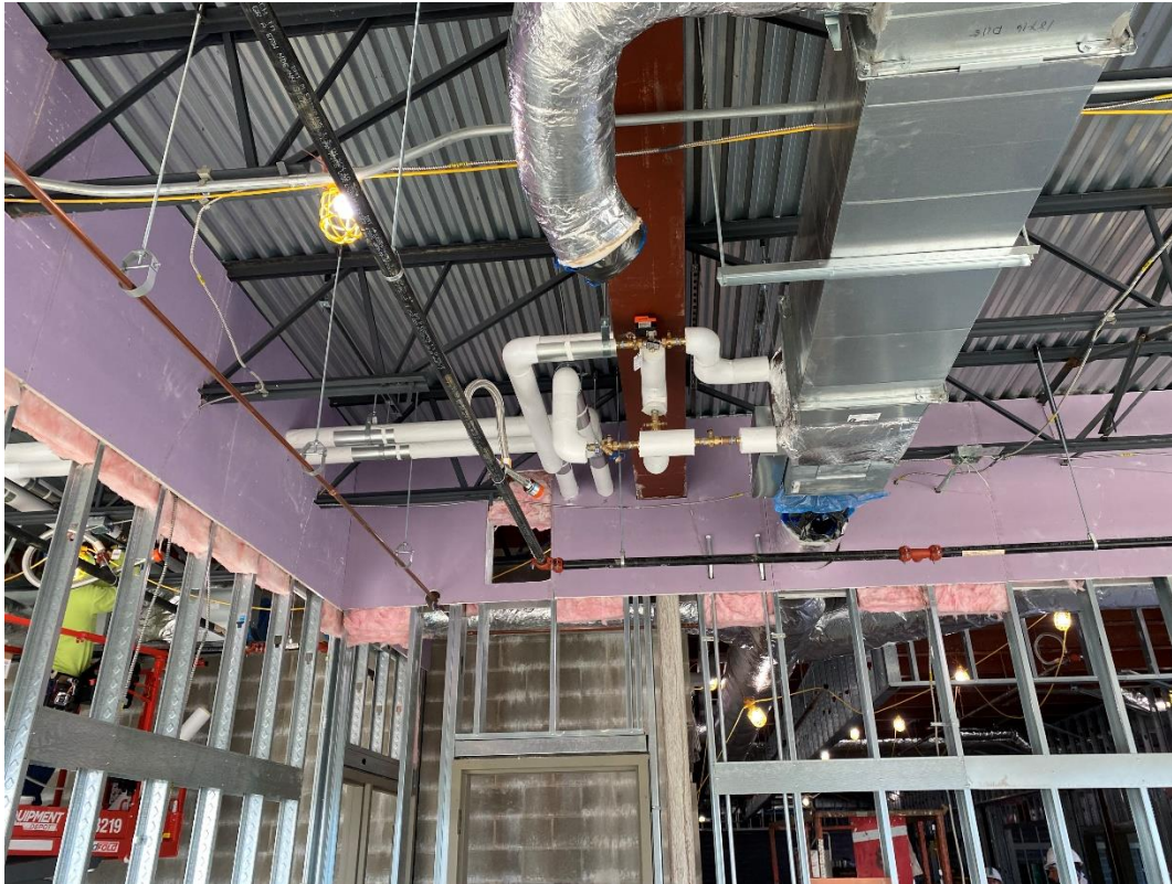
Pipe insulation work continues in area C & D.
