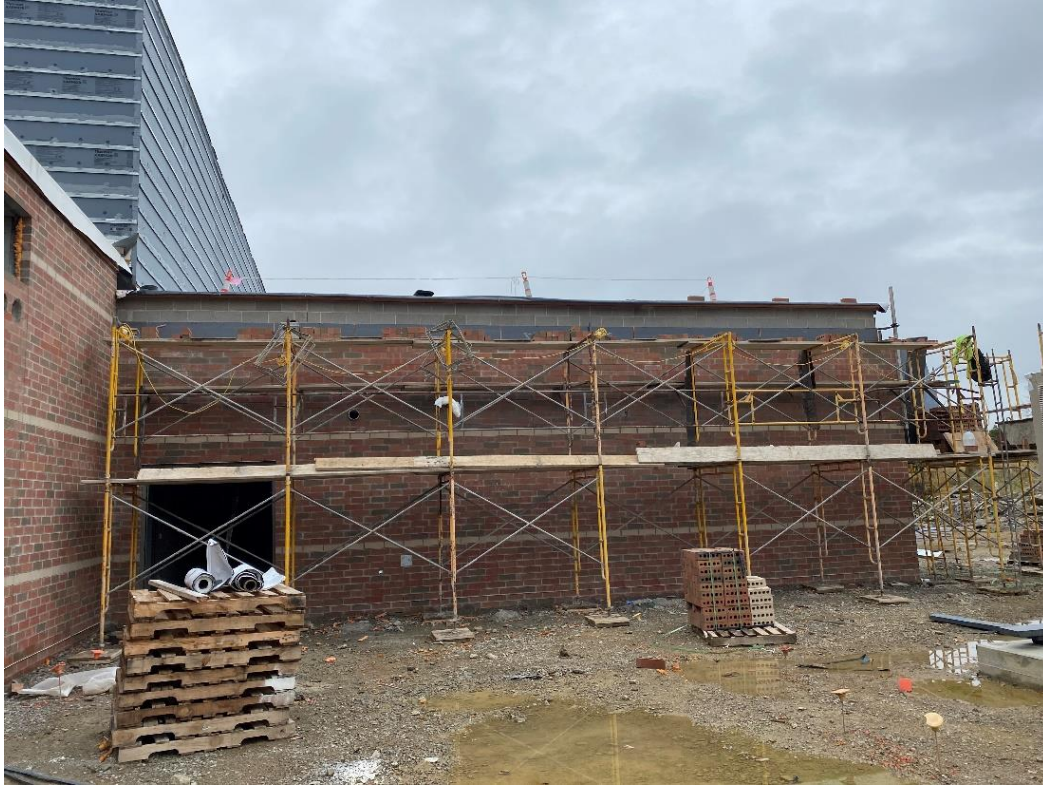
Brick veneer should finish on the west side of the Locker rooms, Area E, today.
