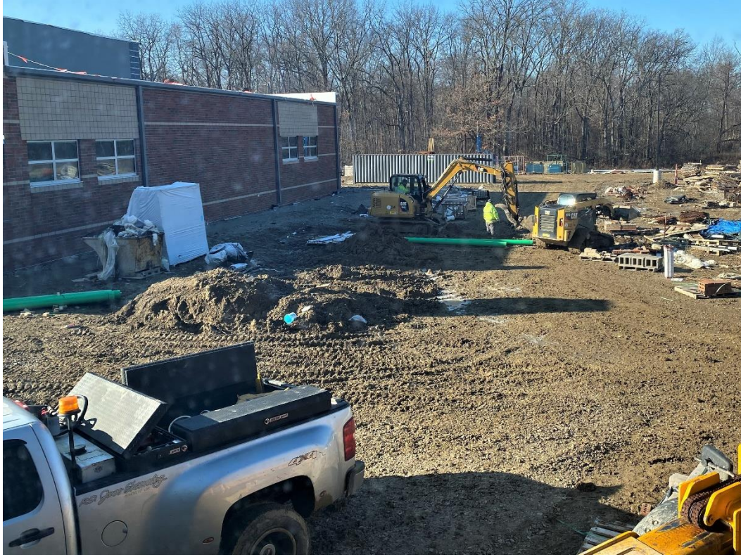
R D Jones is installing below grade storm piping linking the downspouts to catch basins and manholes.
