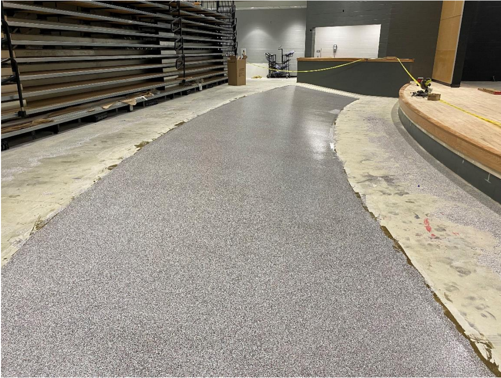
Epoxy flooring beneath the fixed Performing Arts slope seating is complete.
