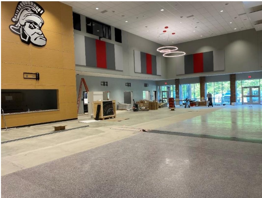
Epoxy flooring installation continues in Area F.
