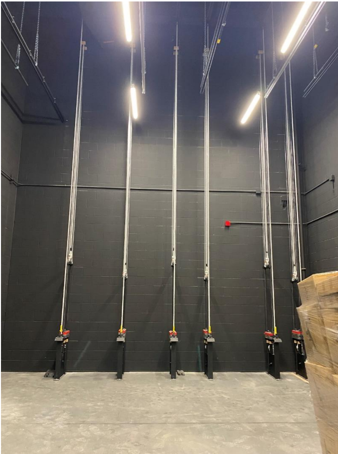
Stage rigging is complete.
