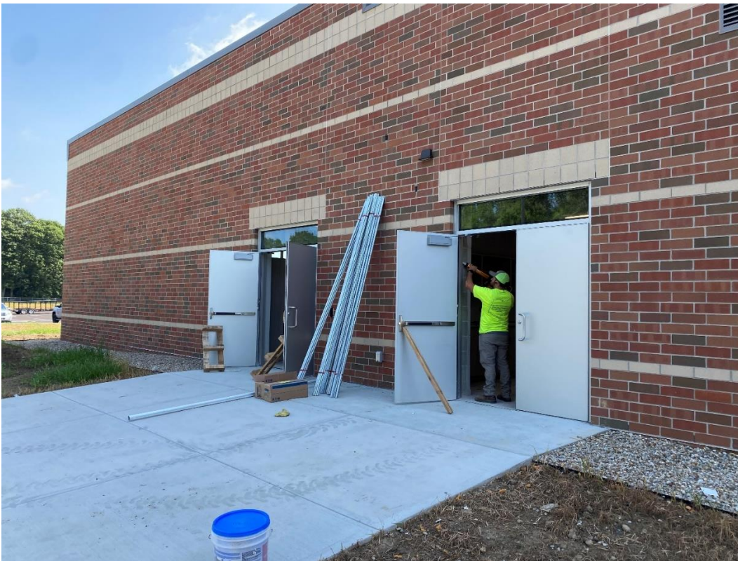
Aluminum doors and transom panels are installed at the Music Classrooms and Stage/Set Storage.
