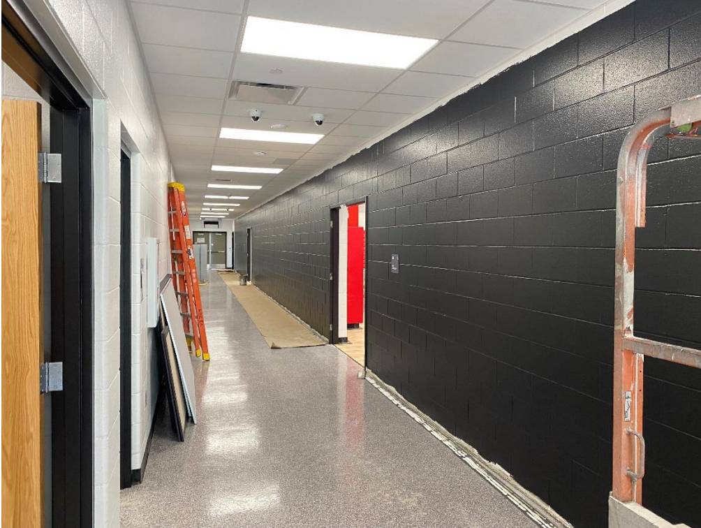
The accent wall in the Locker Rooms Corridor is ready for the Spartan graphics.
