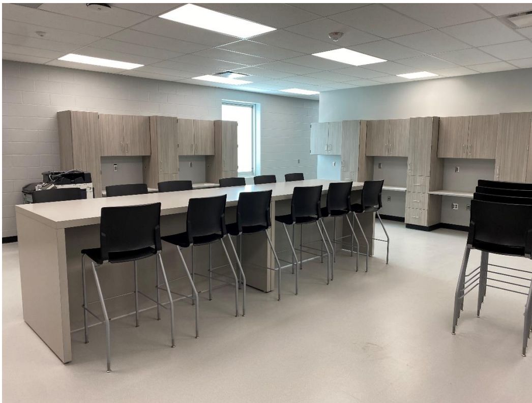
Final data connections and furnishings are being placed in all areas; Teacher's Prep Room is shown here.
