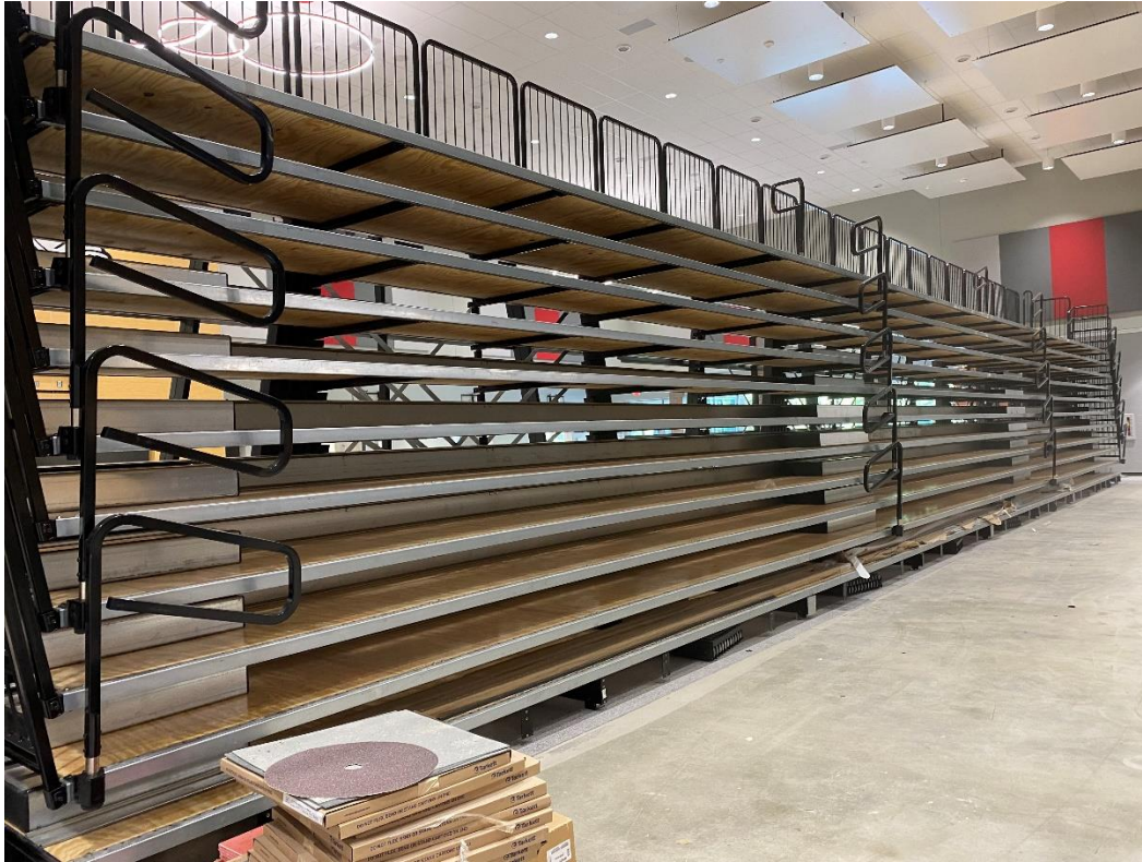
Seating for the Performing Arts Center is nearly complete.
