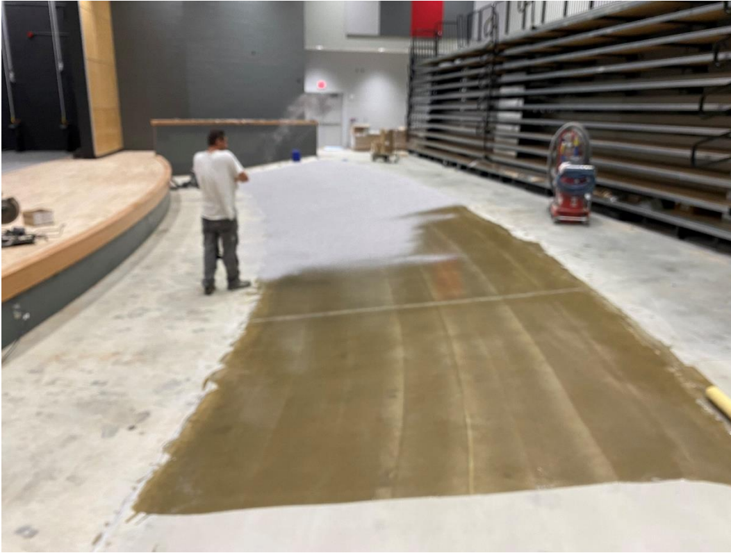
Color flakes are being scattered for the floor below the fixed Performing Arts seating.
