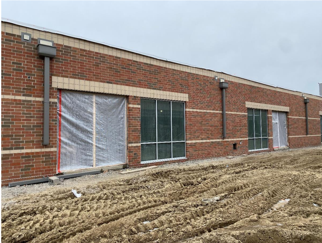
Thru-wall scuppers and downspouts are installed at the north courtyard.
