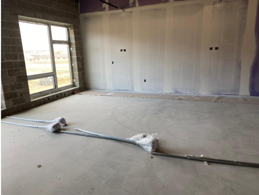
Classrooms are staged with ceiling grid suspension wire at the second floor of Area D. Installation of grid will start in January.
