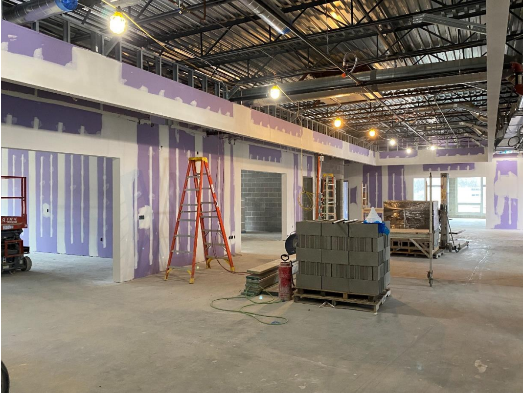
The final finish and sanding of drywall at the second floor of Area C is nearly complete.
