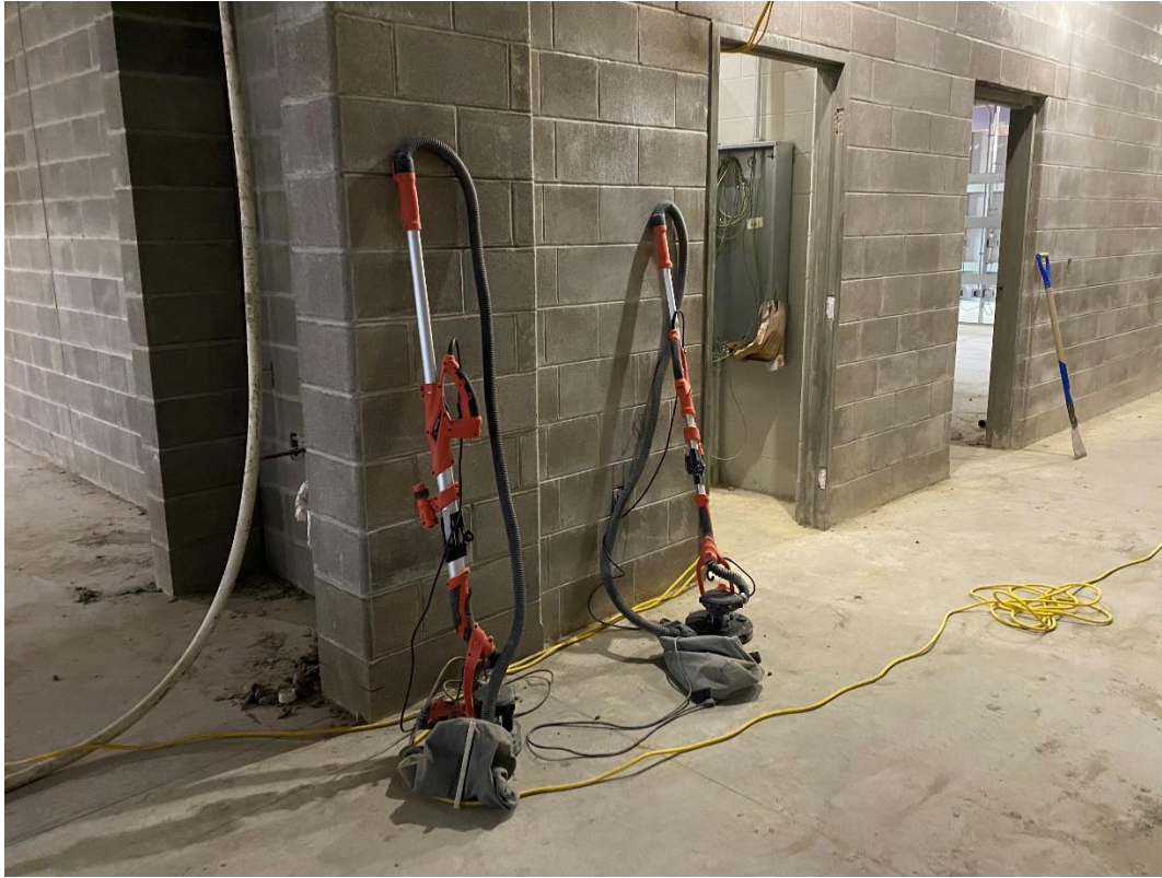
Masonry walls in Areas C & D are being pointed, ground, and cleaned in preparation for painting.
