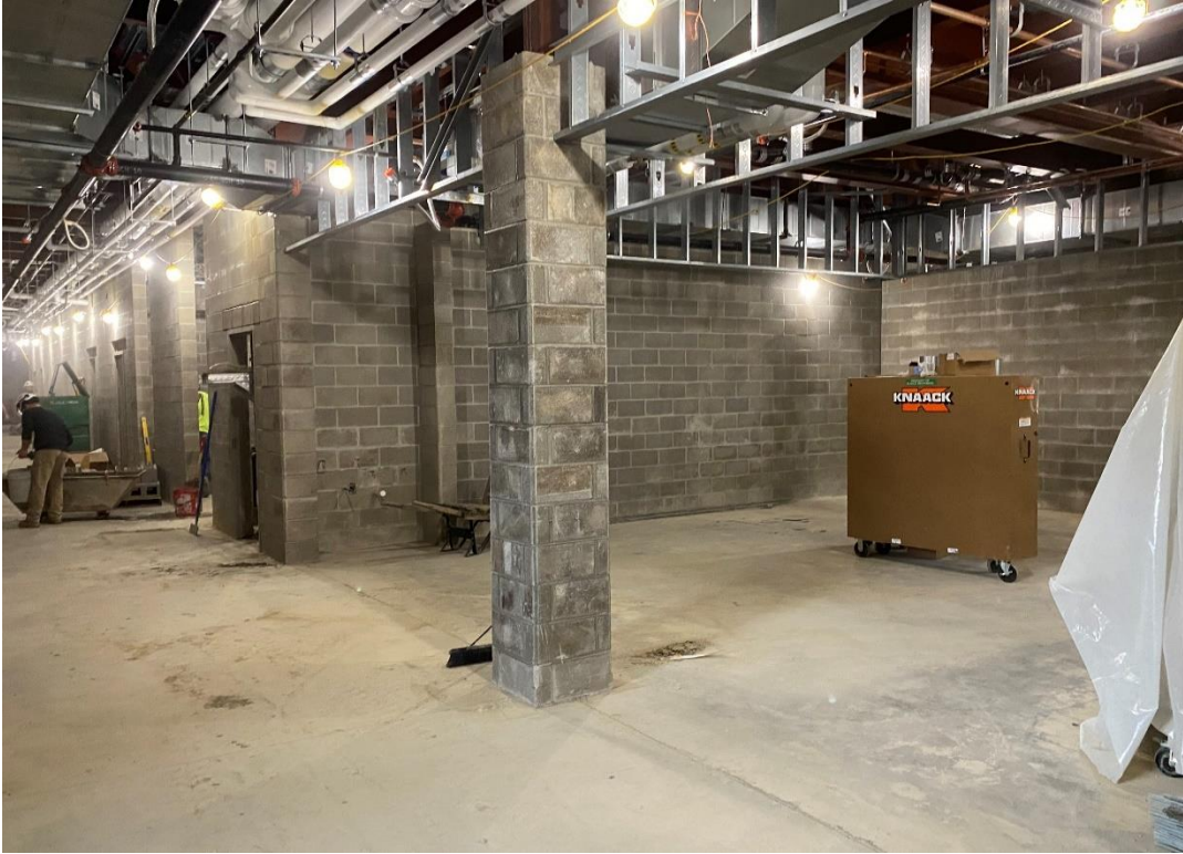
Masonry column enclosure and lightgauge metal soffit framing is installed at the first-floor of Area C.
