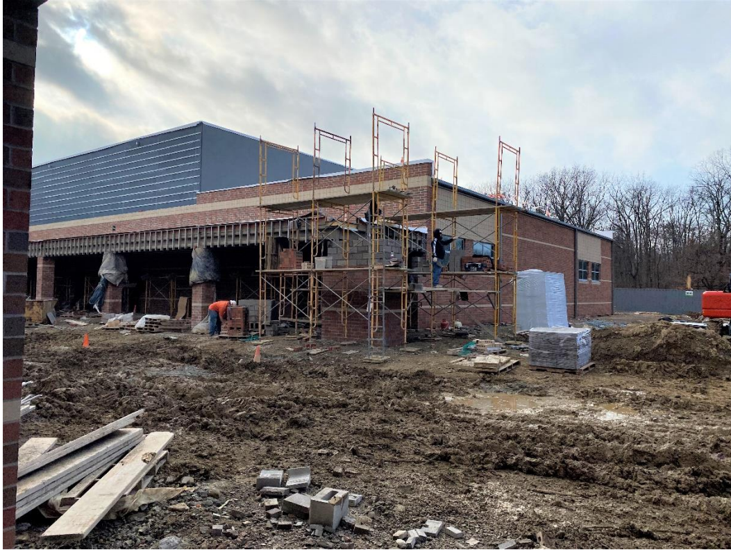
Brick masonry is nearly complete at the north entry canopy.
