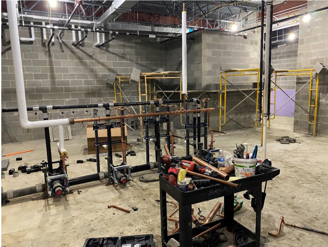
Plumbing rough-in work continues in the main toilets at the first-floor of Area C.
