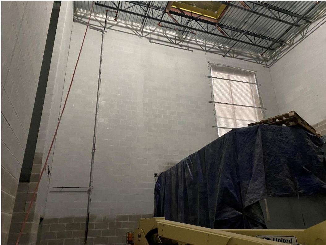
Prime painting of masonry wall in the Area C mechanical room.
