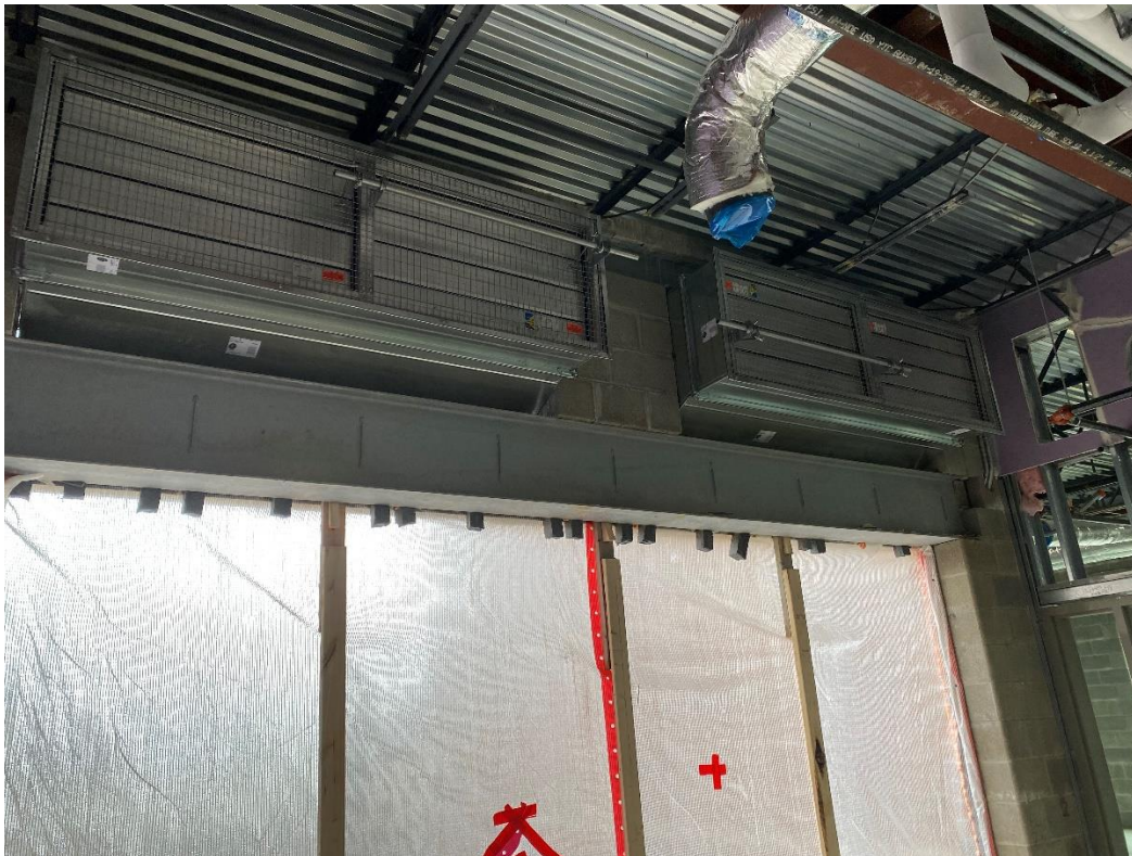
Louvers and motorized dampers are installed in Area D.
