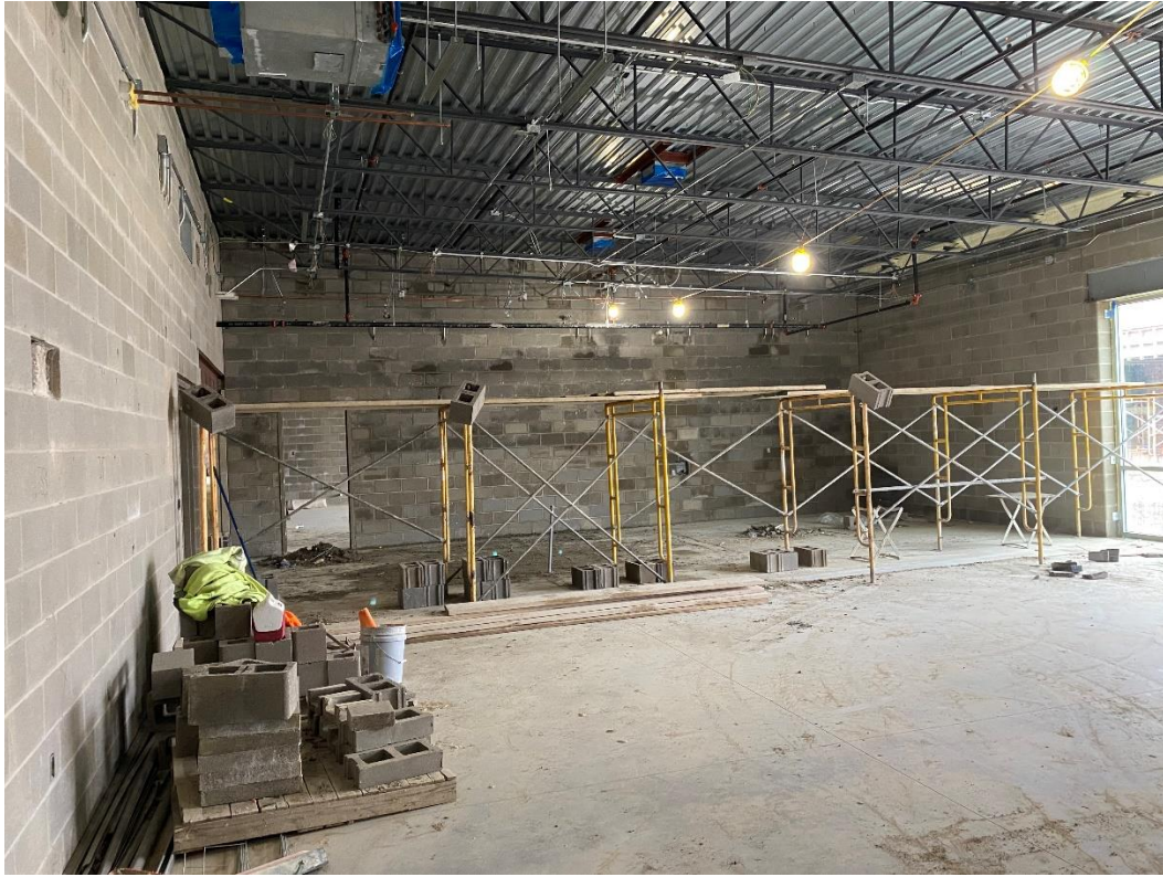
Masonry partition walls are being completed in the Art Rooms.
