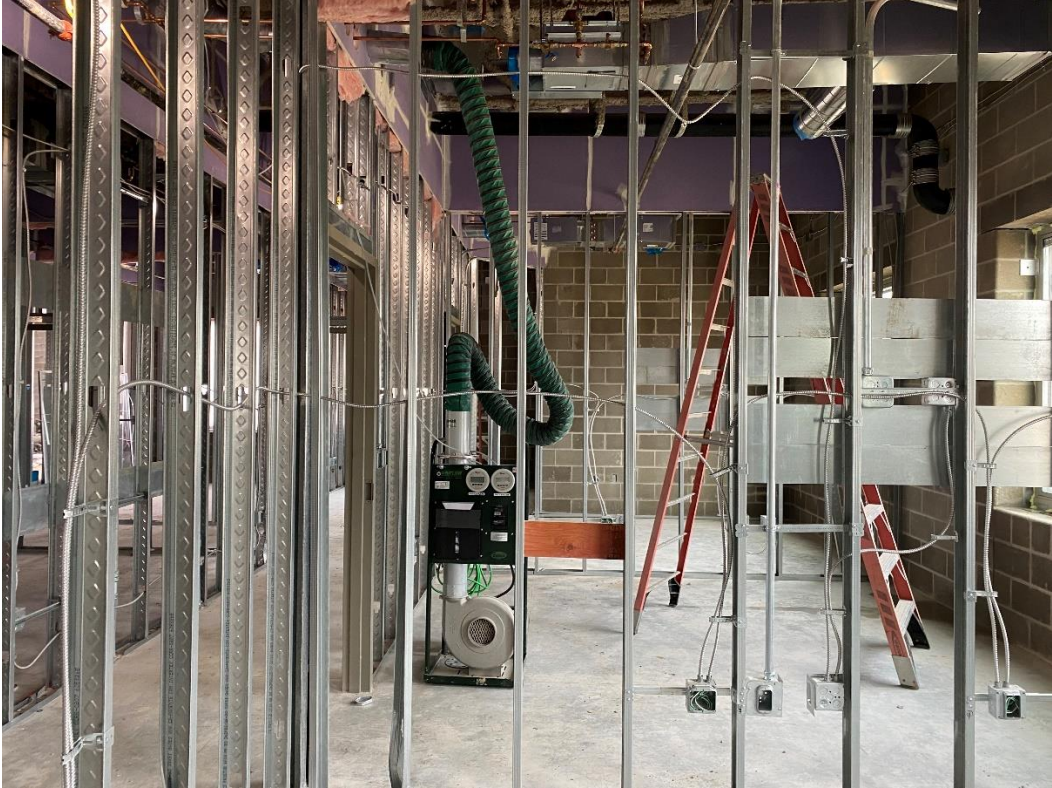
Pressure testing of ductwork in Area A, Administrative Offices.
