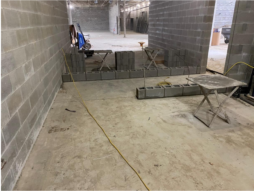
Interior walls of the main restrooms east of the Gym are started.
