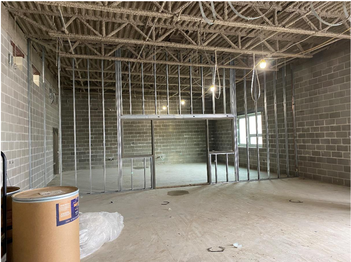
Interior partition at 108 Idea Lab is installed.
