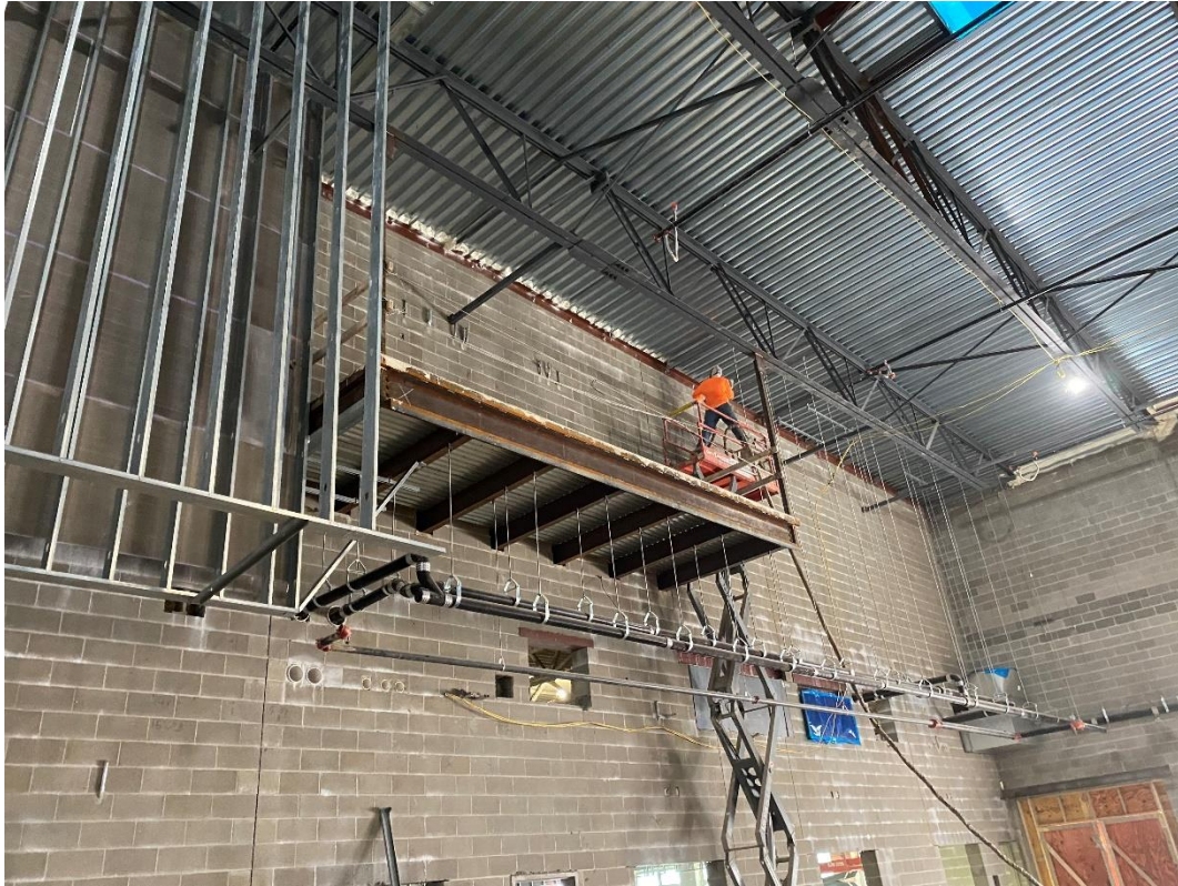
Foam insulation is being installed at the juncture of the roof and wall at the performing arts center.
