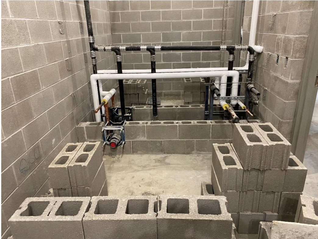
Interior masonry partition walls are progressing in toilet rooms as plumbing is roughed-in.
