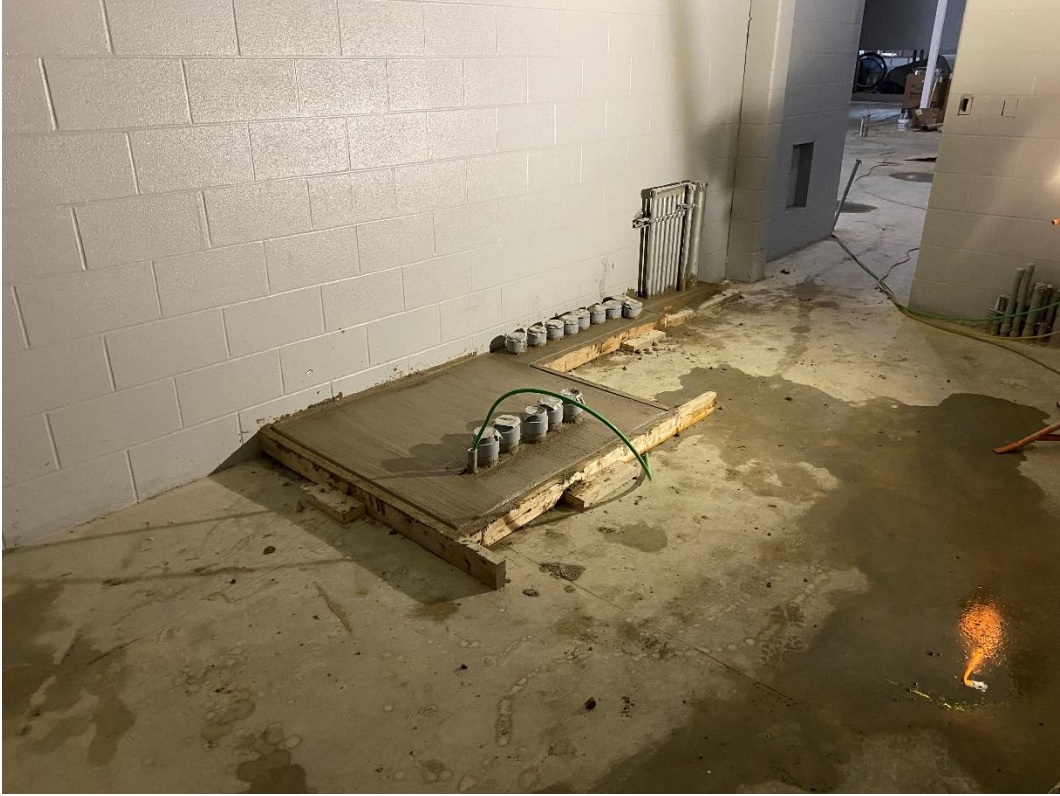
Electrical equipment pad is installed in the main electrical room.
