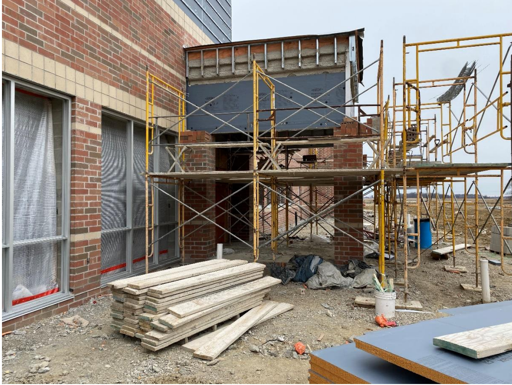
Columns are bricked; just the walls above the vestibule windows to finish with brick.
