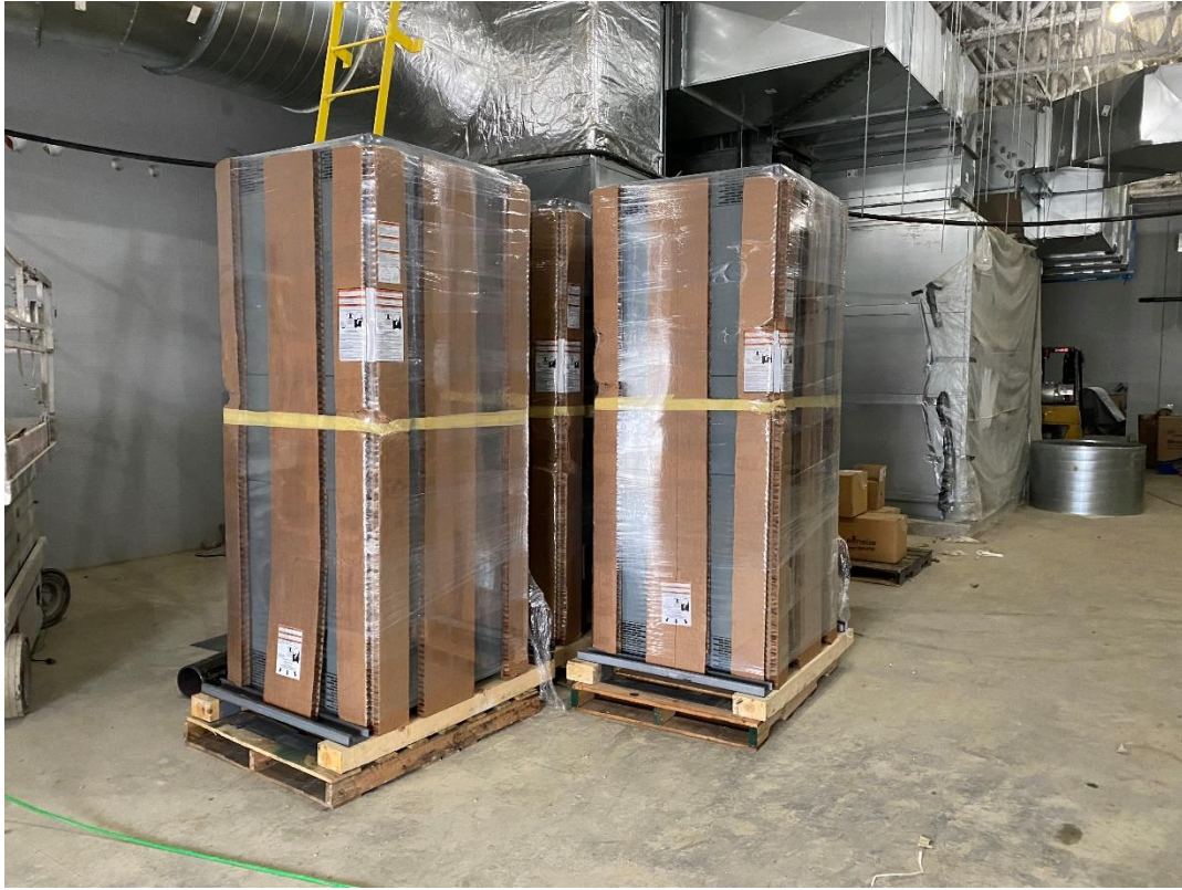
Sections of electrical switchgear are arriving and staged in the mechanical room.
