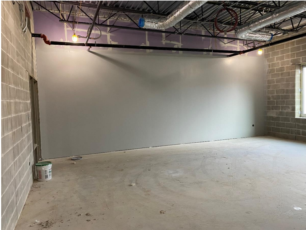
Prime painting of drywall partitions continues in Area C.
