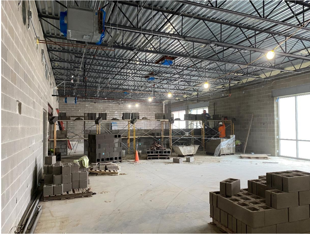
Construction of interior masonry walls is progressing in the Art Classrooms.
