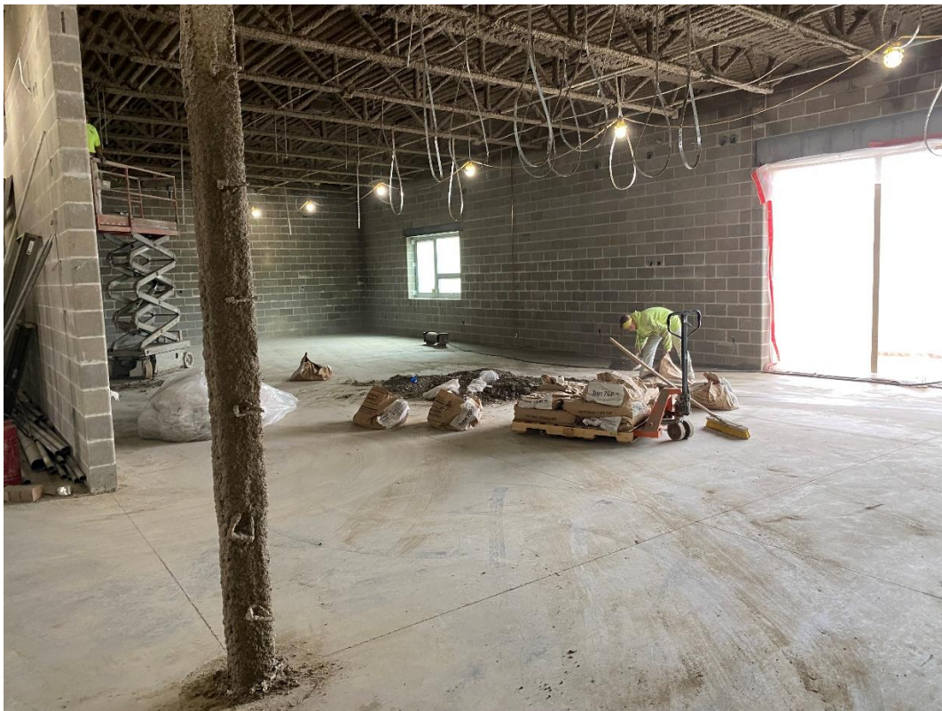
Fireproofing is complete. Room is cleaned for interior partition wall construction to continue.
