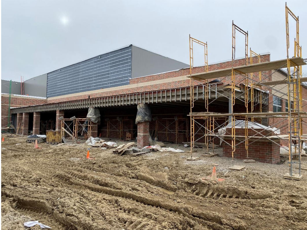
Exterior brick work is idle until weather warms. View looking SW toward performing arts center.
