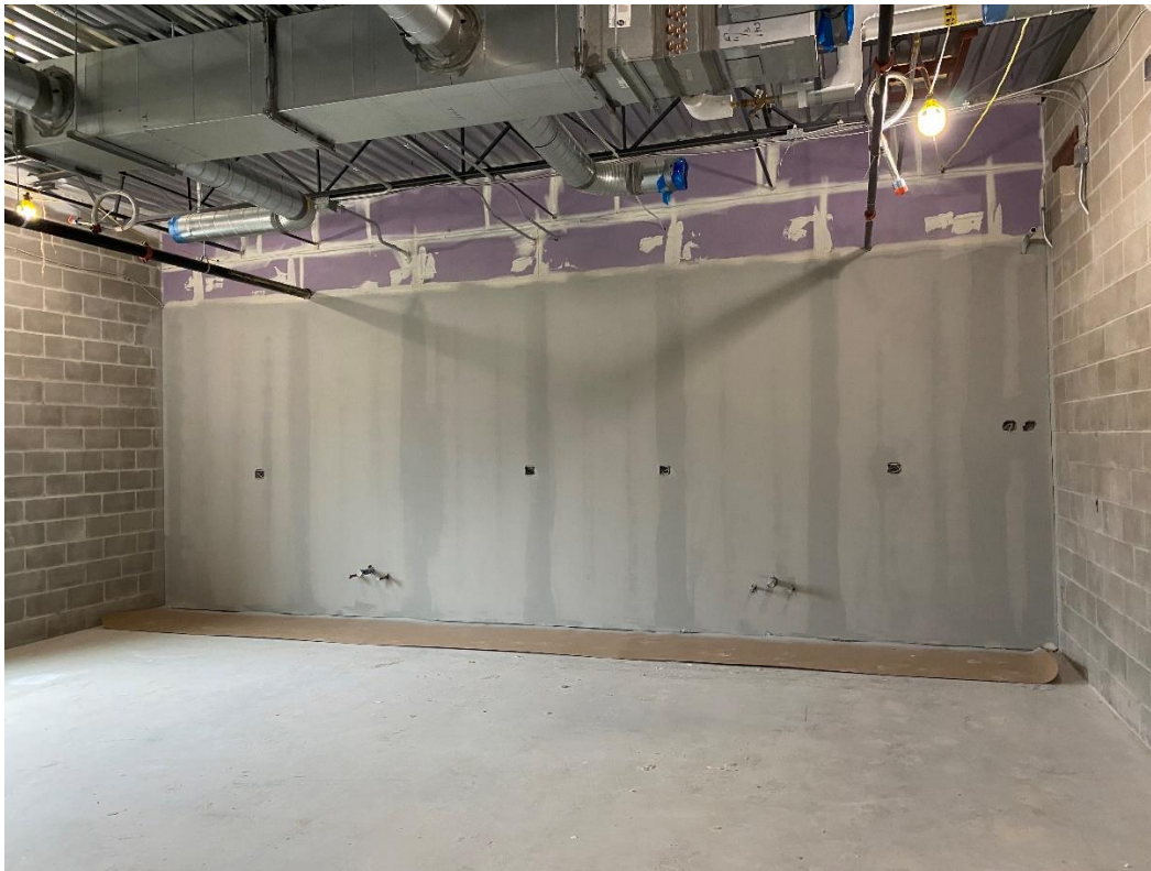
Prime painting of drywall has started in Area C.
