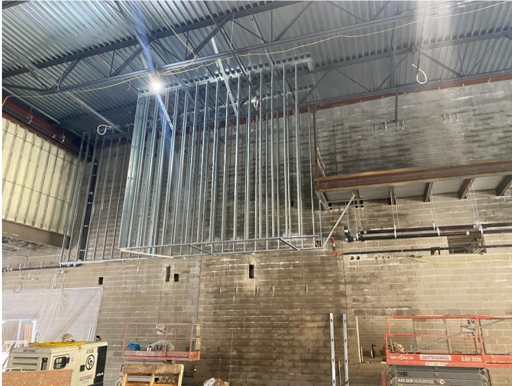
Framing of the soffit above the concessions and stair access to the control booth has started. View looking south at the north wall of the Gym.
