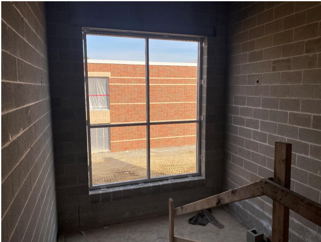
Large windows are installed in the north stair at Classroom Area C.
