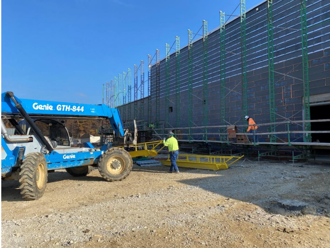
Ships ladders for access to the control booth for the Performing Arts Center.
