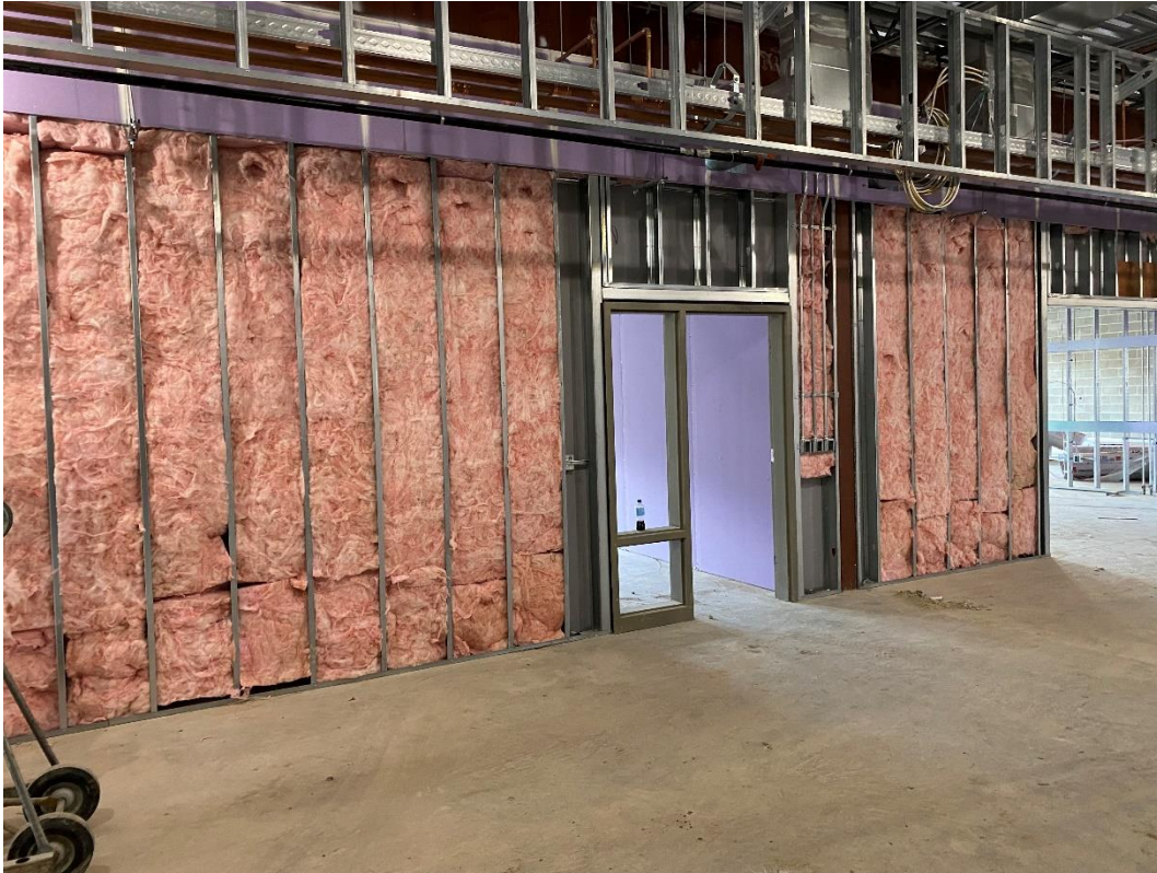
Installation of acoustical insulation in stud walls of Area D Classrooms.
