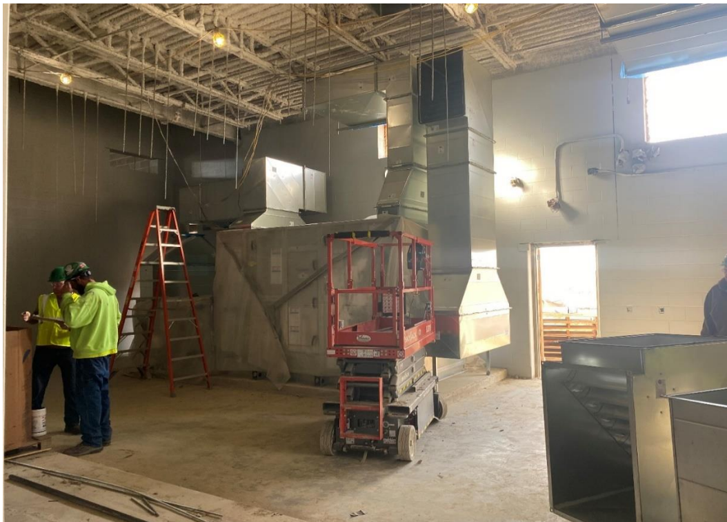
Installation of main ductwork for the air handlers is progressing in the min mechanical room.
