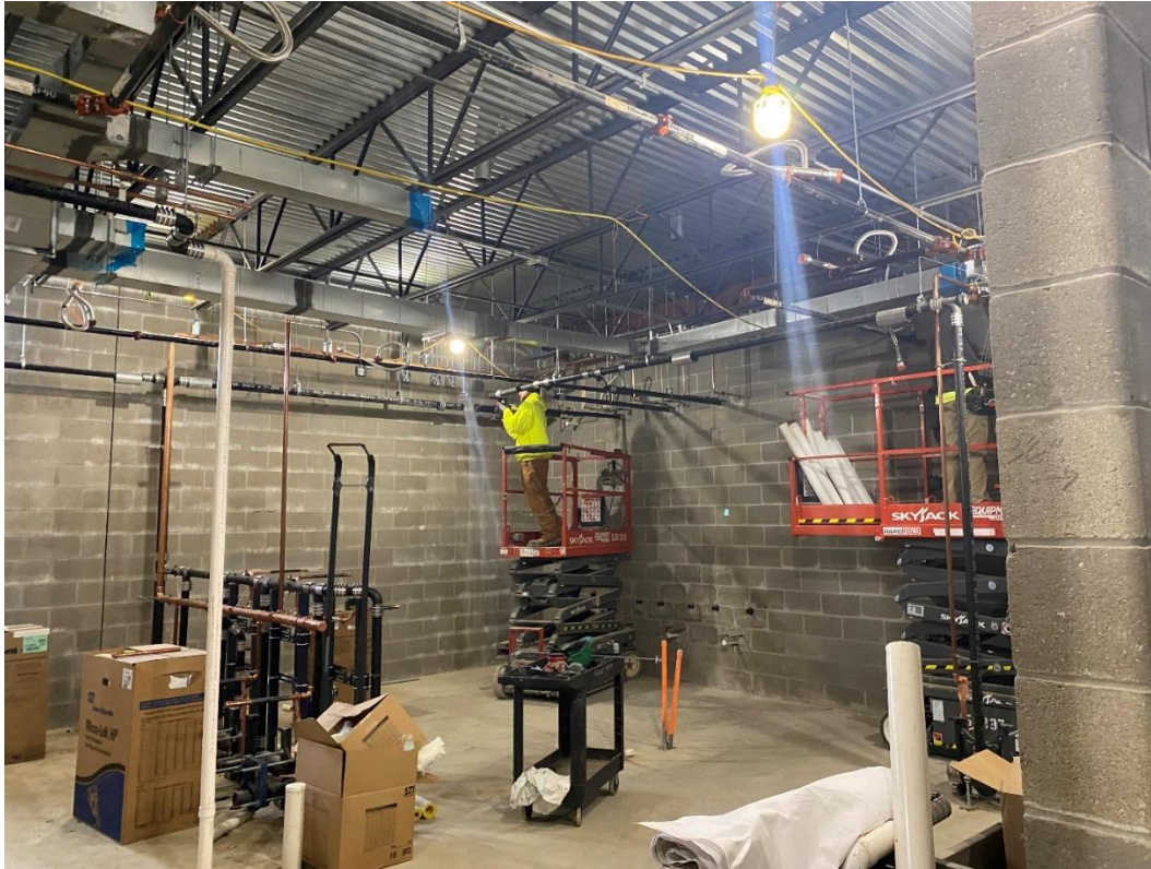
Plumbing rough-in continues in the main toilet rooms, first-floor, Area C.
