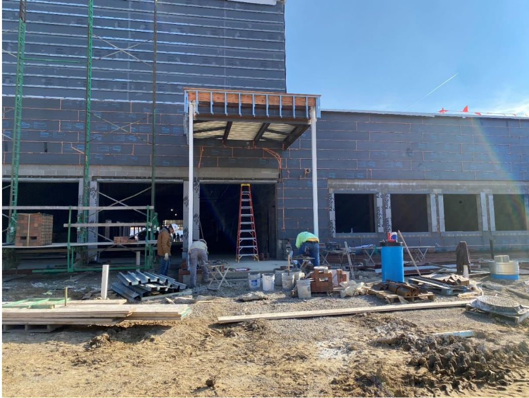
Masons start brick columns at the west entry vestibule.
