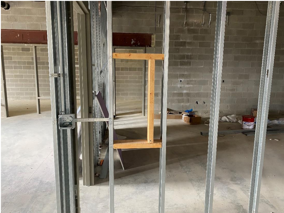
Wood blocking for anchorage of fire extinguisher cabinets.
