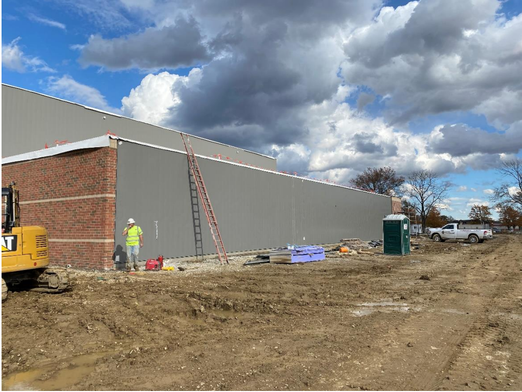
Installation of metal siding is complete on the south wall of the locker rooms.
