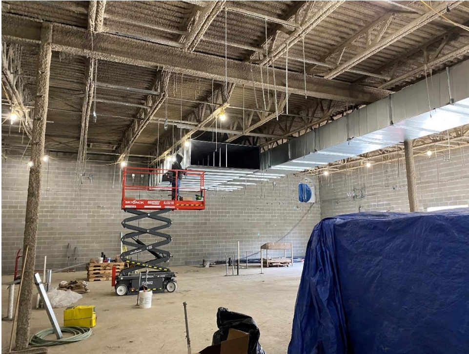
Installation of large main ducts is progressing in the Kitchen.
