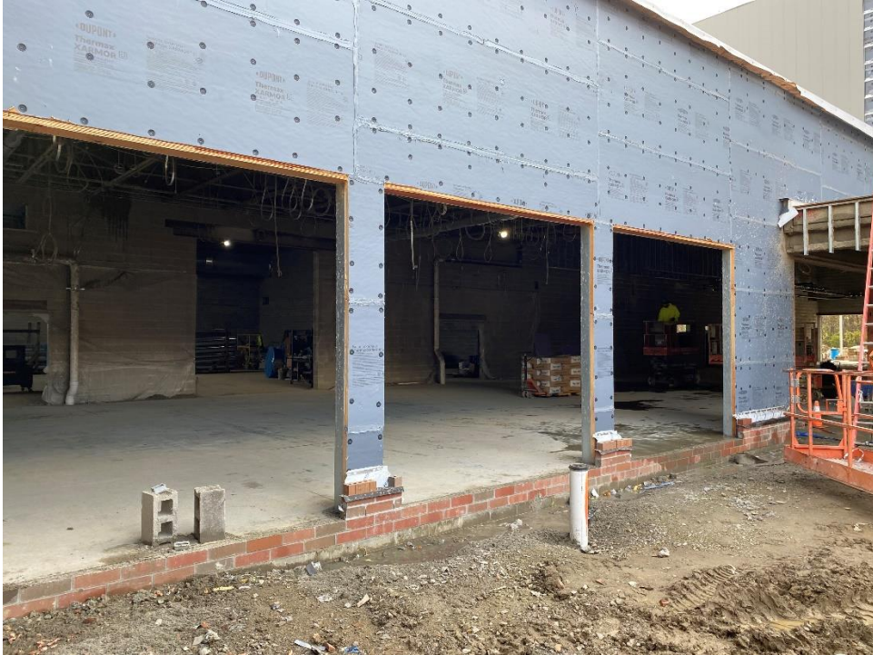
Wood blocking is installed for window anchorage at the north wall of Student Dining.
