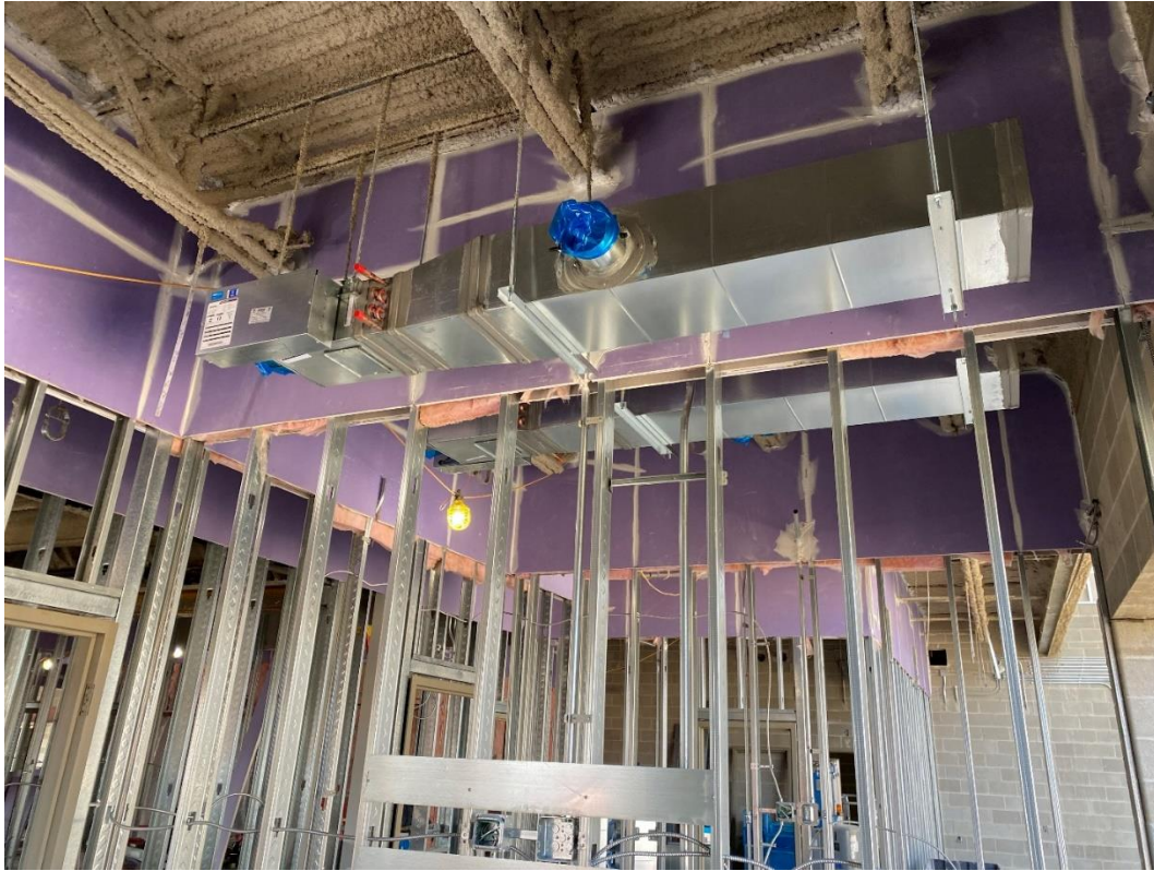
Installation of VAV boxes and above ceiling drywall in Area A.
