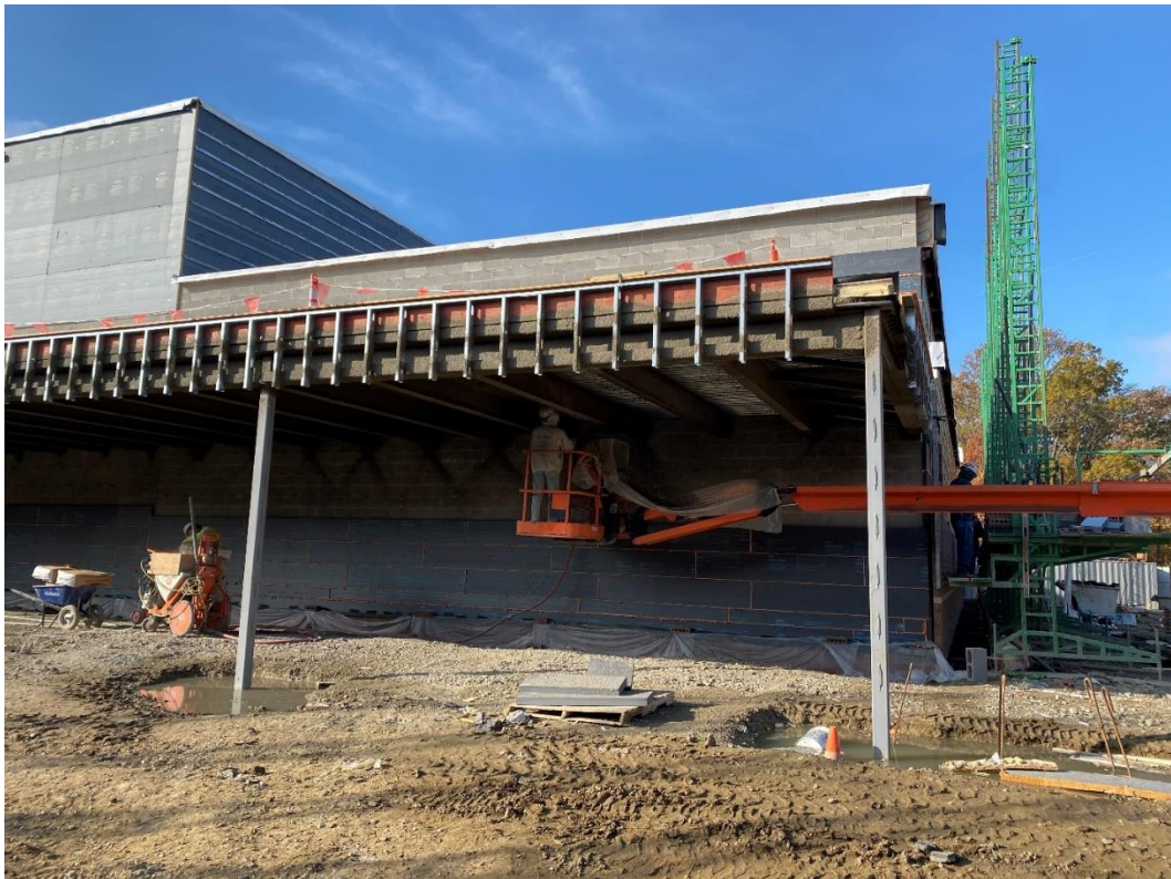
Installation of the air barrier on the east wall of the music classrooms below the north entry canopy.
