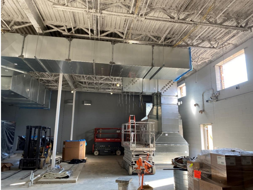
Installation of large ducts from the air handlers in the main mechanical room is progressing well.
