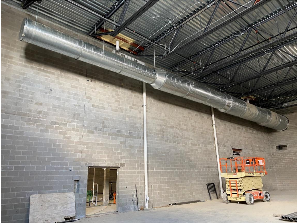
Installation of large spiral duct is progressing in the Gym.
