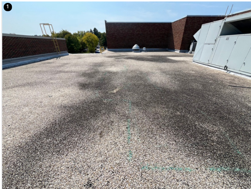
Section C - overall roof photo.
