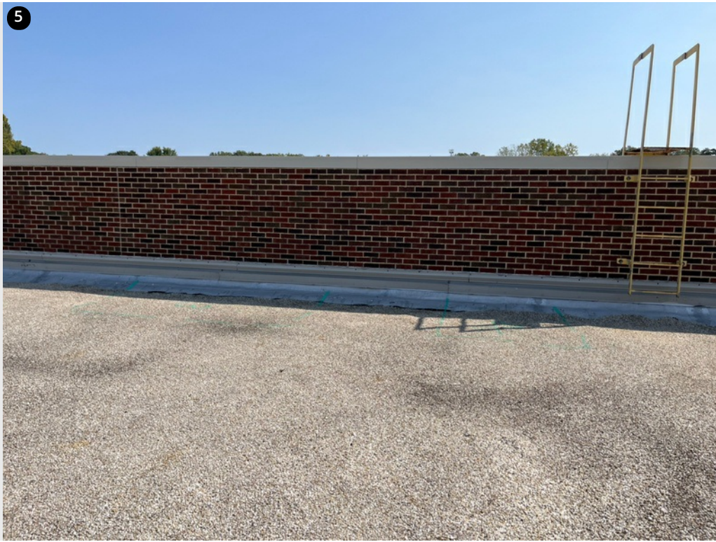
Section C - overall view of the wall. Wall panels are recommended.
