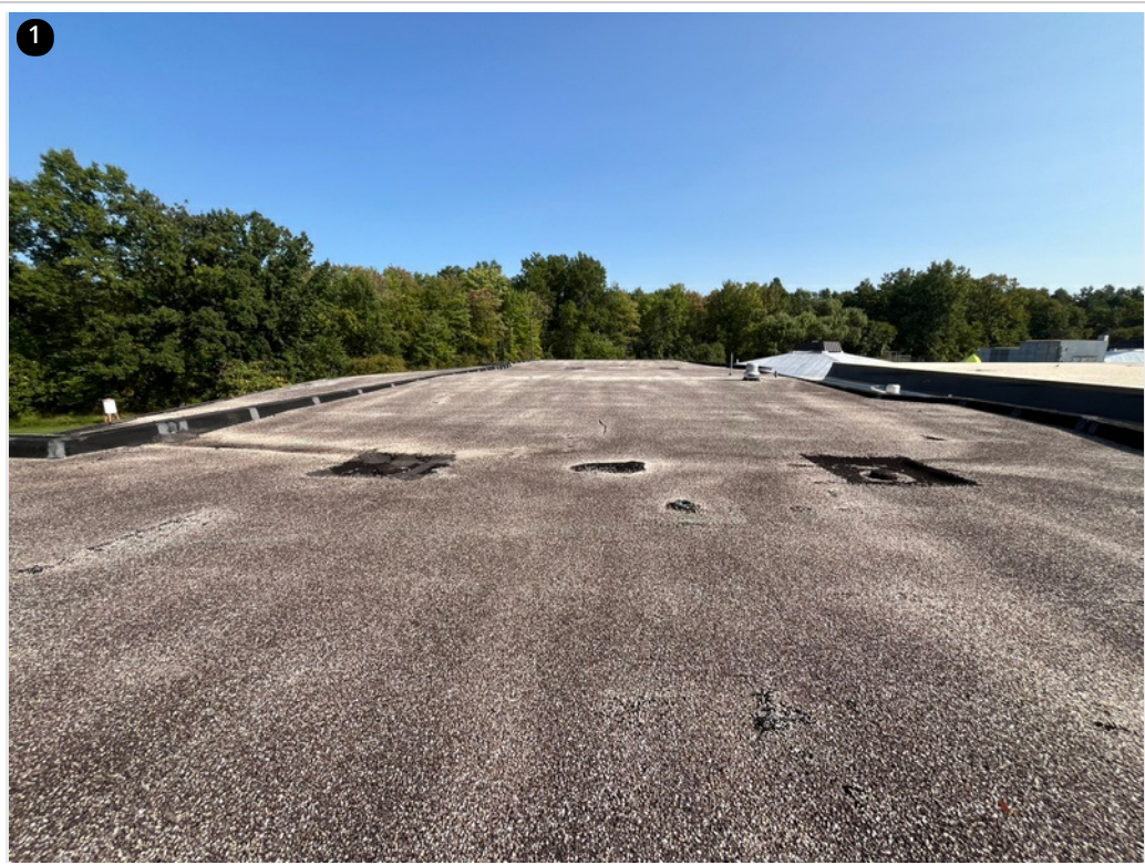
Section F - overall roof photo.
