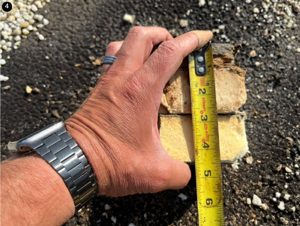
View of the roof assembly.
