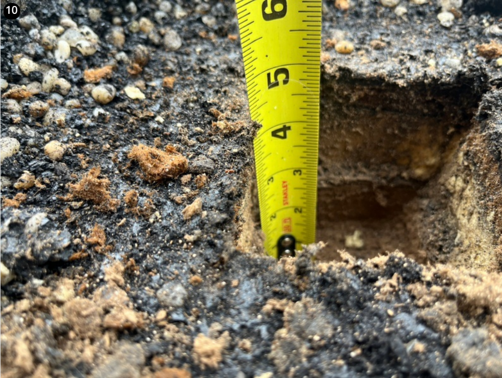
10 The overall roof thickness is approximately 4 inches.
