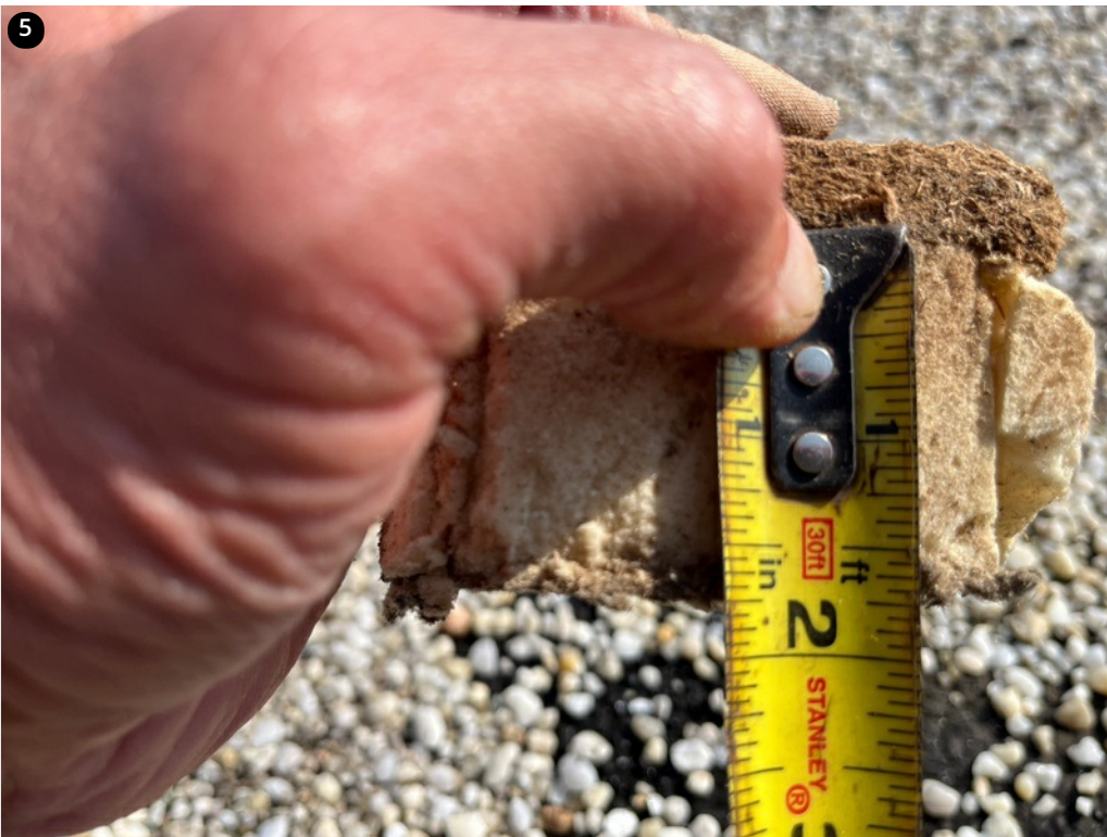
The ISO insulation is 2 layers of 1.75".
