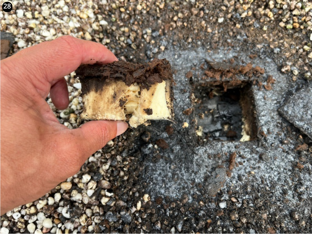
Section D - view of the saturated roof assembly.
