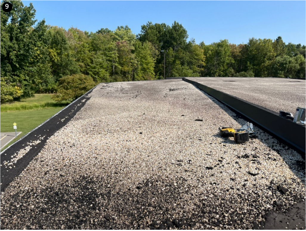
Section G - overall roof photo.
