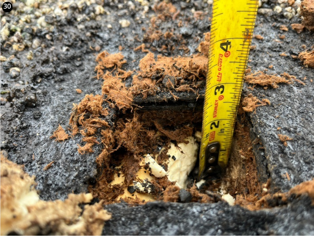
Section D - the roof assembly is approximately 2.5 inches thick.
