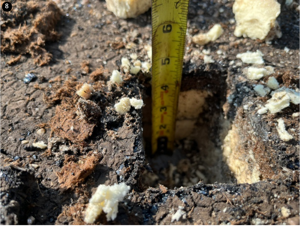
View of the core assembly at the ridge.
