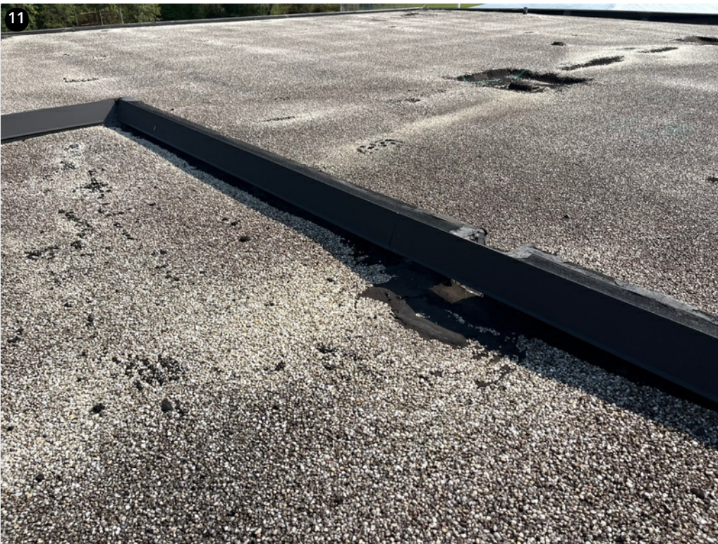
View of the scupper.
