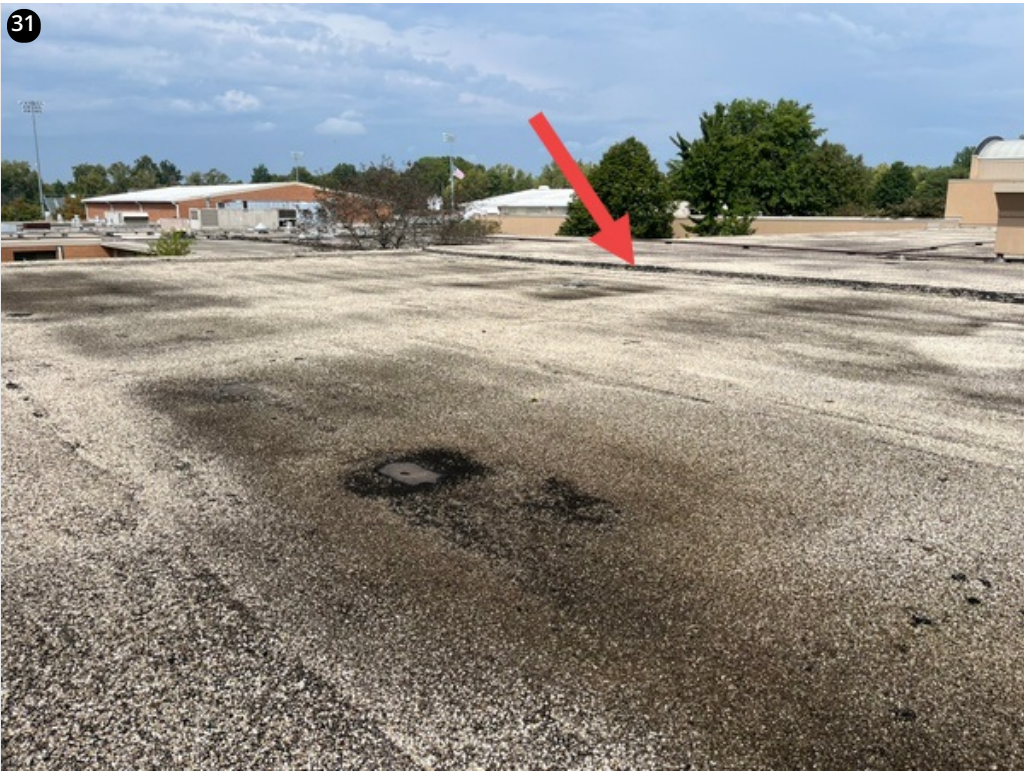
Section E - a transition is present between sections E & D.
