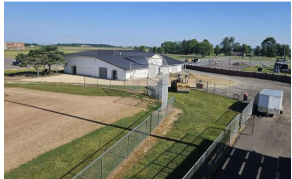
Renovated weight room and locker room
