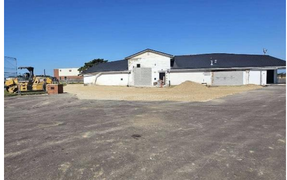
Replacing concrete around new weight room
