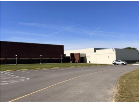
Additional parking and resurfaced blacktop
