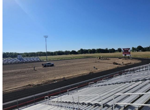
Removing field to replace sod and irrigation
