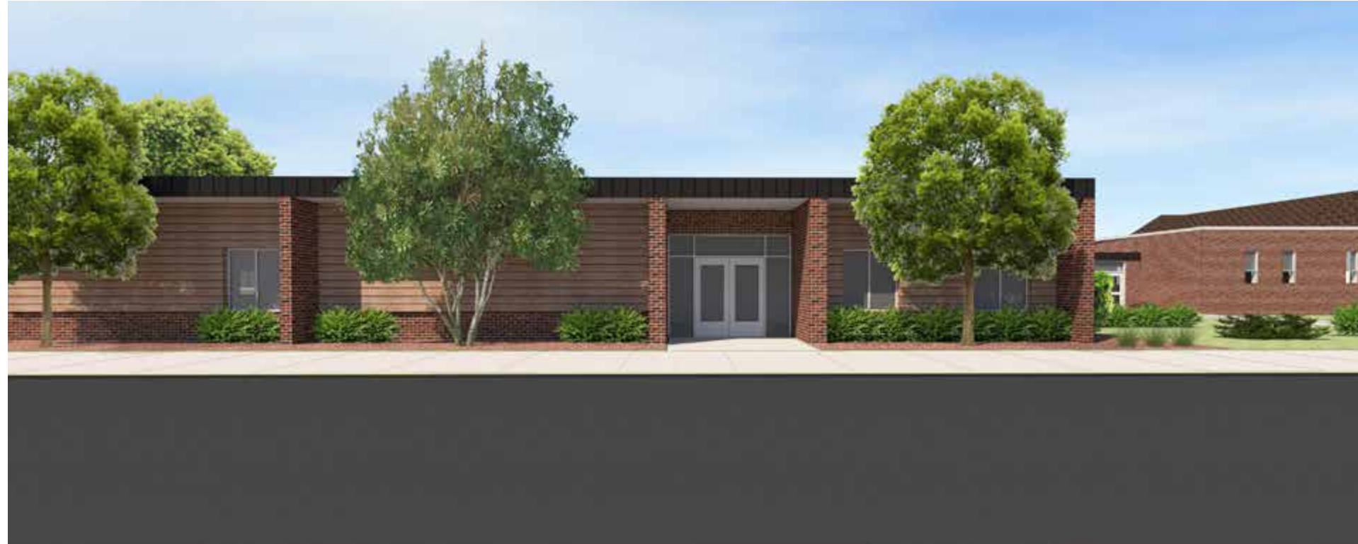
REPLACE WOOD SIDING WITH NEW NICHHA FIBER CEMENT BOARD
