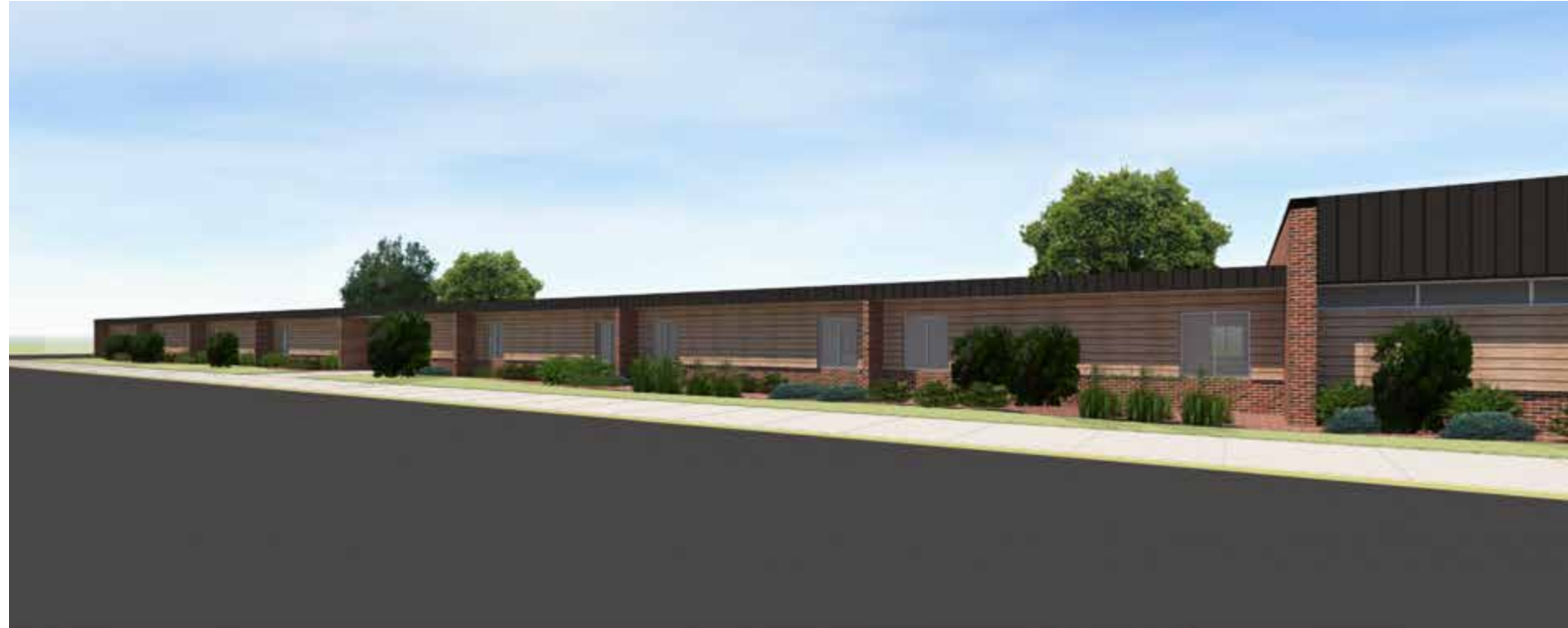
REPLACE WOOD SIDING WITH NEW NICHIBA FIBER CEMENT
