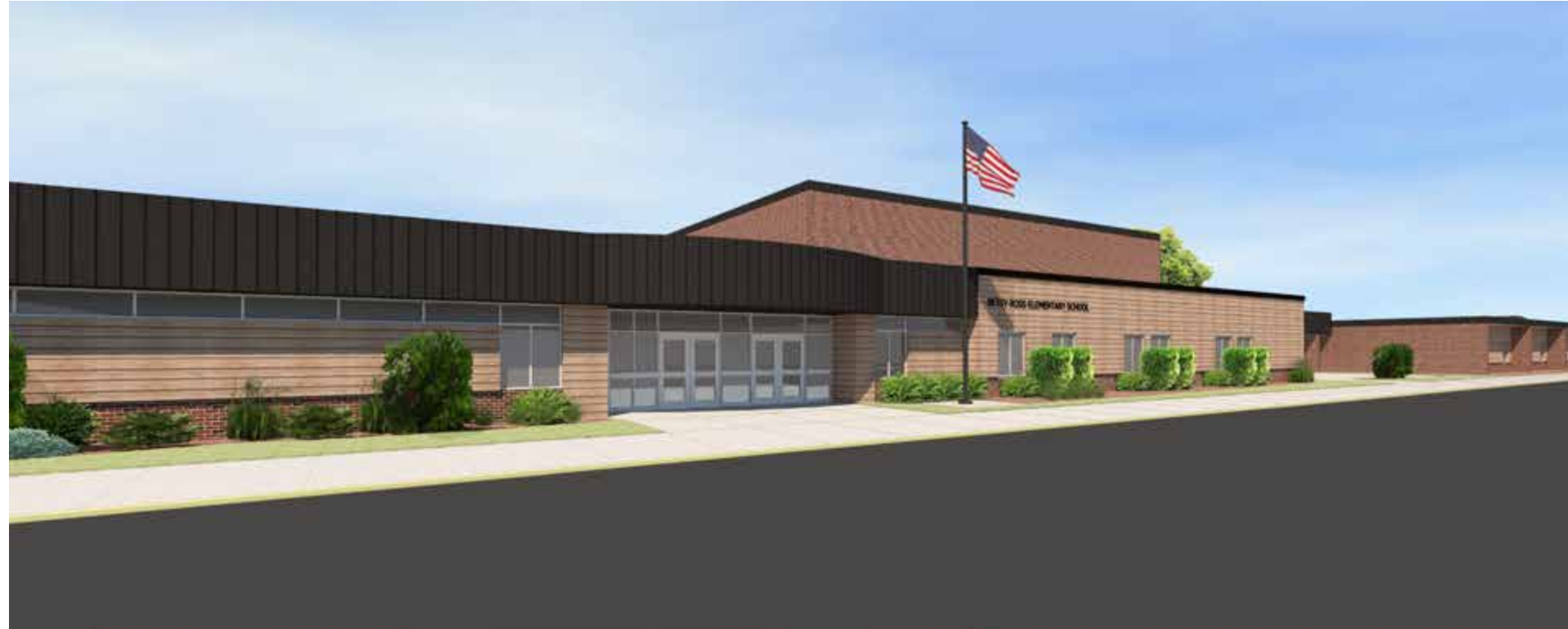
NEW PANELING OVER EXISTING BRICK AT SCHOOL ENTRANCE
