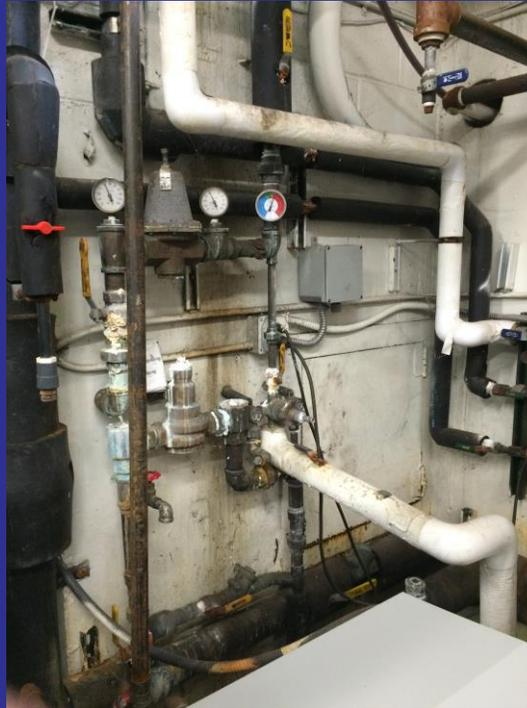
DHW mixing valve in poor condition
