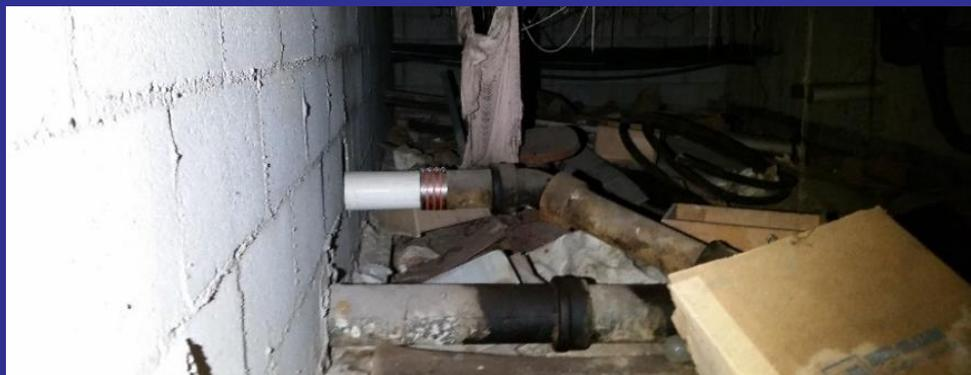
PVC sanitary connections into cast iron
