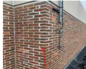
Masonry repairs.
