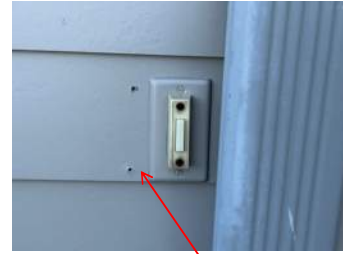
Repair / seal wall
