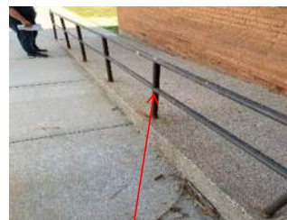
Repaint hand/guard rails.
