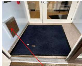
Rusting HVAC Unit
