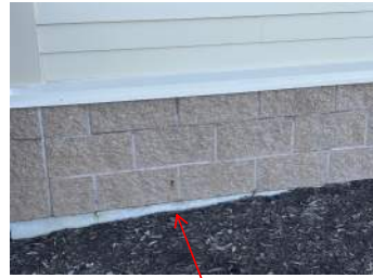
Masonry weeps present
