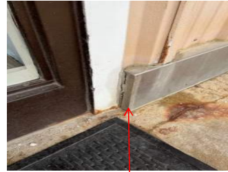
Failing Sealant
