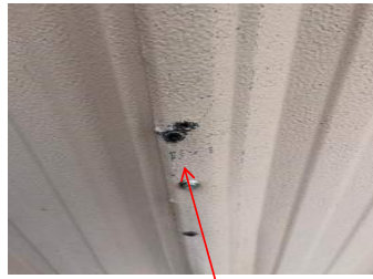
Seal Exterior Wall
