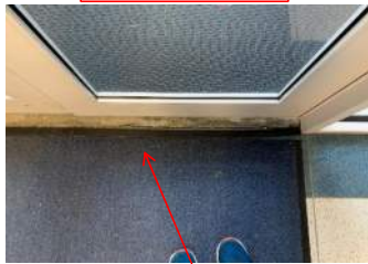
Repair door threshold.
