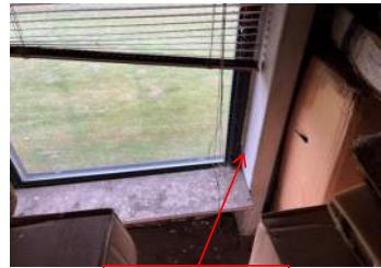
Failing Sealant
