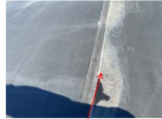
Roofing joint/seam repair.
