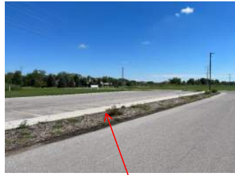
Remove planting area and replace with concrete
