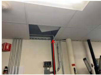
Replace ceiling tiles
