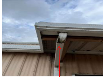
Leaking/Damaged Downspout
