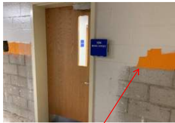
Complete construction work in corridor.
