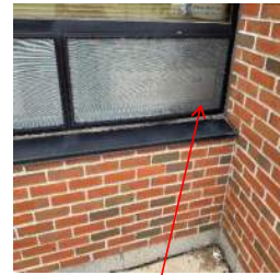
Repair caulk at window sill.
