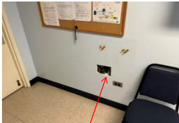
Replace Drinking Fountain
