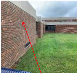
Masonry - repair / tuck point.
