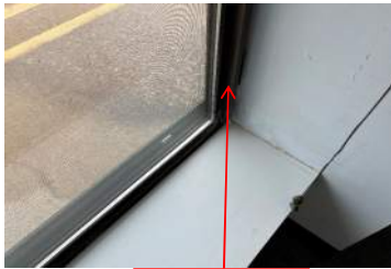
Failing Sealant
