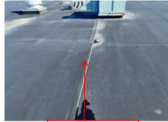
Roofing joint/seam repair.
