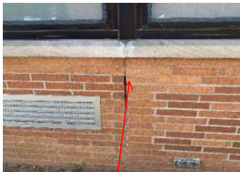
Reseal masonry joint.
