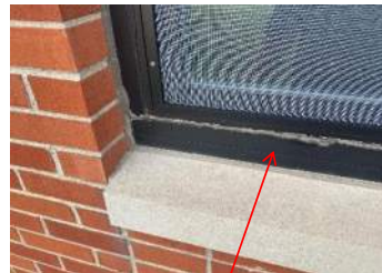
Repair joint sealant at window.
