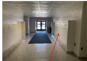
Complete construction work in corridor.
