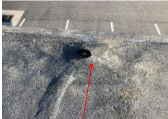
Replace roof drain
