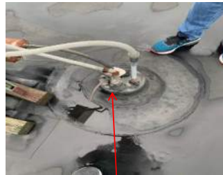
Repair roof penetration.
