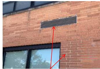
Masonry repairs and reseal louver.
