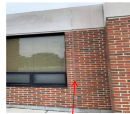
Reseal masonry joint
