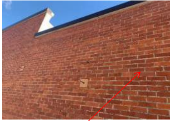
Masonry - repair / tuck point.
