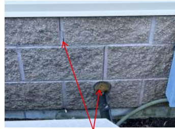
Masonry repairs / seal wall penetration
