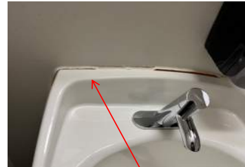
Failing Sealant
