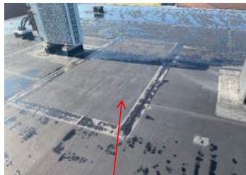
Large roof repair
