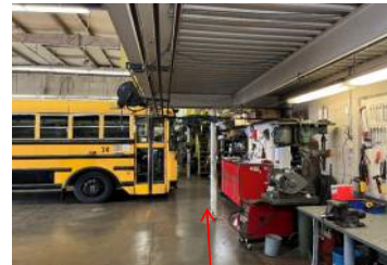
Paint Steel Column
