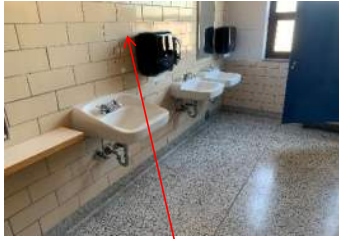
Repair damage to walls / modify sink installation.
