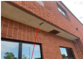
Damaged soffit.
