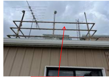
Paint Roof Guard
