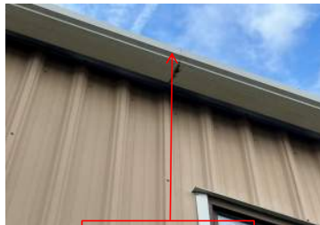
Leaking Gutter
