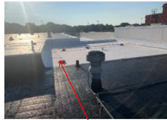
Roofing nearing end of life cycle - white coating applied to extend roof life
