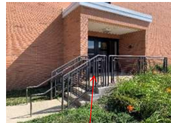
Repaint hand/guard rails.
