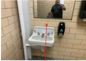
Repair holes in wall.
