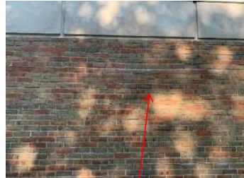
Masonry - repair / tuck point.
