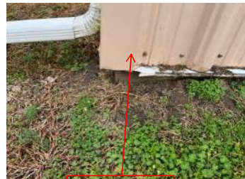
Damaged Sill
