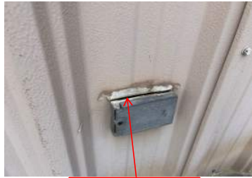
Failing Sealant
