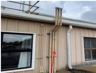
Paint Vent Piping and Conduit
