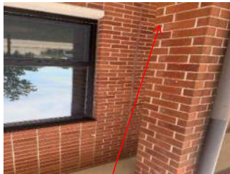
Reseal masonry joint.
