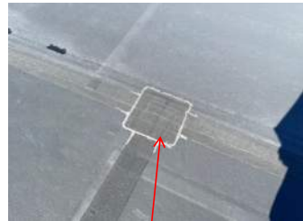
Roofing joint/seam repair.
