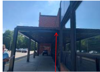
Provide additional roof drainage from canopy.
