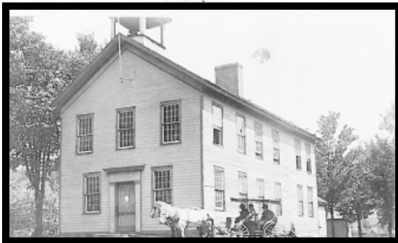
Picture of East Worcester School 1867-1868
